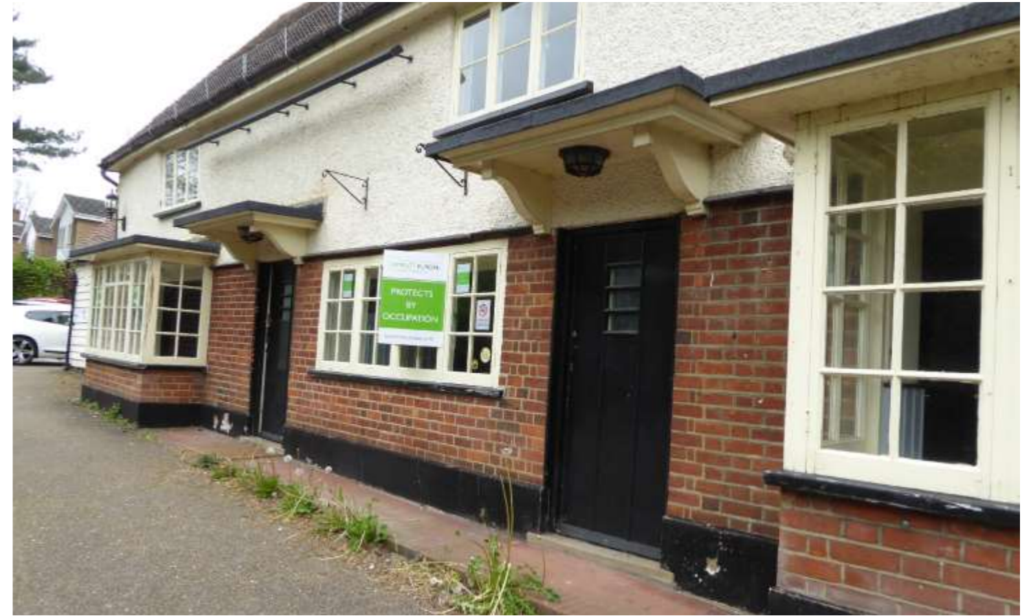
Photo 2: Detail of the façade, from the east.
