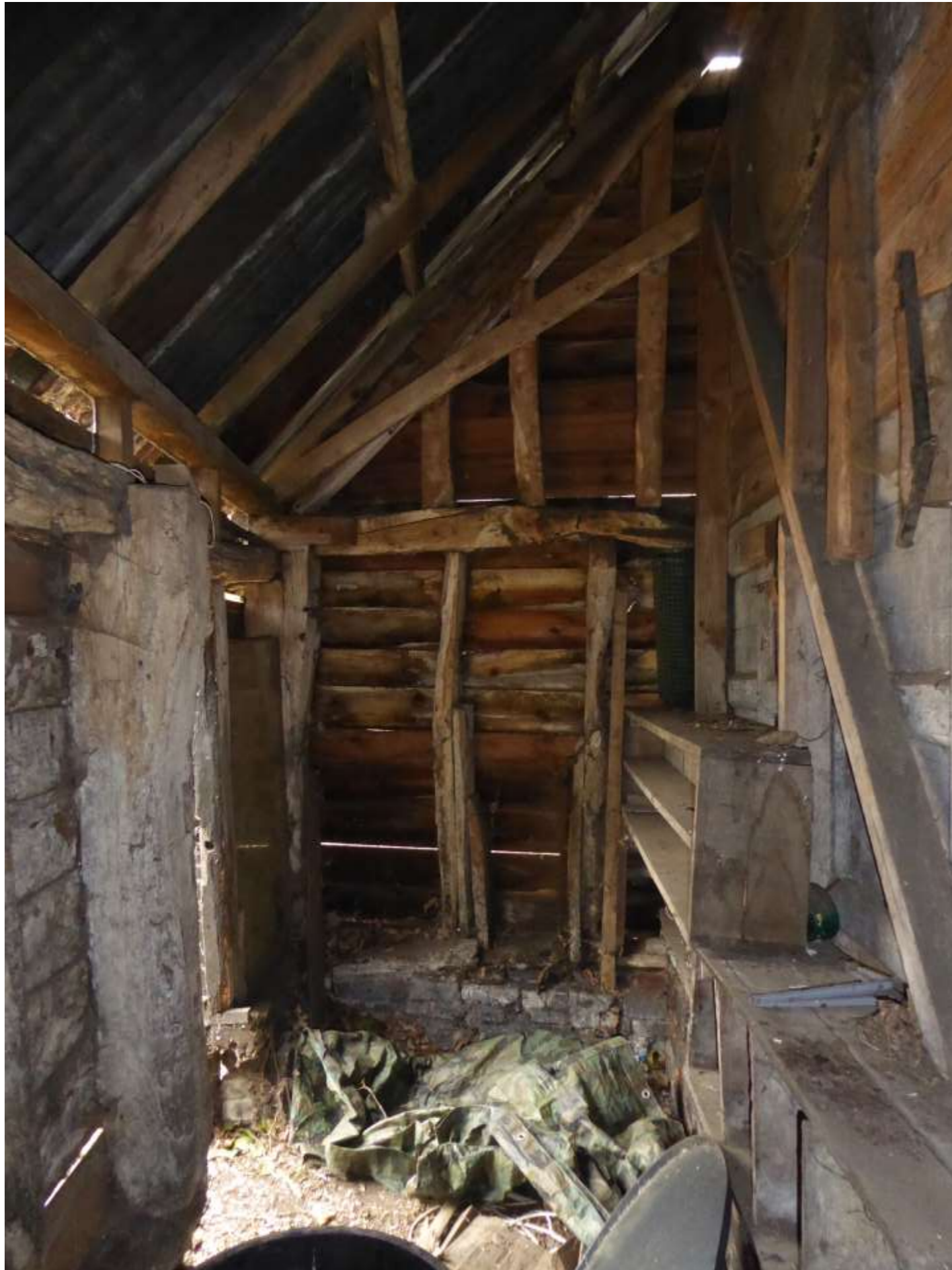
Photo 34: General view south inside the little eastern room with catslide roof.
