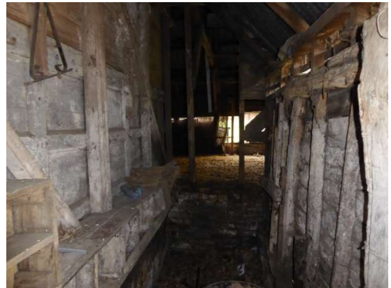
Photo 36: General view north inside the eastern room with catslide roof.
