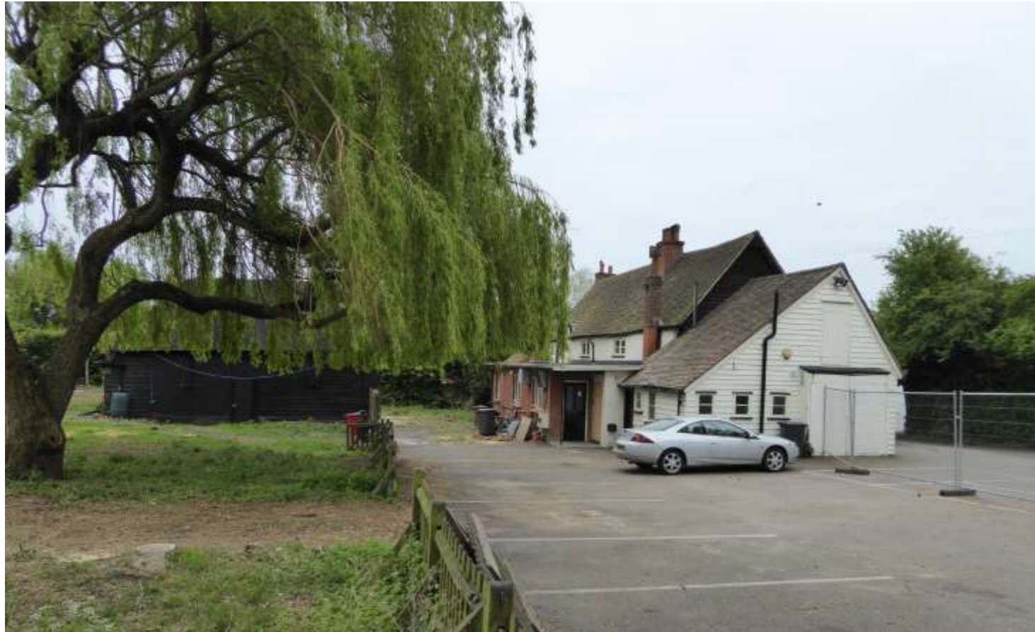
Photo 11: The pub and barn, from the north-west.
