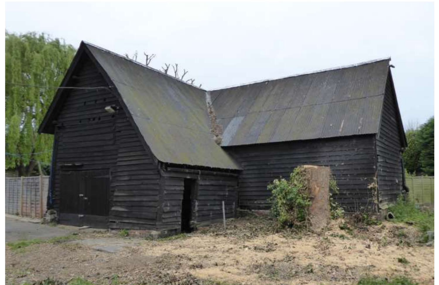
Photo 15 The barn, from the south-east.
