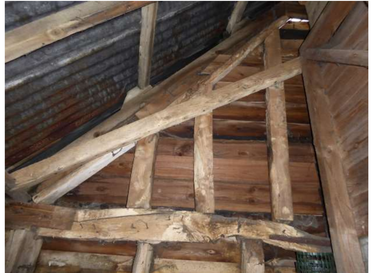
Photo 35: The southern gable of the eastern room with catslide roof.
