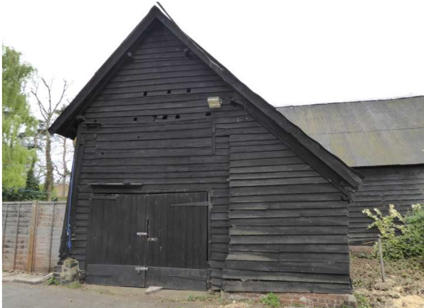
Photo 16: The gabled south elevation of the barn.
