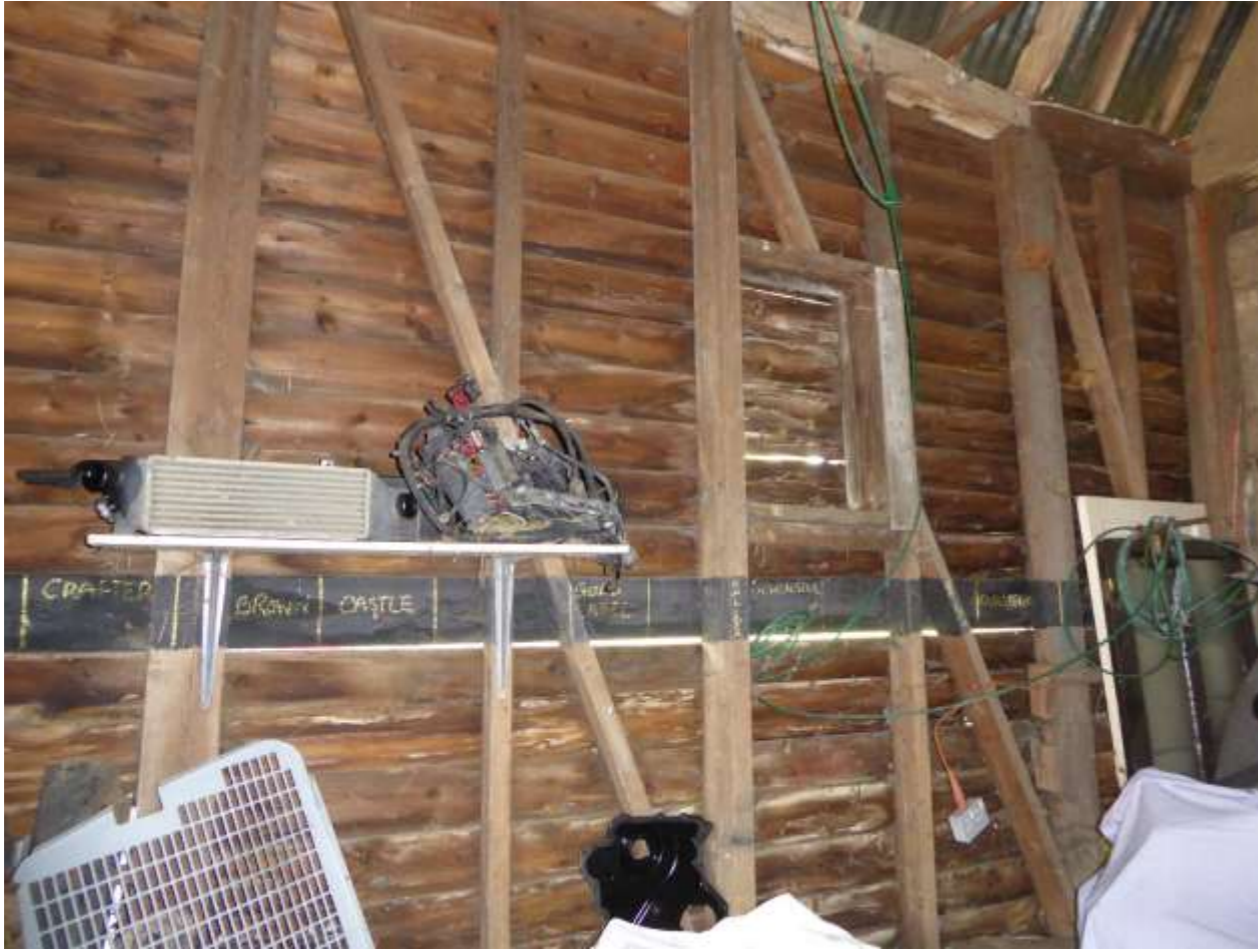
Photo 25: The internal west elevation of the southern part of the barn.
