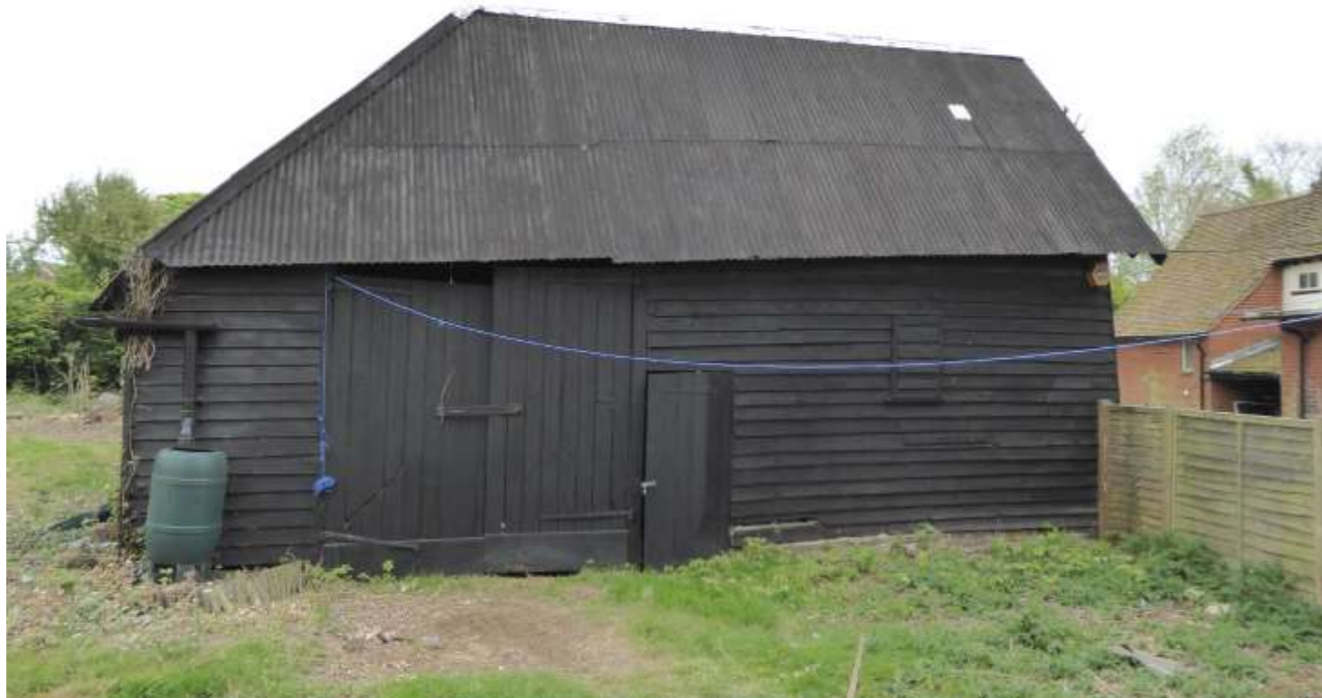
Photo 13: The west elevation of the barn.
