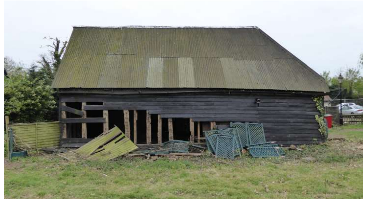
Photo 14: The north elevation of the barn.
