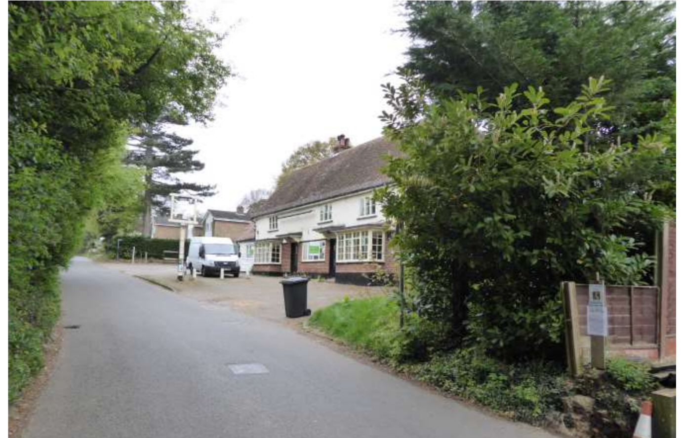
Photo 6: The pub in its context, seen obliquely from the east.
