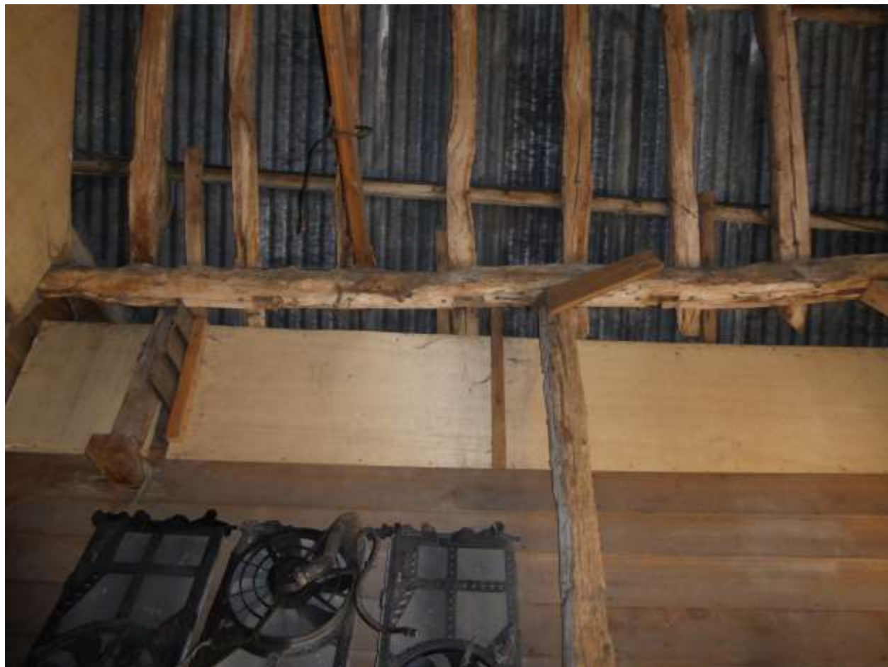
Photo 30: Details of the wall plate along the internal east wall, with stud mortices and stave holes.
