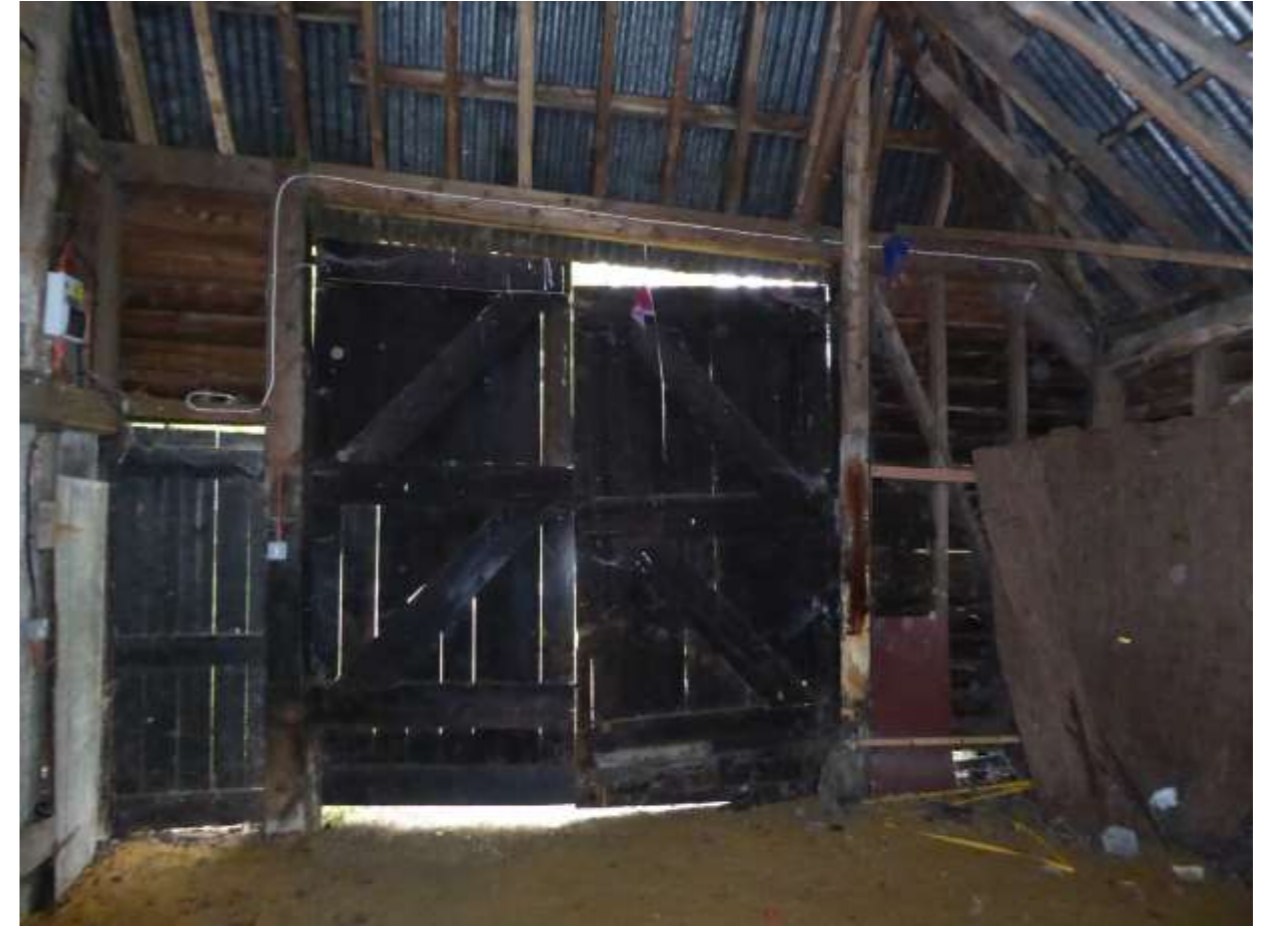
Photo 17: The internal west elevation of the northern part of the barn.
