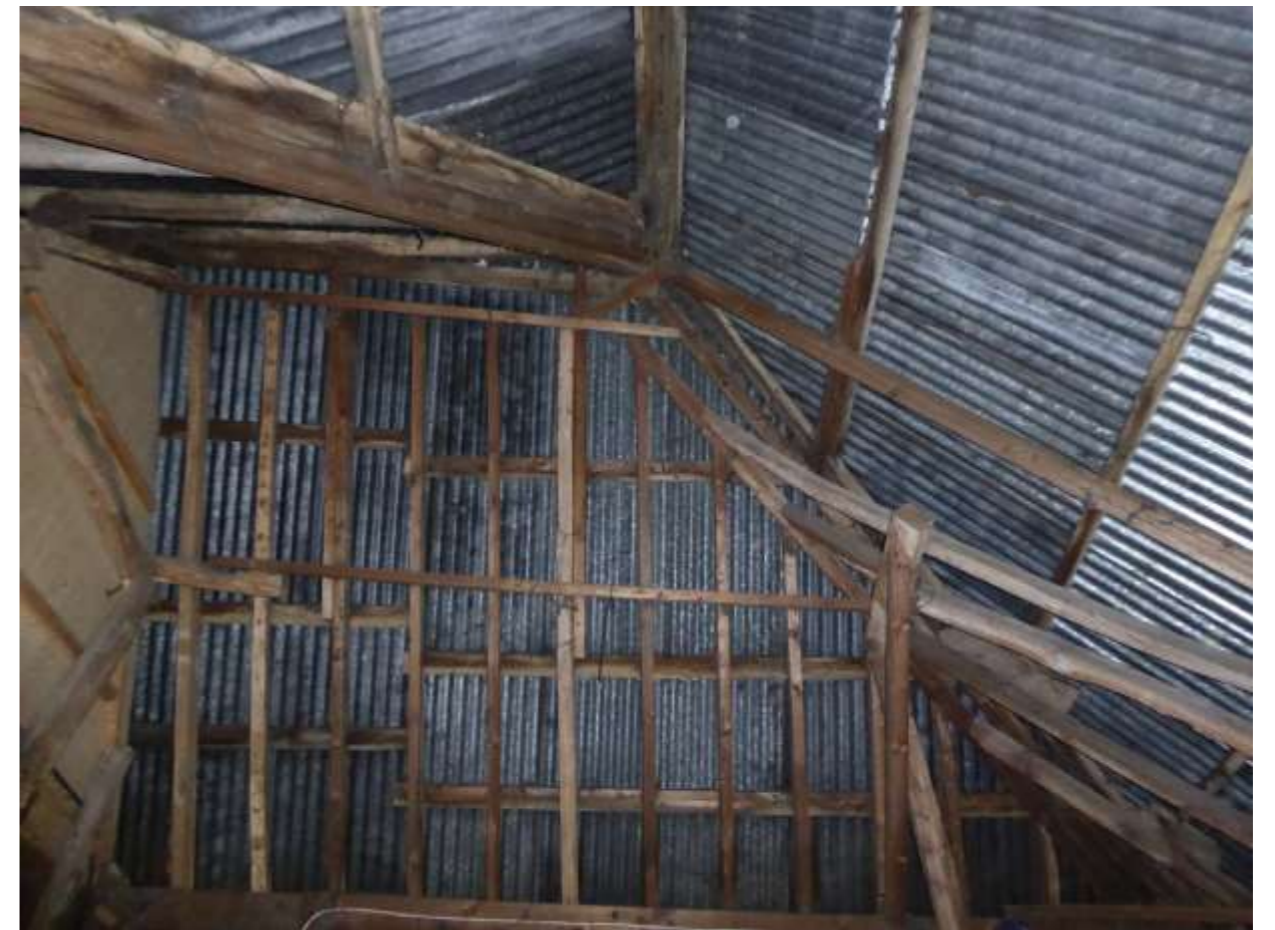
Photo 18: The roof structure in the northern part of the barn.
