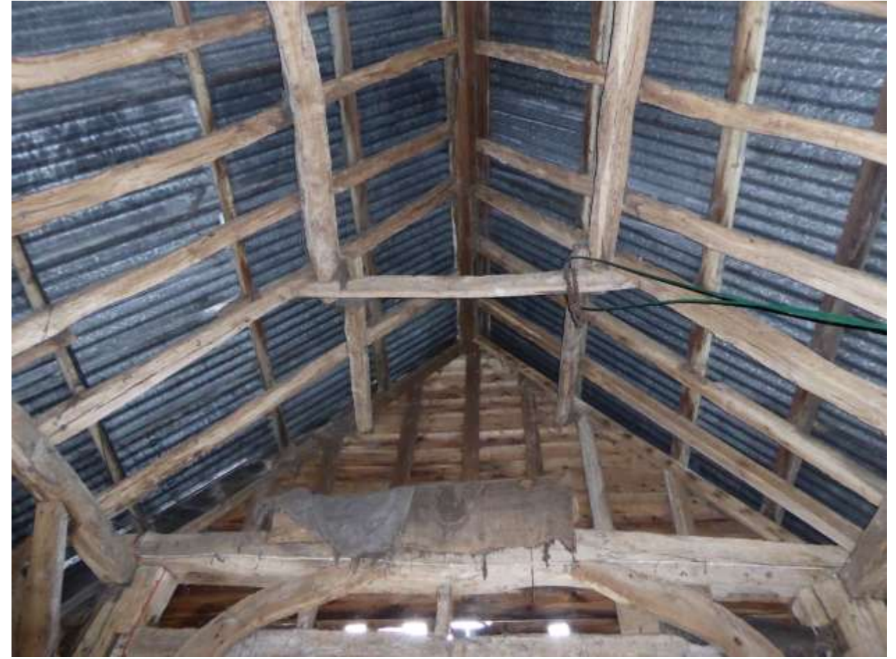
Photo 27: The internal southern gable of the barn.
