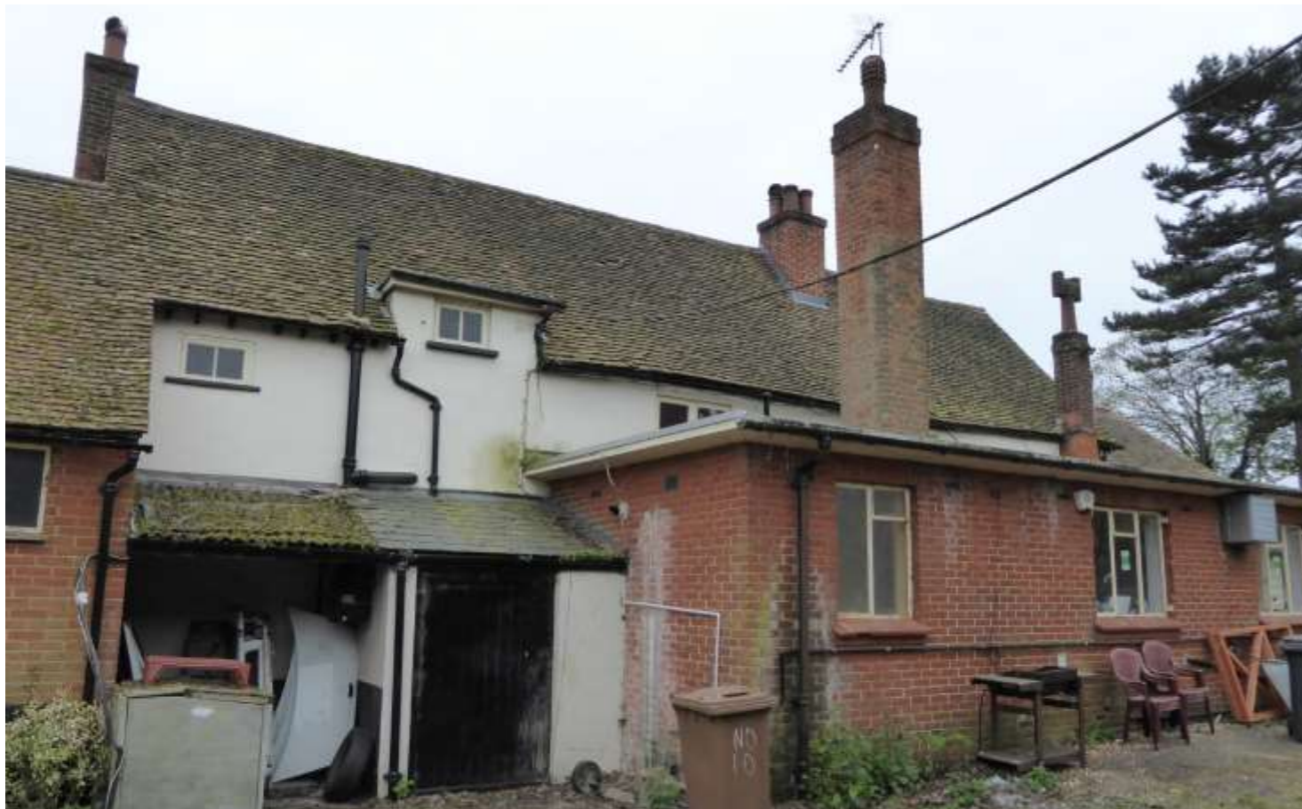
Photo 5: The rear of the pub, from the east.
