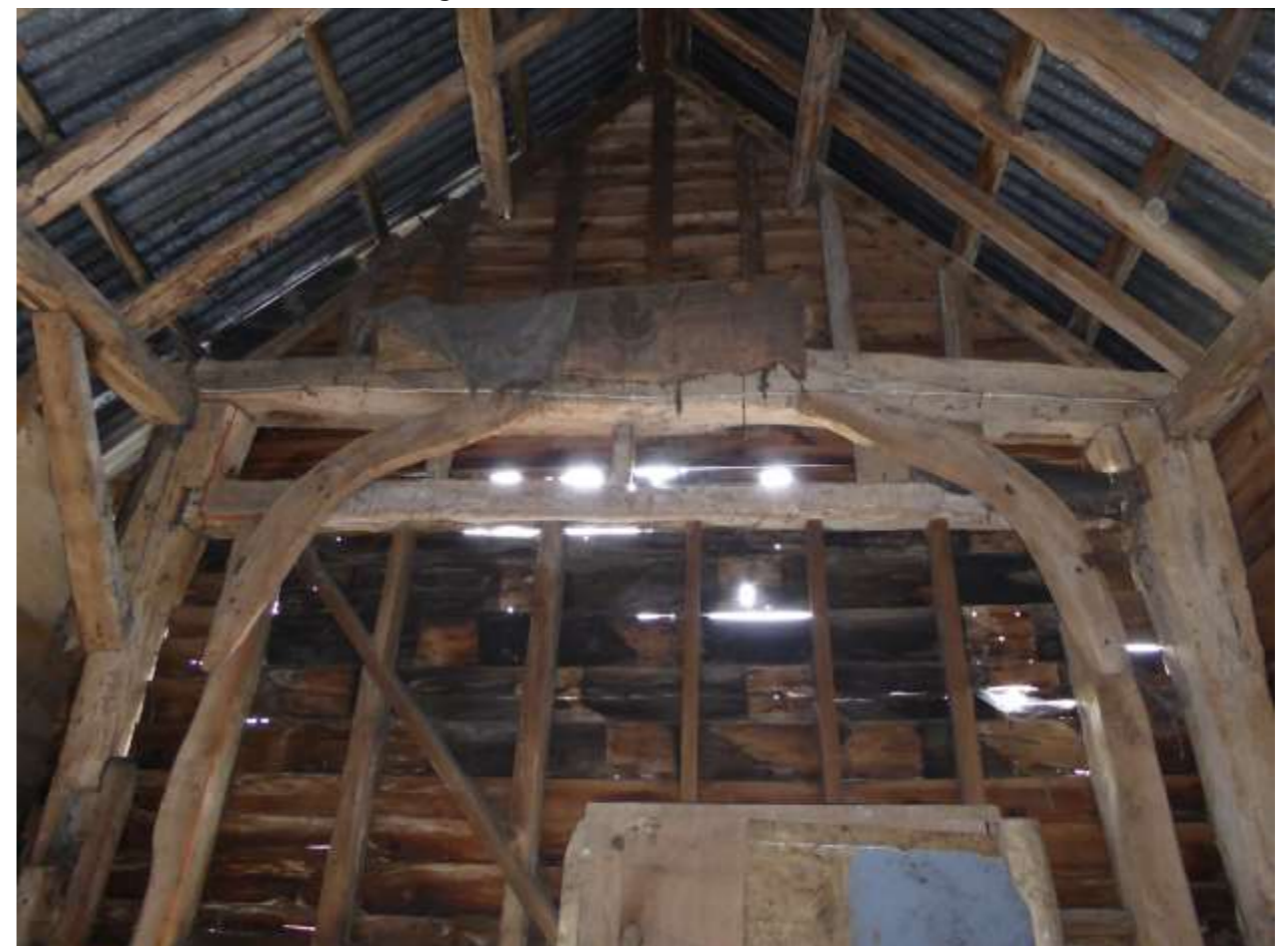
Photo 28: The internal south elevation of the southern part of the barn.
