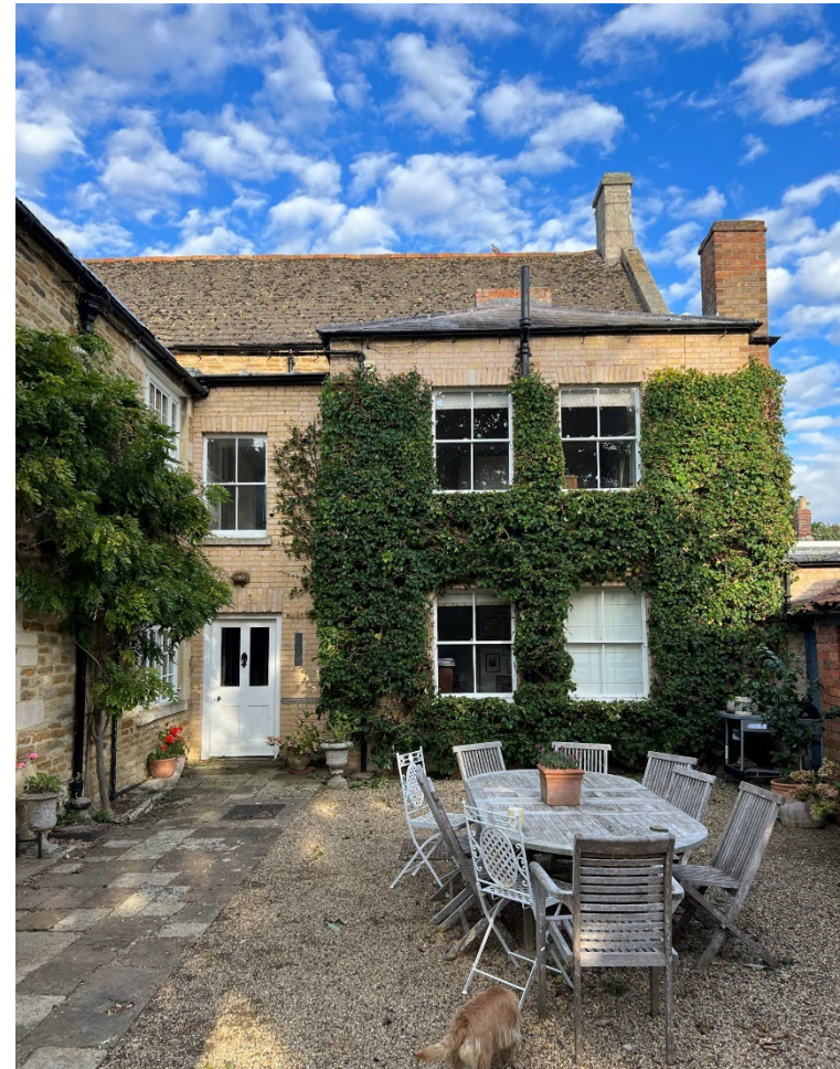
Image 8 Rear Modern extension, new extension location
