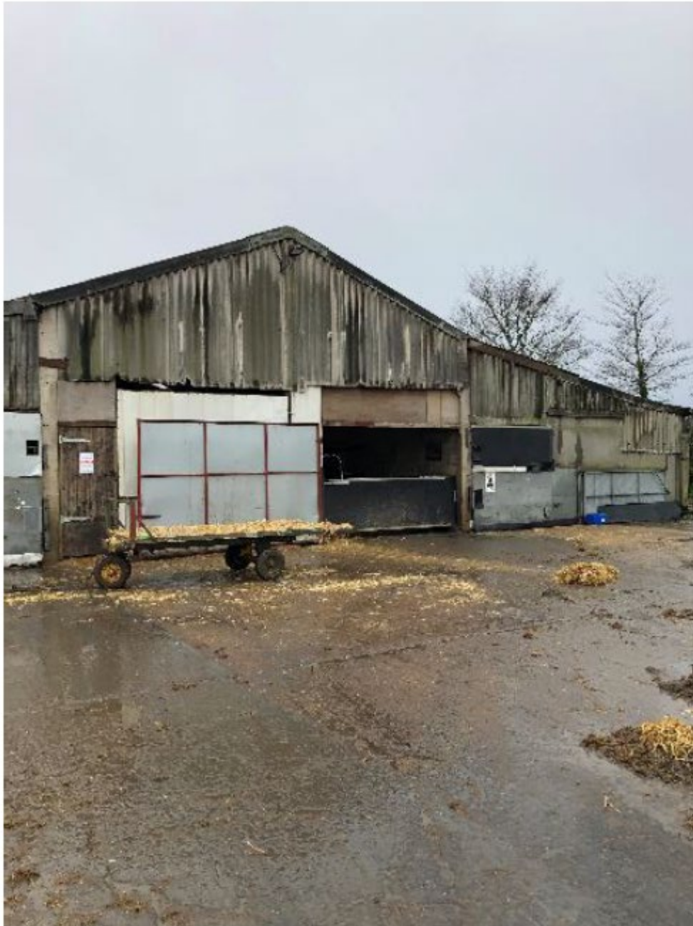
Photo 1: Northern elevation of Building A
