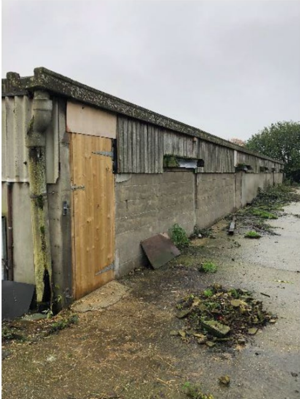
Photo 2: Western elevation of Building A
