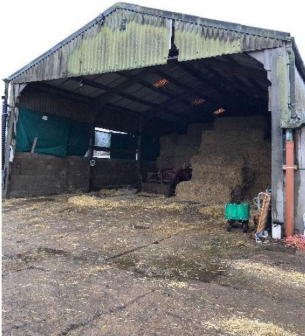
Photo 4: Northern elevation of Building B
