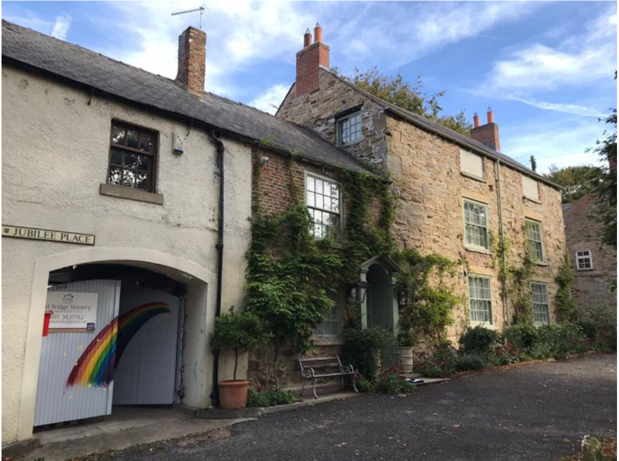
Photo of the Southern Elevations of Nursery and the Old House
