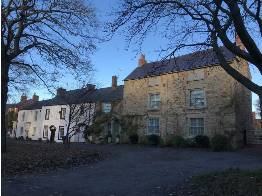
Photo of Wider Street Scene of Jubilee Place
