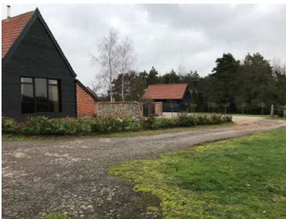
Barn seen from south west
