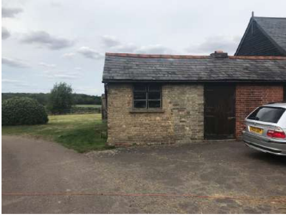
G. Existing south elevation of application site
