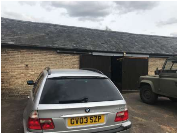
J. Existing west elevation of application site
