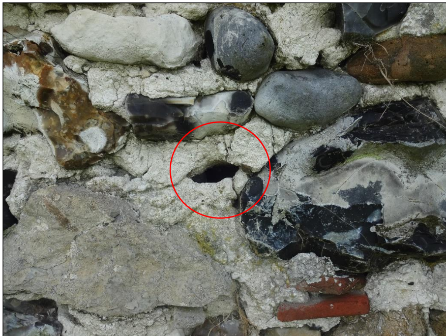
Photograph 6: View of potential roost feature in flint wall. 7 th May 2020.
