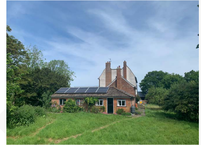
REAR OF THE STABLES
