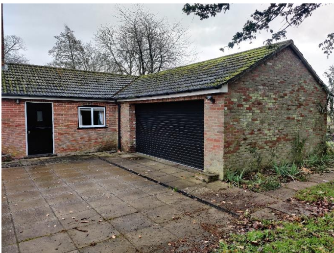
Photo 3 Northwest elevation of existing garage to be partly demolished
