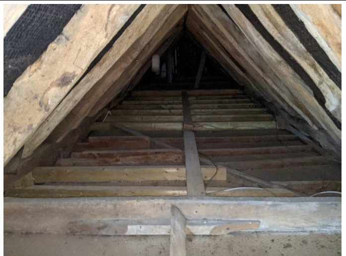
Photo 6 View of the loft above The Grange
