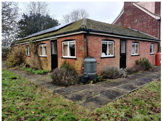
Photo 4 Southeast elevation of existing garage to be partly demolished
