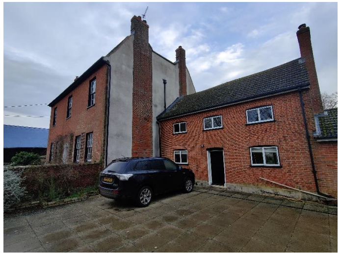
Photo 2 Southwest elevation of "The Grange" and attached cottage
