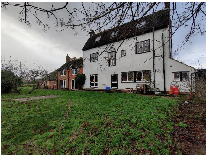
Photo 5 East elevation of The Grange and attached buildings
