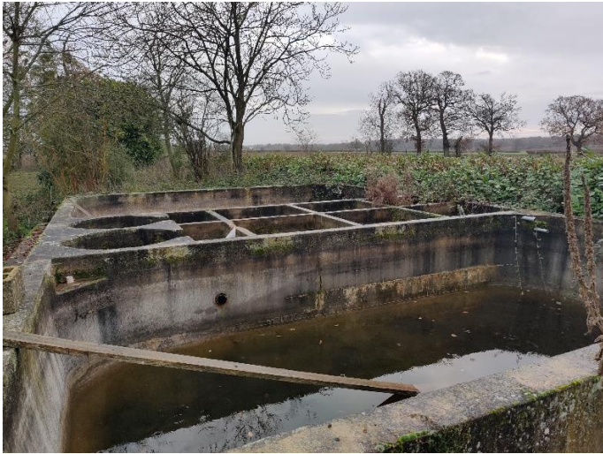
Photo 7 Concrete tanks previously used to rear fish
