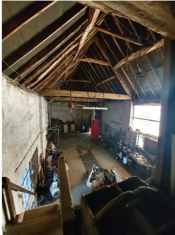
Photograph No. 7 – Internal view of building no. 3
