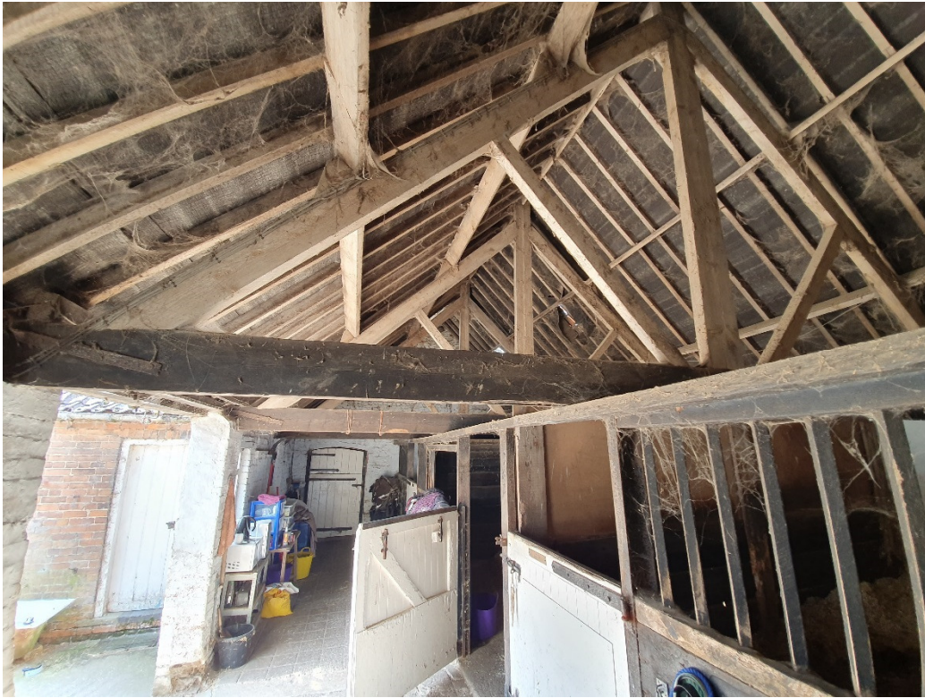
Photograph No. 1 – Roof to building No. 1
