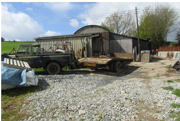
Plate 3. Side, eastern elevation of building.
