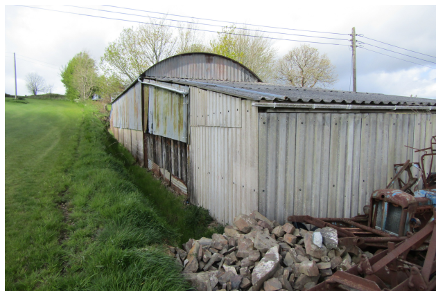
Plate 4. Rear, southern elevation
