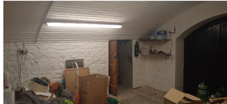
Inside the garage space showing 1500mm high door to entrance lobby
