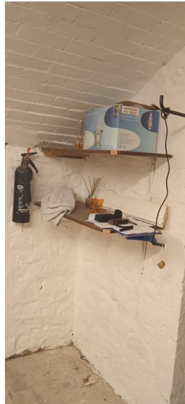
Lime washed stone and brick vault
