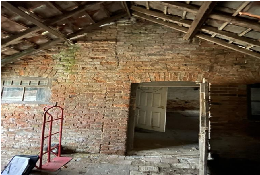
Photograph 7: Building 3 – southern elevation
