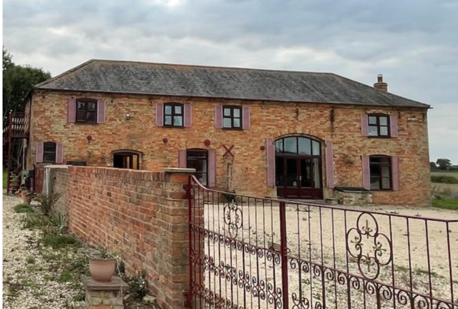
Photograph 1: Building 1 – Beechwood Barn eastern elevation
