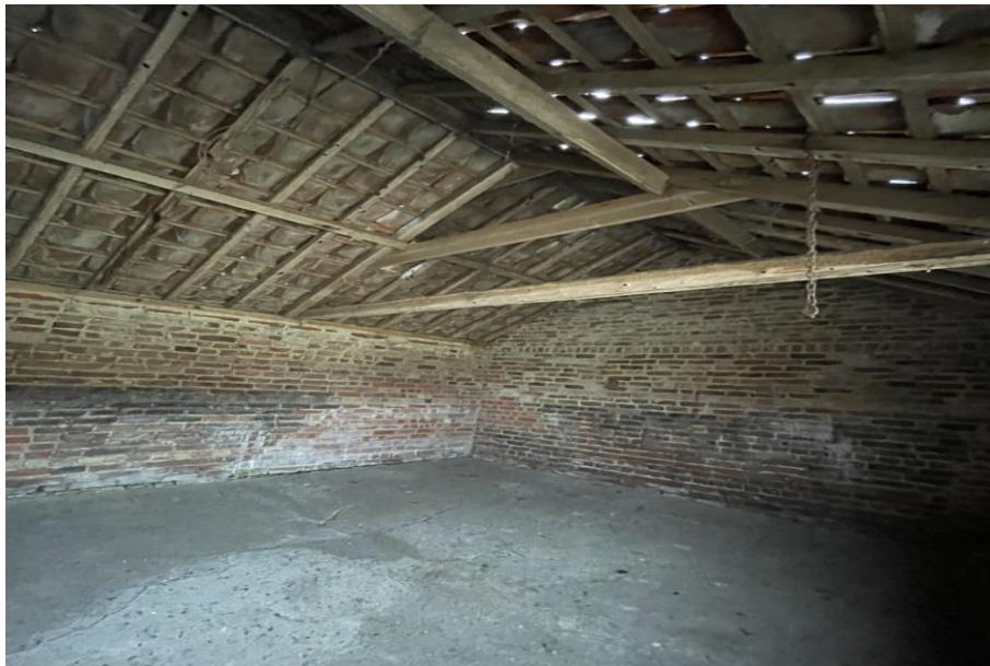
Photograph 14: Central room of building 4
