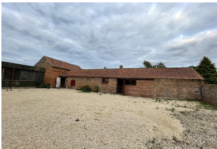
Photograph 12: Building 4 – western elevation
