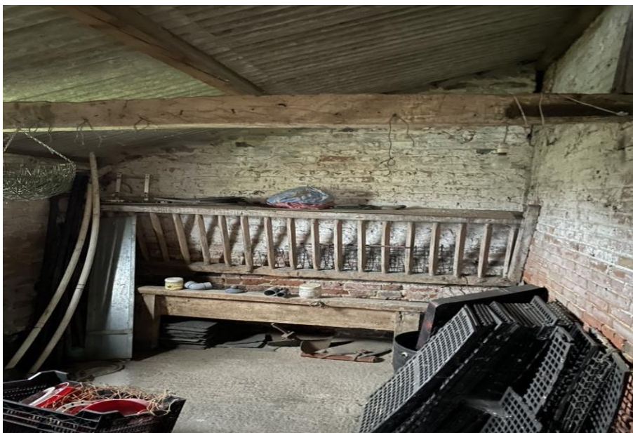
Photograph 6: Building 2 – internal view
