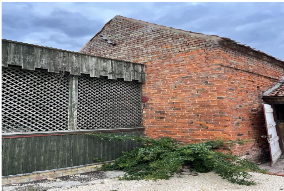
Photograph 8: Building 3 – western elevation
