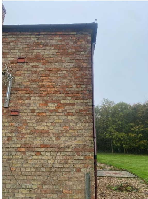
Photograph 23: Beechwood Barn – area where two bats were recorded emerging
