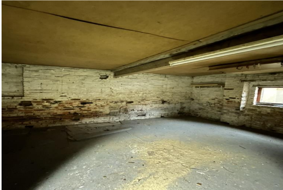
Photograph 13: Room at the northern end of building 4
