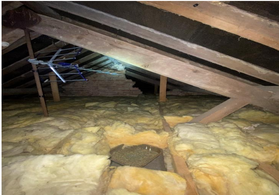
Photograph 2: Beechwood Barn – Loft void
