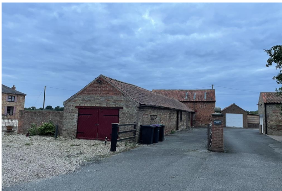
Photograph 11: Building 4 – southern & eastern elevations
