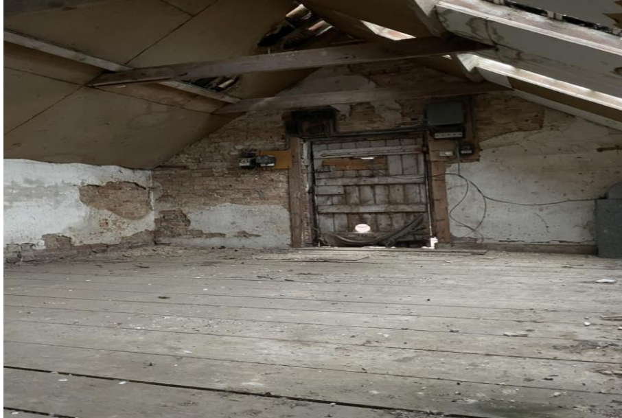
Photograph 9: Building 3 – Upper floor
