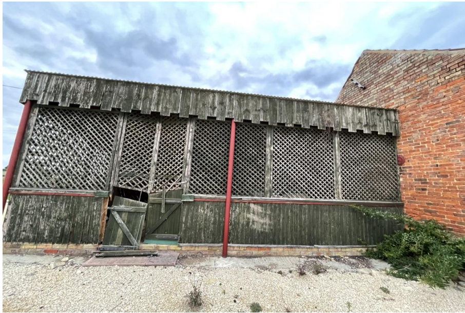
Photograph 3: Building 2 – southern elevation
