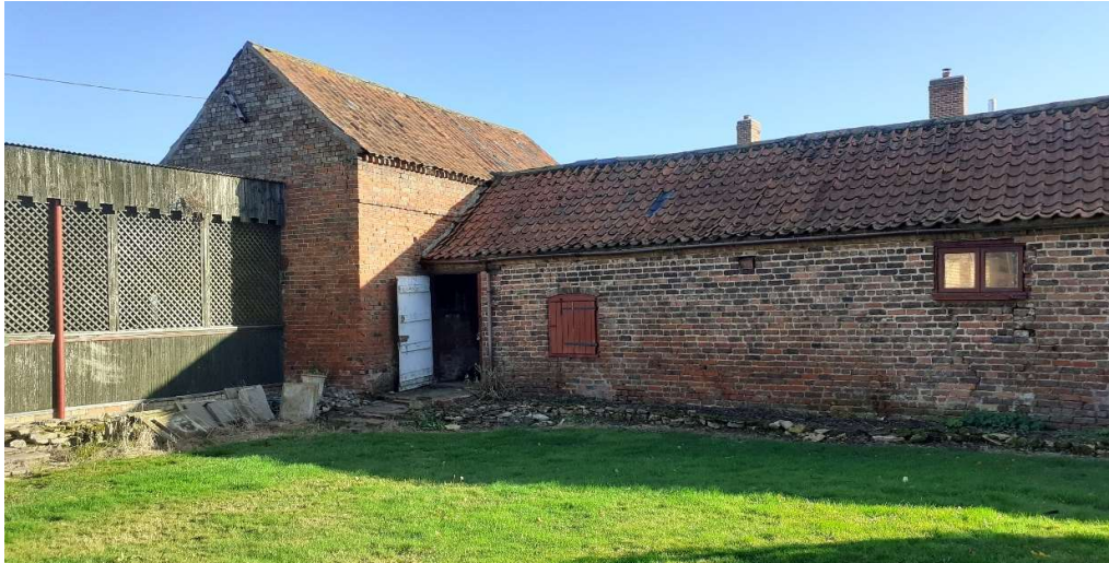
Photo 1: Existing Set of Brick Barns at Beechwood Barn, Martin.
