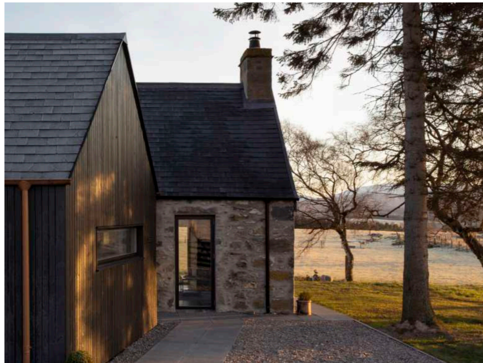
Example of black vertical timber clad extension alongside a existing traditional stone built cottage
