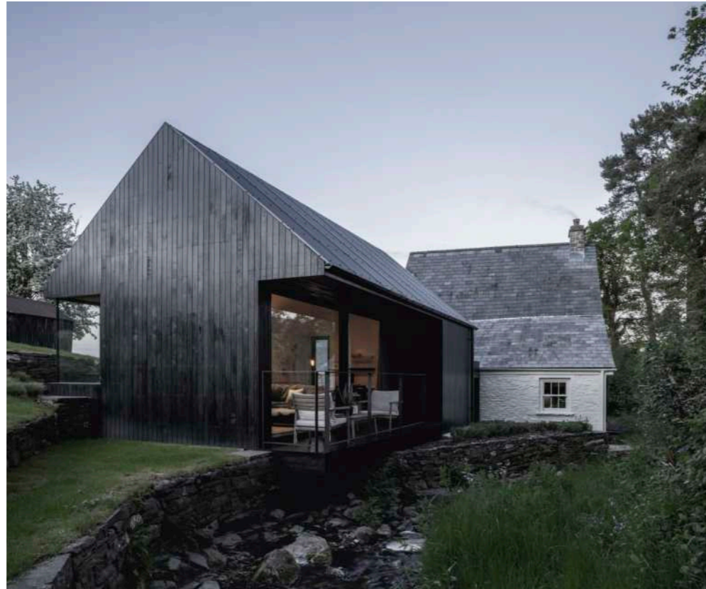
Example of contemporary corrugated sheet and black vertical timber cladding
