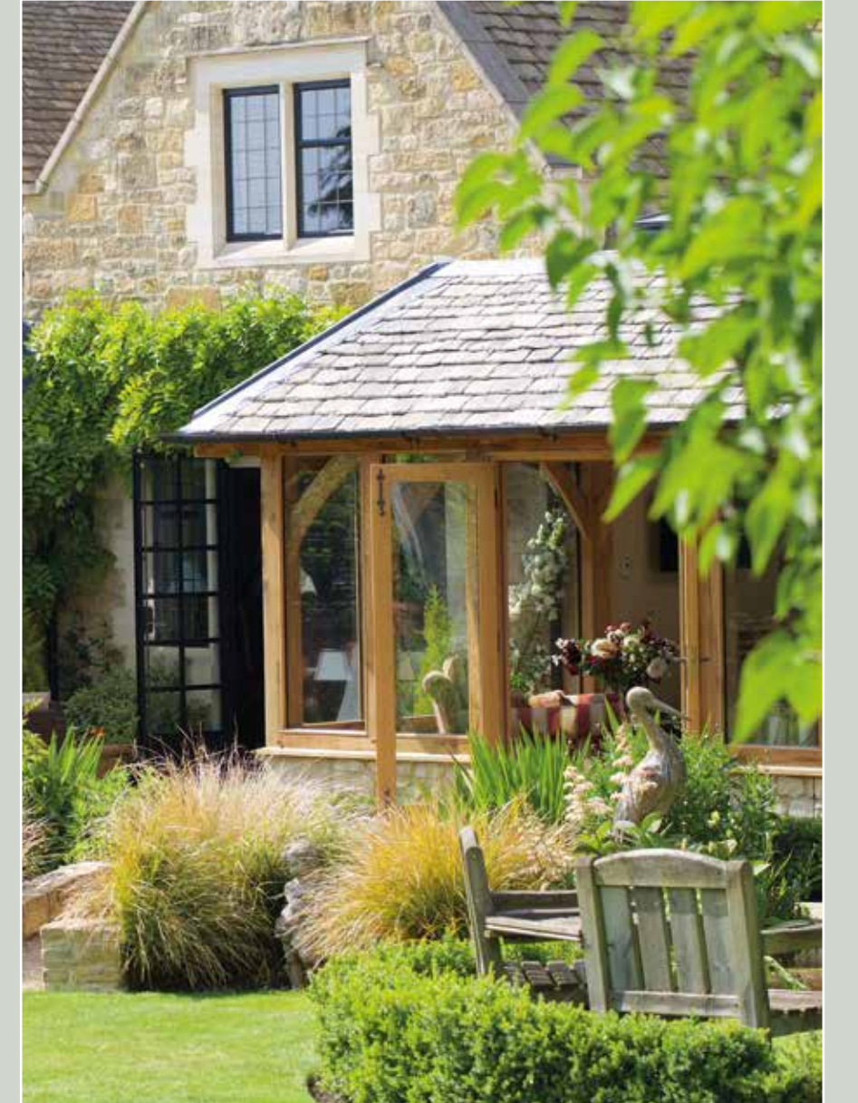
New Reproduction Cotswold Slates work well against the existing.
