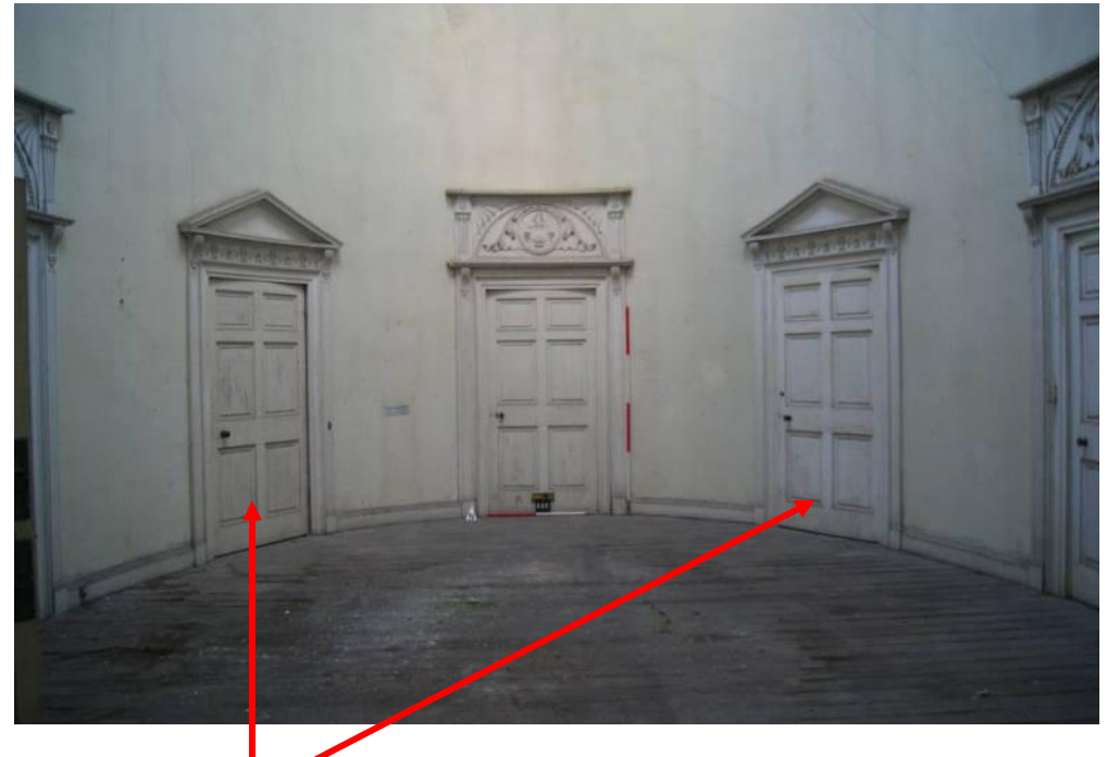
Cupboard doors on the north wall. The central door is false.
