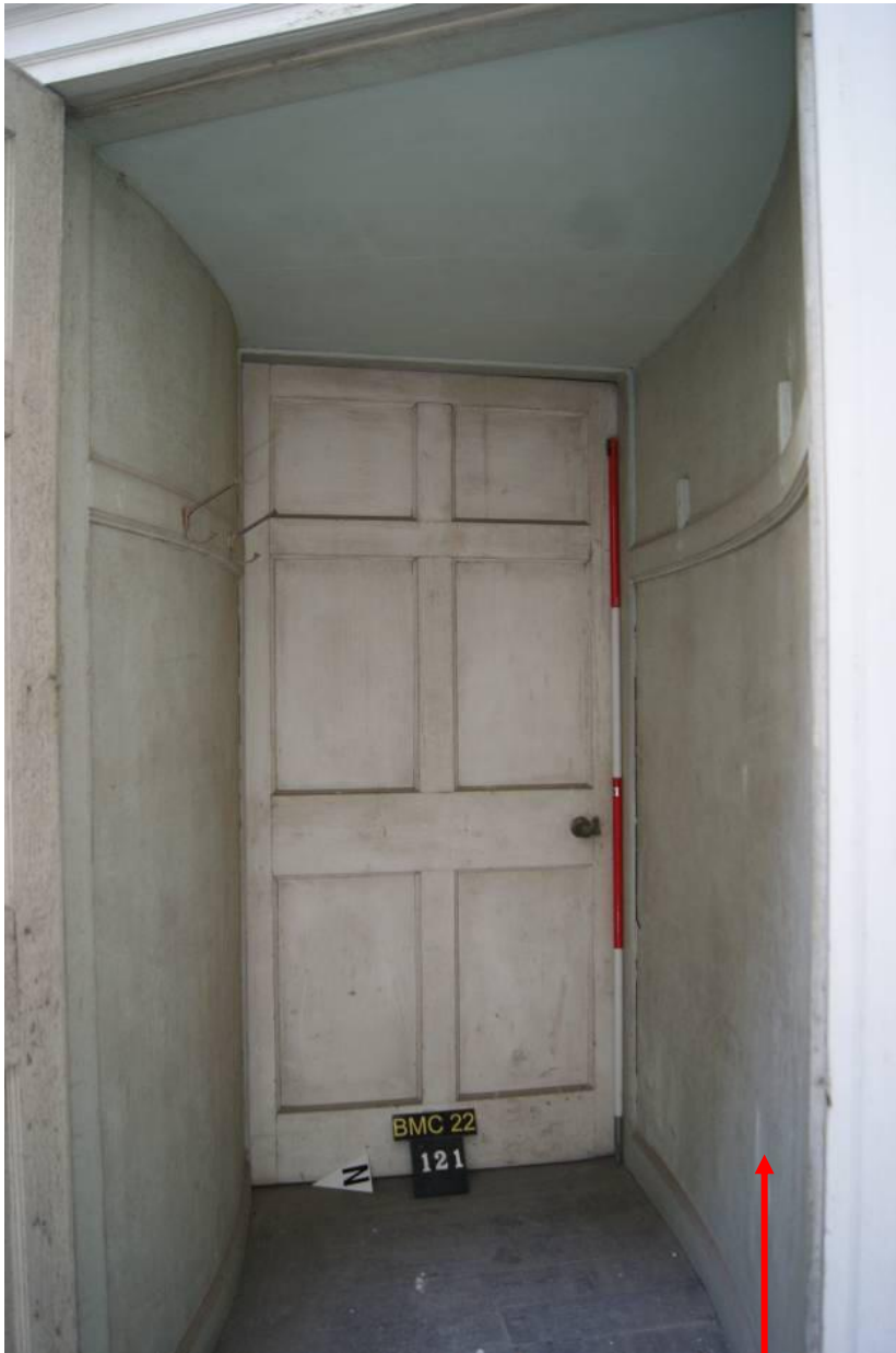
The corridor link between the two rooms. The investigative intrusion would be made in the curved wall on the right hand side and the coat hook curved batten would remain intact.
