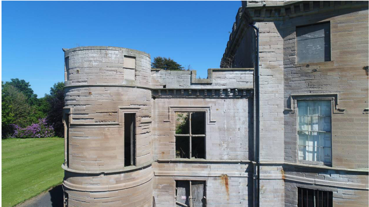
P21. Drone photograph of the west wall of the North Range at first floor level showing mullion and transom window [145], turret window [144] (left) and 'Eating Room' window [101] with 1801-4 curved sashes (right).
