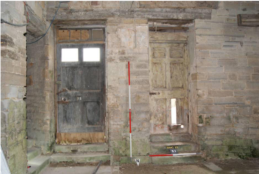
P55. R8 scullery south wall. A new doorway is proposed to be fitted in the opening into R13 (right). The remains of the first floor joists and boards to R40 survive above. The lower courses of masonry to the right of [31] dip down markedly, perhaps subsiding into
