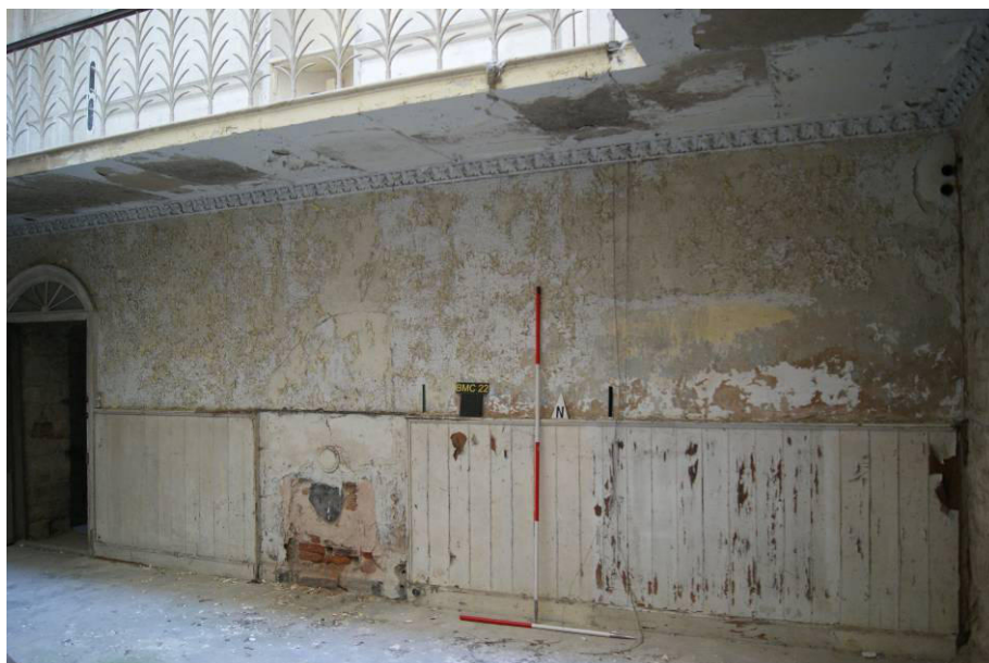
P59. R9 looking north-west to the site of blocked pre-1801 doorway [60], which is proposed to be re-opened. The position of the blocked doorway is marked by two black bars above the
