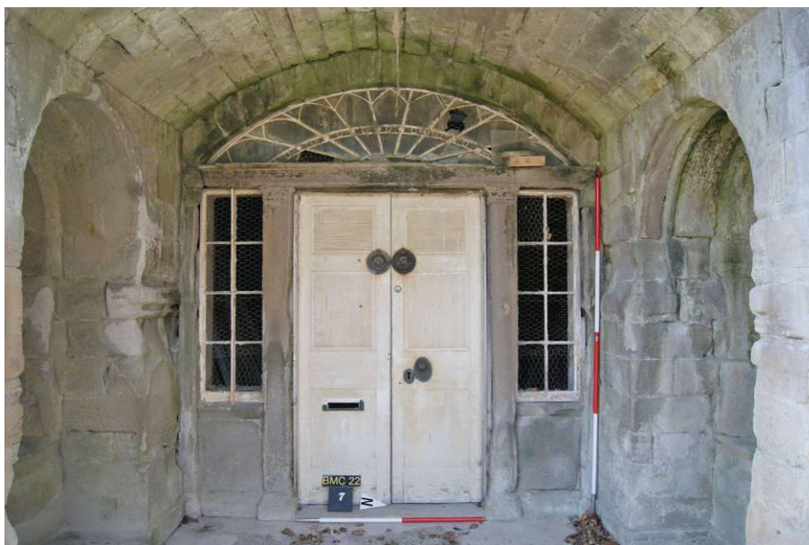
P9. East facade, principal entrance looking into the vaulted porch to screen wall [7] with double doors, overhead, and side lights divided by shallow pilasters possibly recycled from the pre-1801 building. Alcove niches in the north and south porch walls.
