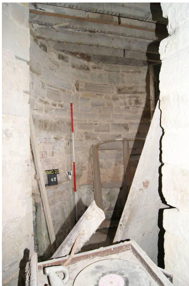
P64. R13, labelled the 'Pastry' on the 1801 floor plan. Looking west through [44], with detached fittings, blocked fire [47 (left)], and showing evidence for old
