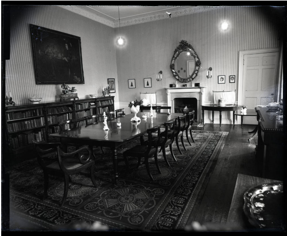
Fig.16. R42 looking north to fire [127] and door [126]. Country Life c.1960.
