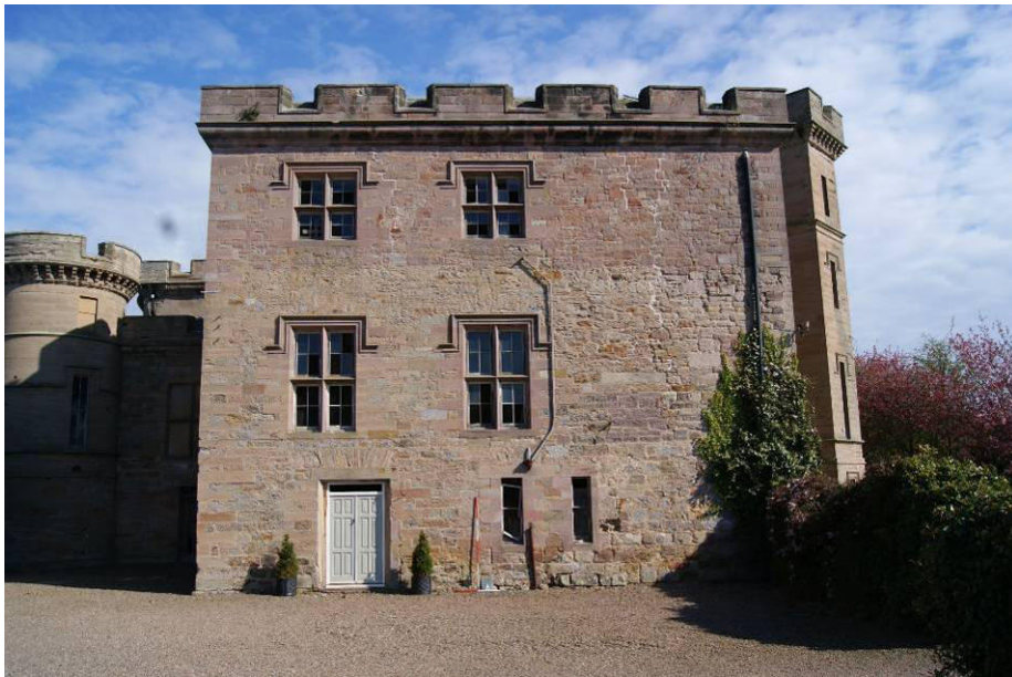
P28. South Wing south facade, showing the colour change in fabric from yellow-grey - which appears to be 1801-4 (right) but with some earlier (?late 18 th century) masonry,(left) - to the purple-red of the c.1892 raising to second floor level.
