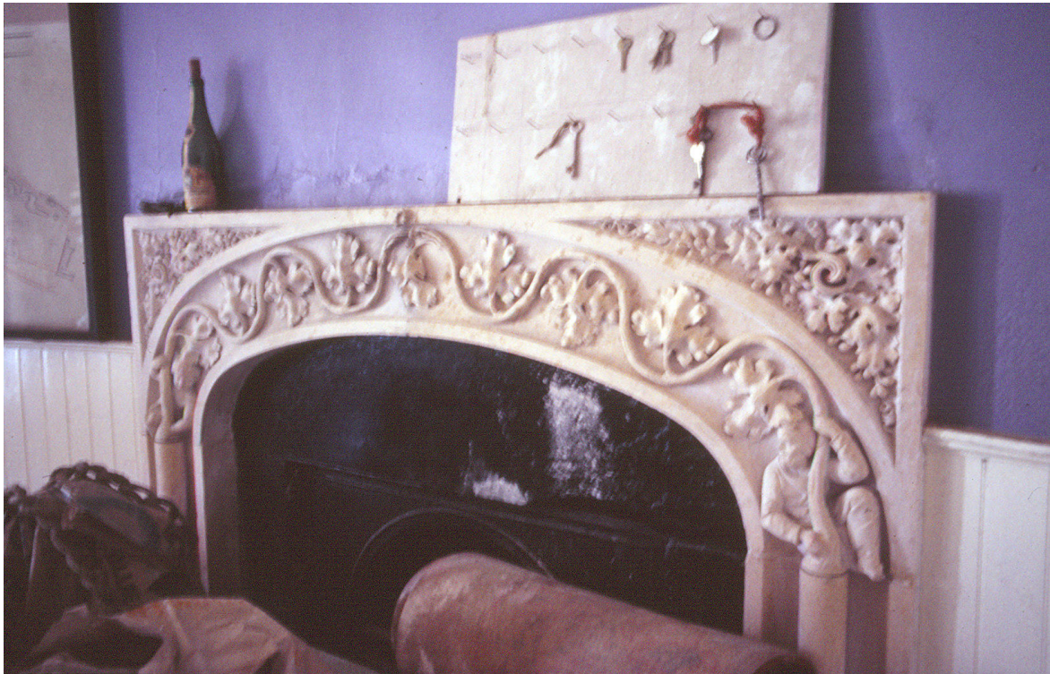
Fig. 45. Gatehouse, R10, c.1986, showing fire [197], plastered wall and matchboarding (J.Penn).
