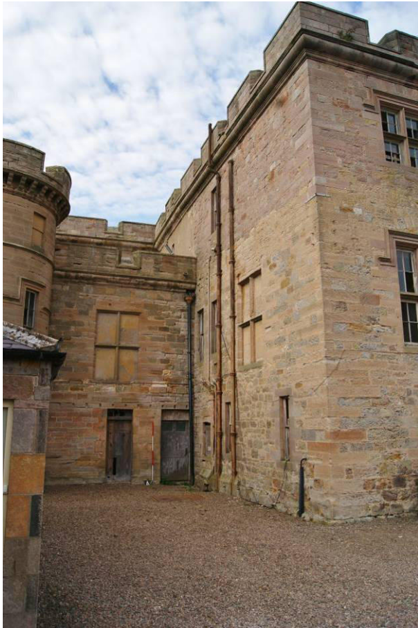
P23. South-west facade of the South Wing (left) and 1801-4 south facade showing doors [31] (originally a window) and [32], also 'blind' windows [153] and [161],
