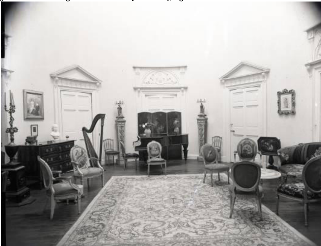
Fig. 15. R41 looking north to Doors [112-114], again c.1960.
