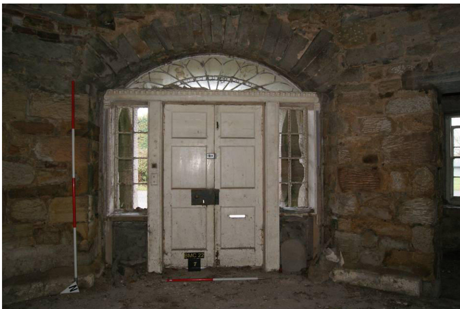
P63. R10 looking east to [7] showing the principal entrance doorway with flanking windows and overhead. Little changed since 2012. This feature will be restored.
