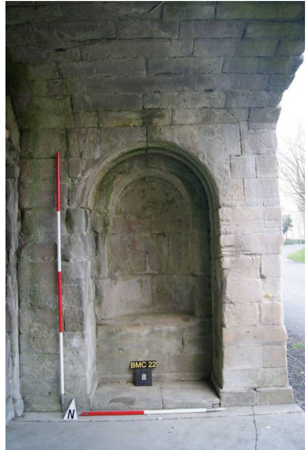
P13. East facade, north alcove of Gatehouse porch showing masonry again butting the screen wall [7], and also possibly containing reused masonry.
