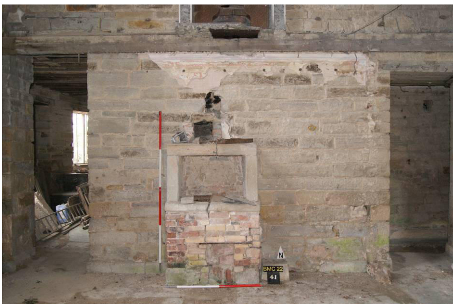
P56. R8 north wall of the scullery with a 'copper' [41], which is proposed to be removed, and doorways [41] and [42] either side. A new north-south partition is proposed to be inserted to the right of [41]. The stub of the 1801-4 partition wall can be seen beside [43].
