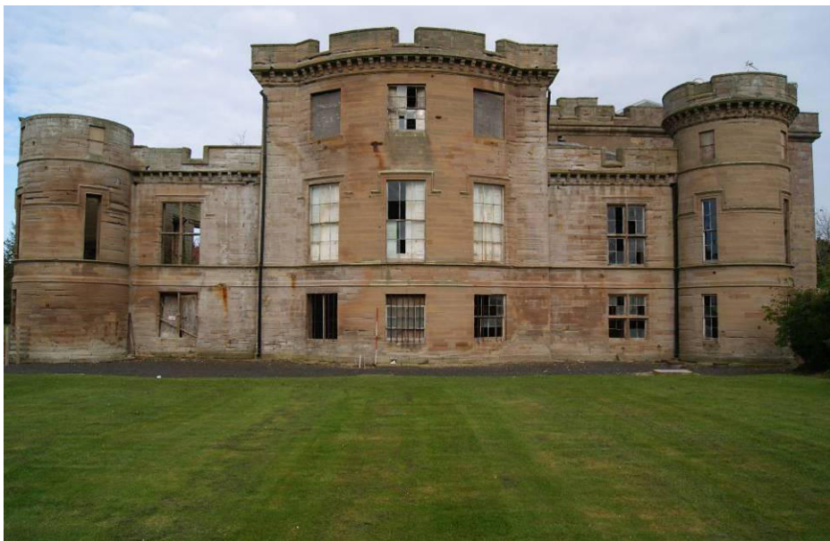
P20. West facade of the West Range of 1810-4, general view looking across the site of the infilled ornamental pond (which is proposed to be reinstated), showing barred ground floor kitchen windows [24-25], and tall sashes to the 'Eating Room' above [101-103].
