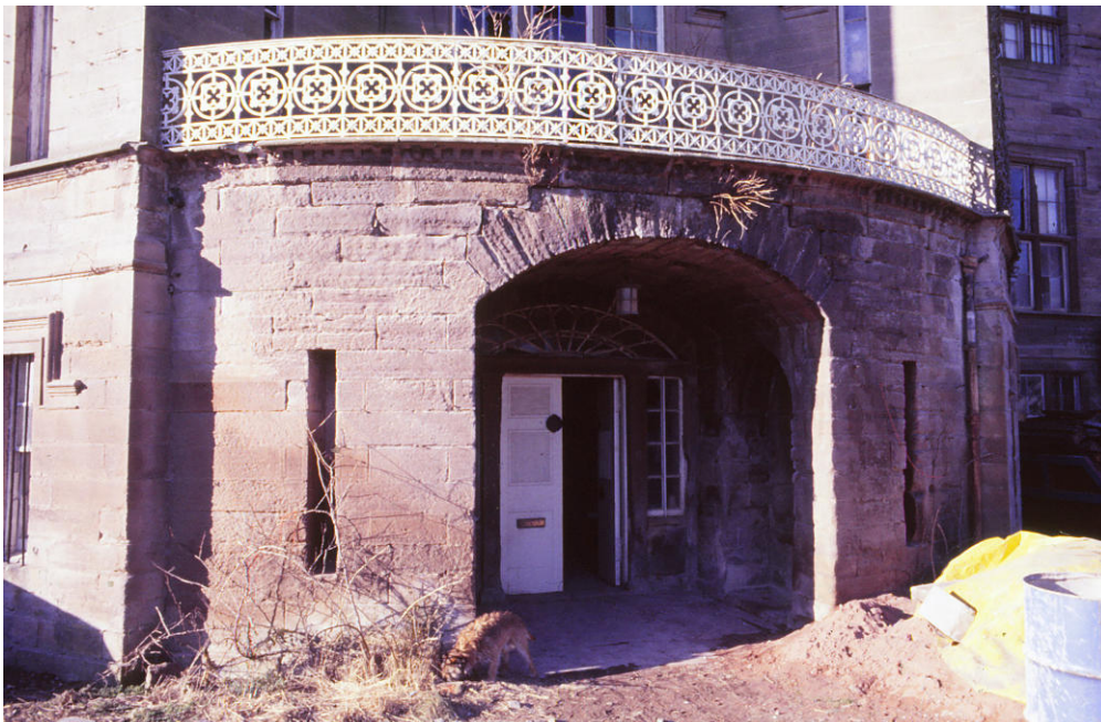
Fig. 42. The bow-fronted porch, balcony and front door [[107] c.1986. (J.Penn)
