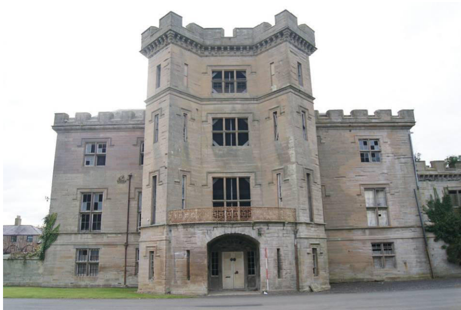
P3. East facade, dominated by the four-storied Gatehouse. To the south (left) the raising to second floor level of c.1892 is distinguishable by its use of red sandstone.
