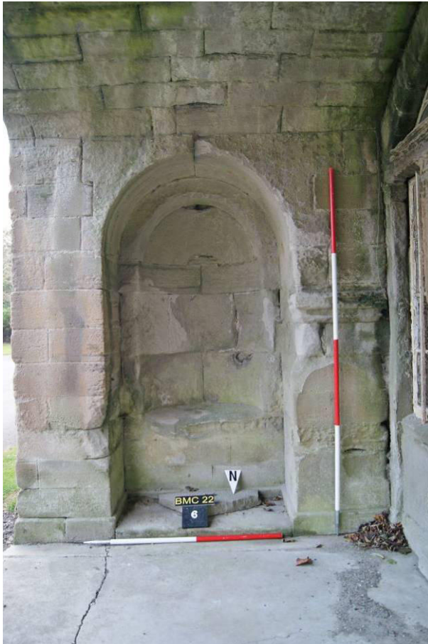
P12. East facade, south alcove of Gatehouse porch showing masonry, some possibly reused from the pre-Paterson 'House', butting the screen wall [7].
