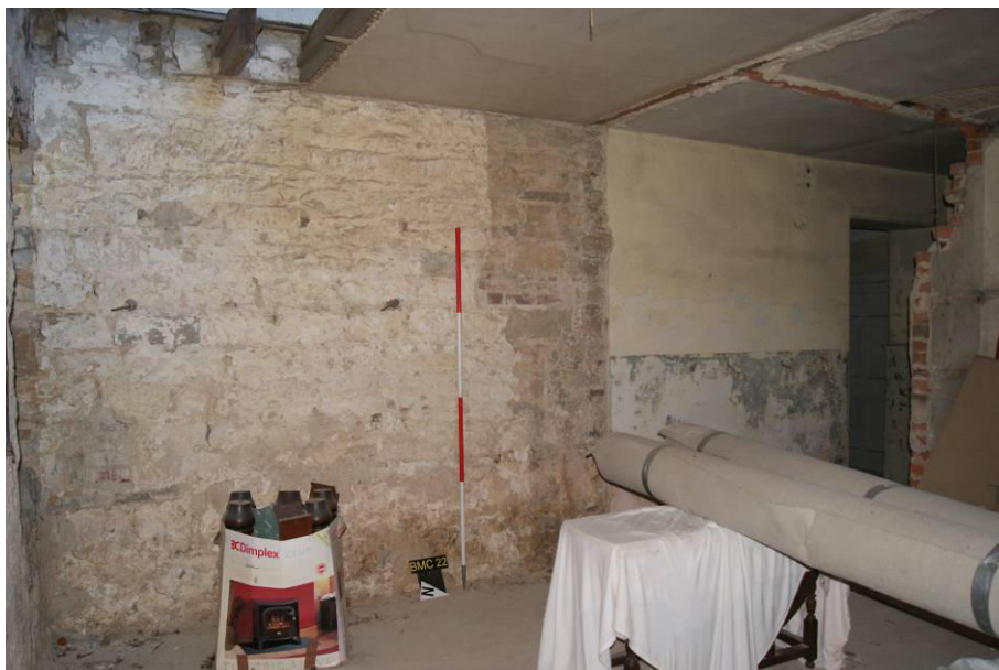
P49. R5. Looking north-west to the site of a proposed new doorway from R2, where render (R4) changes to exposed masonry. This wall was suggested in 2012 to be a thinned medieval feature but it now appears most likely to be 1801-4.
