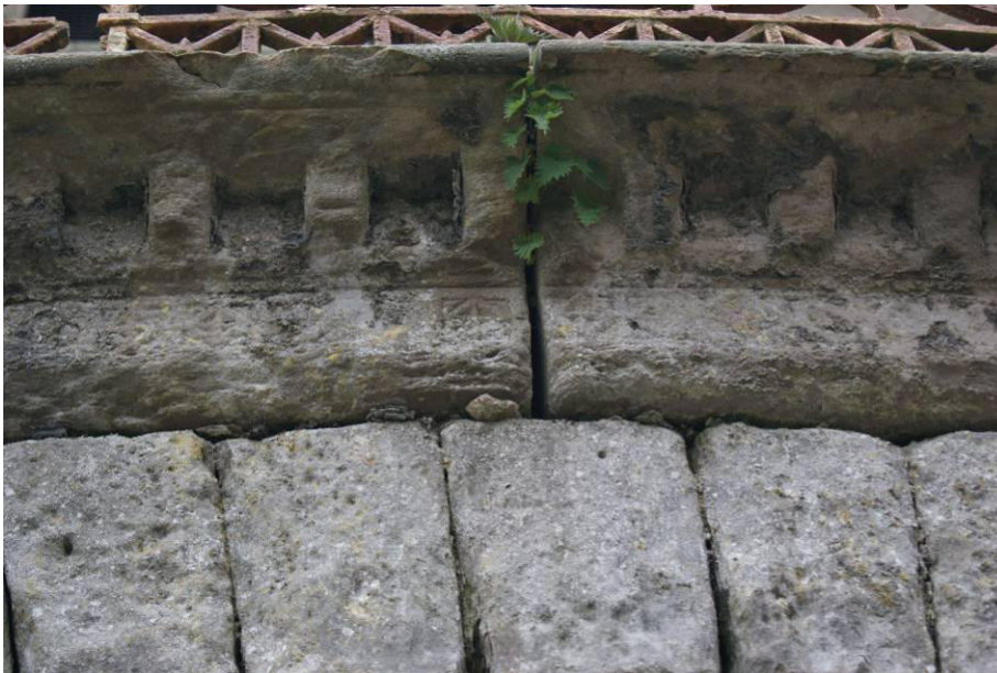
P8. East facade balcony. Detail of the moulded cornice to the balcony showing dentils above a badly-weathered frieze of square panels with raised lozenges and crosses – see enlargement below. Slivers of slate and stone used as levelling pieces can be seen above the arch voussoirs.
