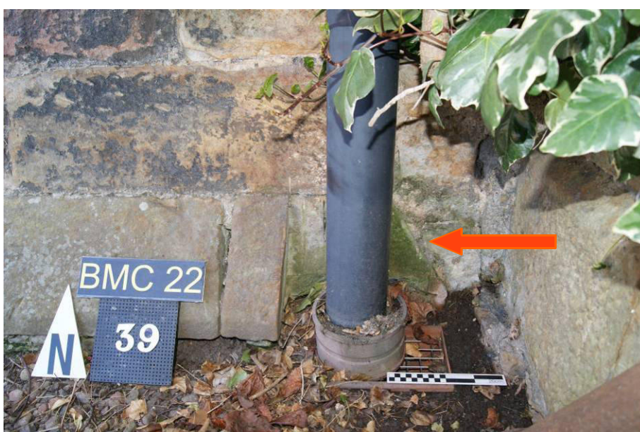
P34. South facade. The south-east corner of the chamfered plinth [39]. The chamfer has been cut back with a Stihl saw to insert the UPVC downpipe, but the angled face of the northward-returning chamfer can be seen behind the pipe (arrowed).
