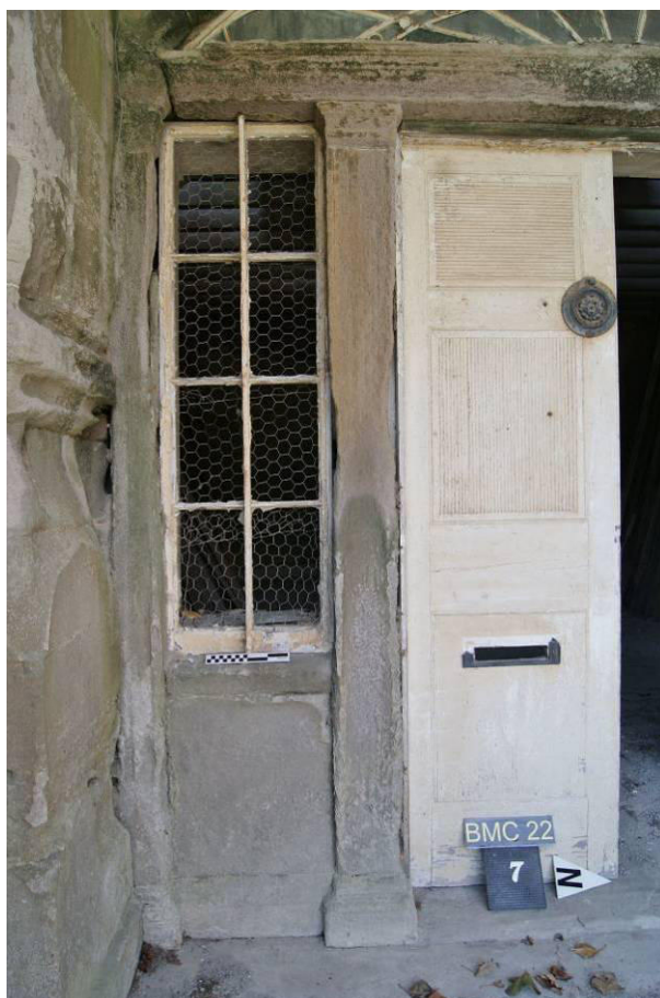
P9. East facade, principal entrance looking into the vaulted porch to screen wall [7] with double doors, overhead, and side lights divided by shallow pilasters possibly recycled from the pre-1801 building. Alcove niches in the north and south porch walls.
