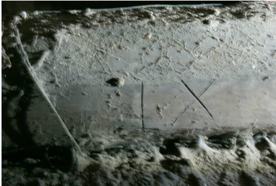
P175. Attic space R72. Assembly or timber-merchant's mark on the principal of truss [314].
