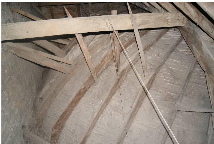
P176. Roof space R76, looking from R72 onto the inner surface of the cupola over the Great Stair, showing laths attached to shaped ribs, with some possible old patched repairs.
