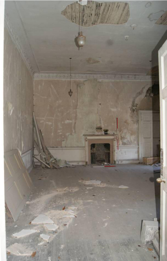
P126. R42 'Billiard Room' in 1801. Room view looking north to fire [127] showing ceiling plaster fallen since 2012. This is proposed to remain a
