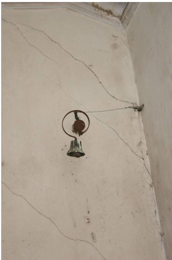
P144. R52. Servant's sprung bell and bell crank above the Service Stair on the south wall. Features like this will be retained within the proposed conversion.
