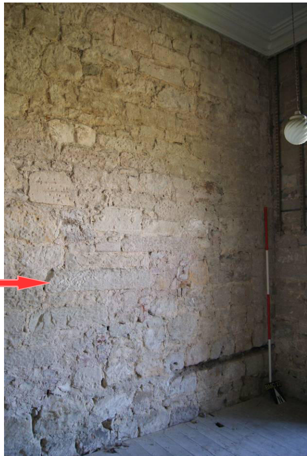
P106. R30. North wall looking north-east showing exposed masonry with apparently truncated stone stair treads as in R6 (arrowed) and a raking line of hand-made brick inserts which possibly mark the site of a later 18 th century timber stair.
