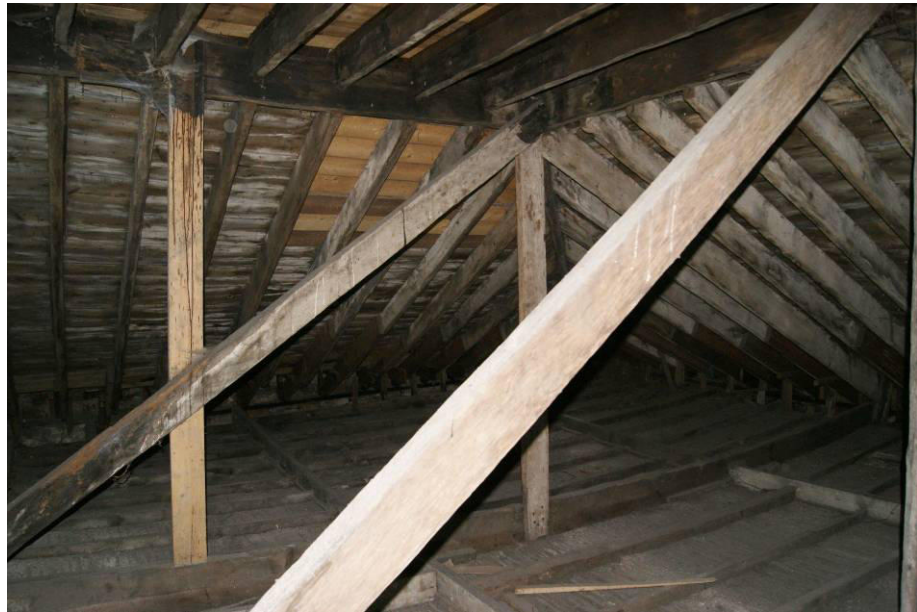
P172. Attic space R72 looking north showing trusses [313] and [314]. The joists to the ceiling of R62 below show evidence for deflection on the tie-beams. Loft hatch [236] is at bottom left.
