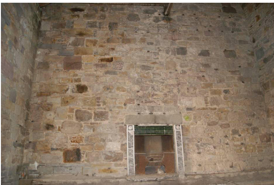
P114. R39 looking north to fire [157]. The rubble masonry appears to be 1801-4, and shows differences in size of material used on the west and east sides. It is not clear if this reflects Sitwell economies, or has any dating significance. A new opening is proposed to be inserted left of the fire.
