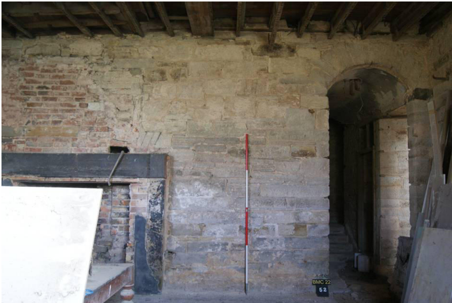
P67. R14. East wall between doorway [52] (right) and fire [50], showing lower long, purple-grey ashlars with the remains of a relieving arch cut by [50], and yellowish sandstone rubble above.
