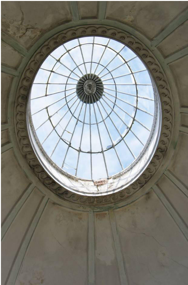
P124. R41, the glazed cupola over the Oval Saloon. Some minor delapidations since 2012 are apparent, largely a result of Storm Arwen which resulted in the shard of glass embedded in the floorboards
