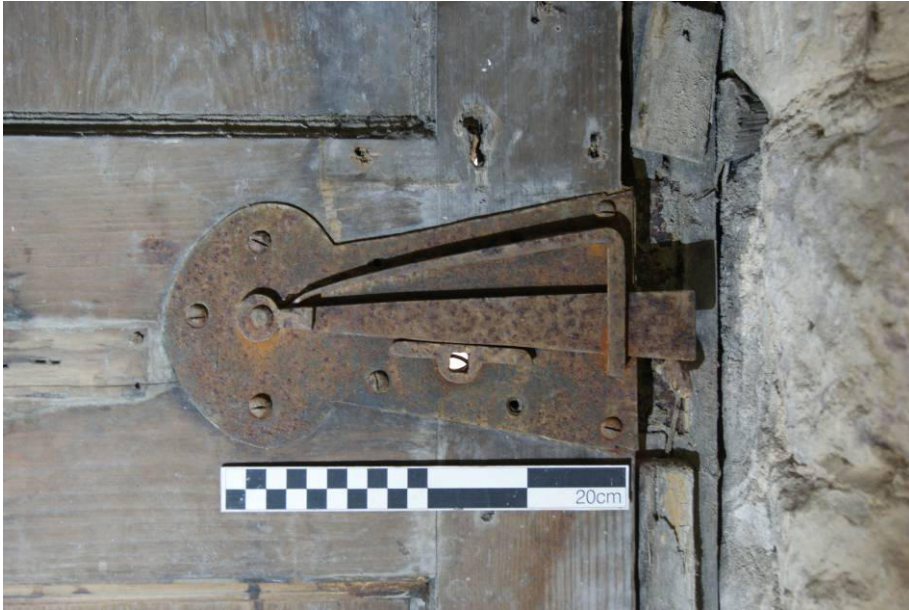
P98. R8.2 Detail of the early 19 th century spring catch on the inside of door [107].
