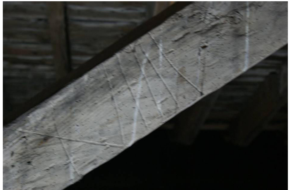
P176. Roof space R76, looking from R72 onto the inner surface of the cupola over the Great Stair, showing laths attached to shaped ribs, with some possible old patched repairs.
