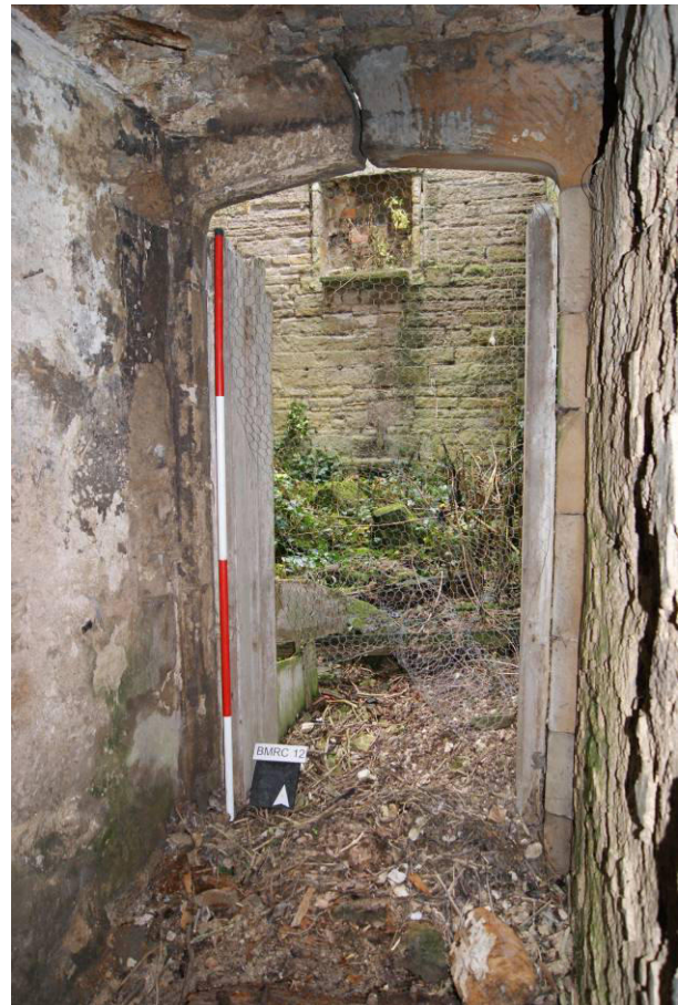
P78 - 79. R19. 'Servants Hall'. Doorway [64] in 2022 (left), showing that significant deterioration has occurred since it was photographed in 2012 (right).
