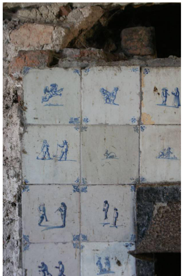
P155. R57. Tin-glazed 'Delft' tiling around fireplace [231], with detail of patterns (left) The surround is unlocated.
