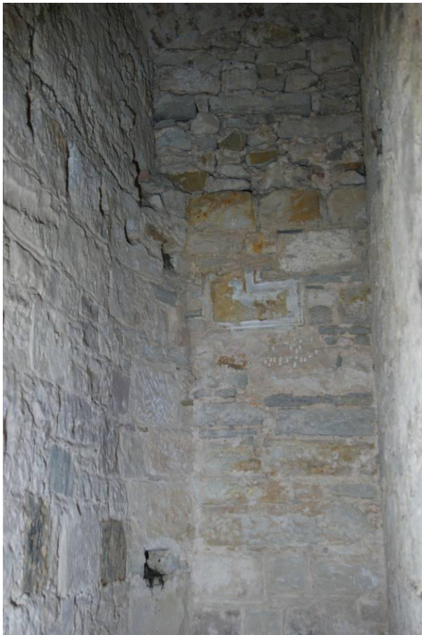
P96. R8.2 Fragment of ?17 th century fire surround reused in 1801-4 fabric at First floor level in the south wall of the mural stair.
