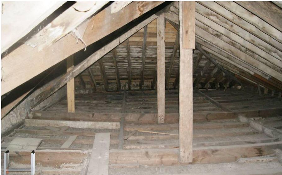
P173. Attic space R72 looking south with framing and supports of the Great Stair cupola in the distance. This shows part of a fossilised gable [313] from the pre-Paterson 'House' and a possibly 18 th century tie-beam
