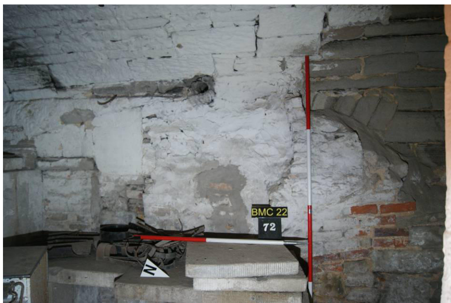
P71. R15. 'Cellar' on the 1801 floor plan. The west wall, showing patching and remains of voussoirs of an earlier arched opening [72] behind the 1801-4 stone larder shelving.
