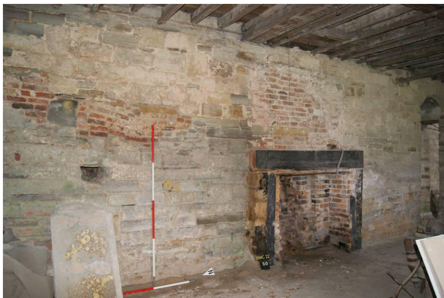
P66. R14 the 'Kitchen' on the 1801 floor plan. East wall looking south-east showing changes of masonry and ?early 19 th century brick patching. The lower grey ashlar probably pre-date 1801-4.
