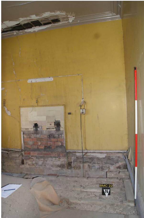
P106. R30. North wall looking north-east showing exposed masonry with apparently truncated stone stair treads as in R6 (arrowed) and a raking line of hand-made brick inserts which possibly mark the site of a later 18 th century timber stair.
