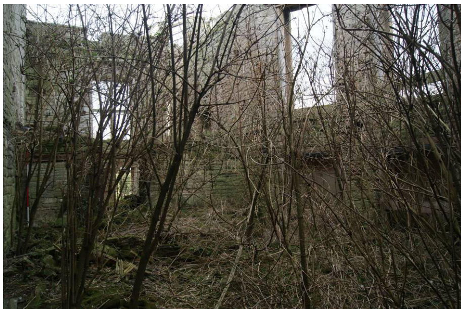
P91. North Range. R22 looking west. This area is proposed for a new 'freestanding' 'house', with a patio in the bay front (right). The lower part of a dividing wall demolished in 2013 is just visible. Since 2012 extensive undergrowth, principally elder, has rooted in the debris covering the floor.
