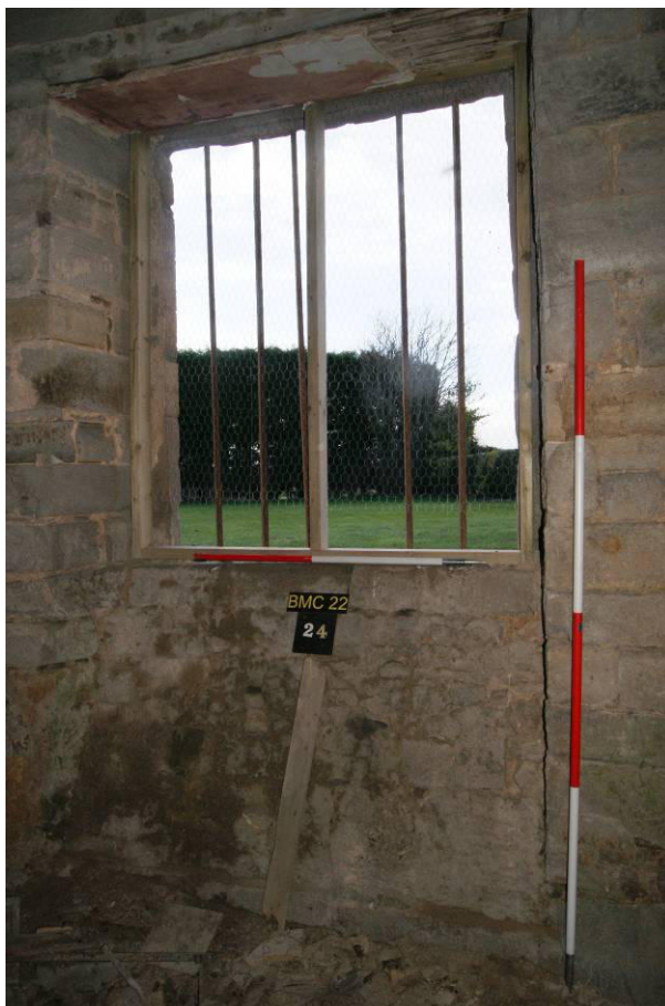
P68. R14. West wall window [24,], which has lost its frame and glazing since 2012. External iron bars are visible. Right - mason's marks on exposed jamb stones in the window reveals. This is proposed to be in a patio area.
