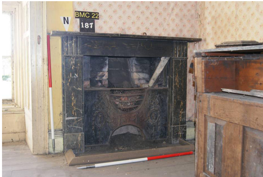
P100. R27, part of the c.1892 remodelling, looking south-west to fire [187]. The hob grate is earlier and may have been repositioned.
