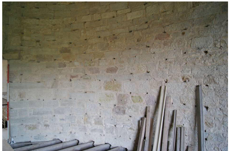
P114. R39 looking north to fire [157]. The rubble masonry appears to be 1801-4, and shows differences in size of material used on the west and east sides. It is not clear if this reflects Sitwell economies, or has any dating significance. A new opening is proposed to be inserted left of the fire.
