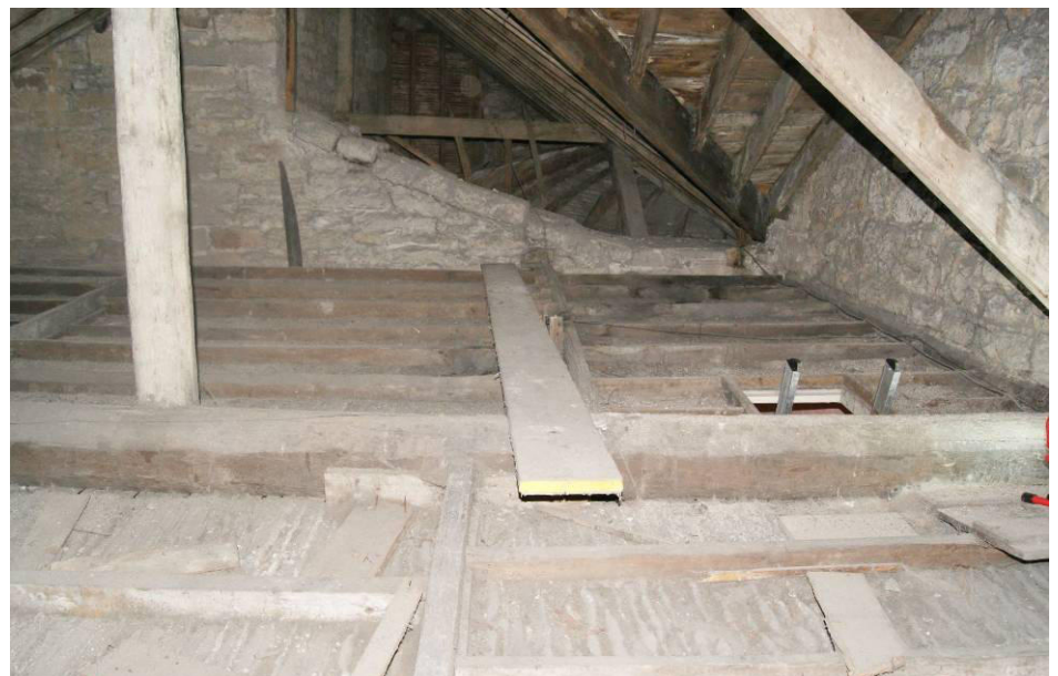
P173. Attic space R72 looking south with framing and supports of the Great Stair cupola in the distance. This shows part of a fossilised gable [313] from the pre-Paterson 'House' and a possibly 18 th century tie-beam
