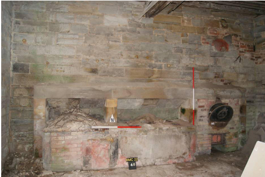
P70. R14. 'Kitchen'. The 1801-4 stewing range. Detail of right-hand part of the range with five 'pots' and a smoke vent above.
