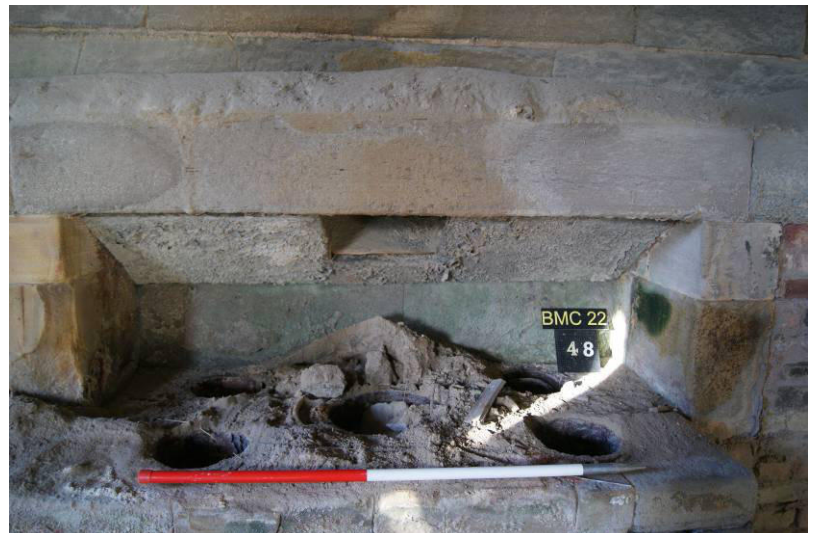
P71. R15. 'Cellar' on the 1801 floor plan. The west wall, showing patching and remains of voussoirs of an earlier arched opening [72] behind the 1801-4 stone larder shelving.
