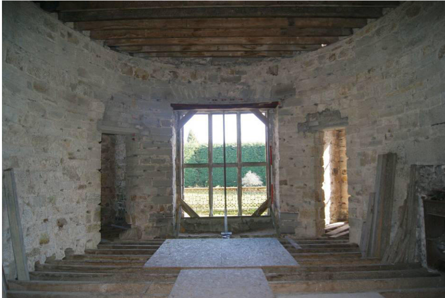
P113. R36 looking northwest to proposed site of a new doorway coming from R42. The wall is 1801-4 rubble masonry, stripped of lath and plaster. Replaced floor joists occupy the sockets
