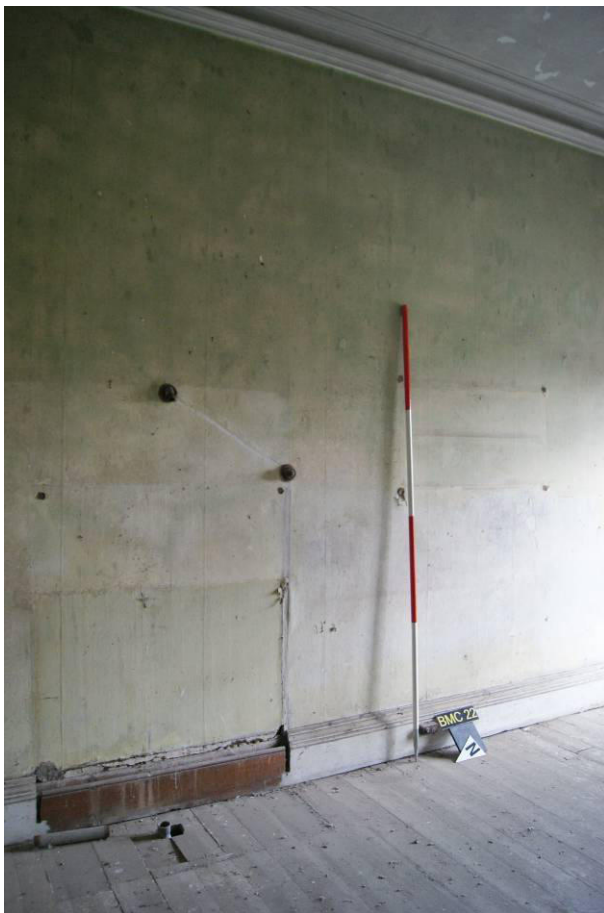
P141. R50. The section of east wall that is proposed to be opened out. The unpainted section of skirting marks the site of vanity unit.
