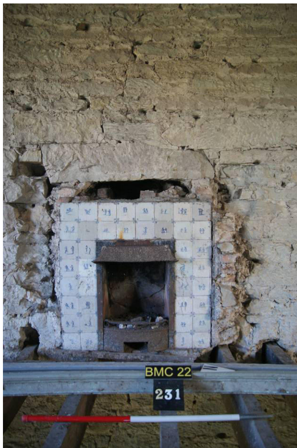
P155. R57. Tin-glazed 'Delft' tiling around fireplace [231], with detail of patterns (left) The surround is unlocated.
