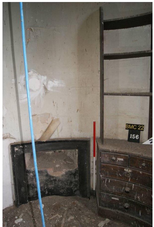
P117. R40 looking south-east to fire [259] which has been converted into a stove position (vent-pipe opening is infilled).
