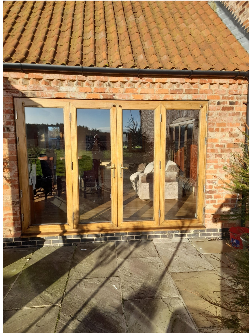
Figure 1—image showing materials, recycled brick, pantiles, limestone paving, window/door profile and colour of staining to wooden doors and windows
