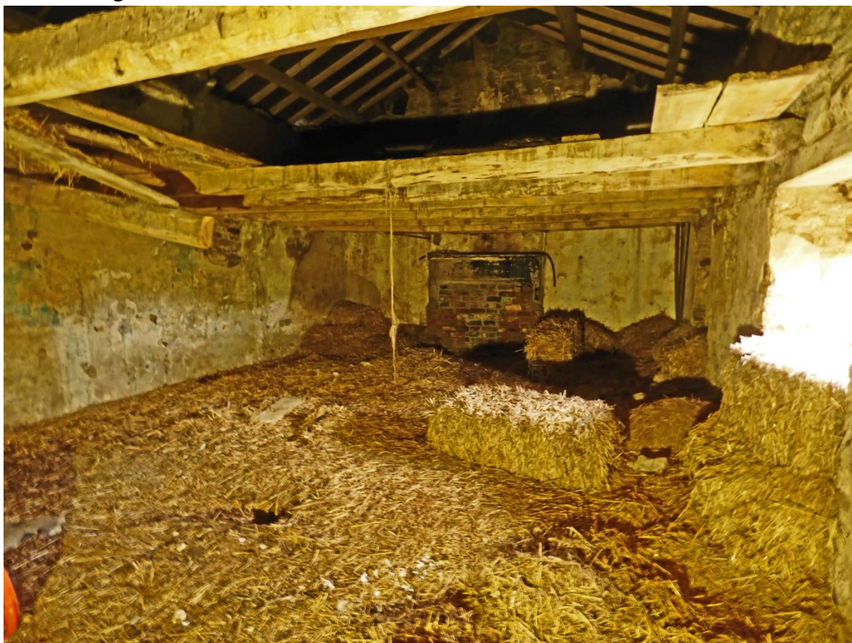
The Bastle-derivative House, first floor looking east
