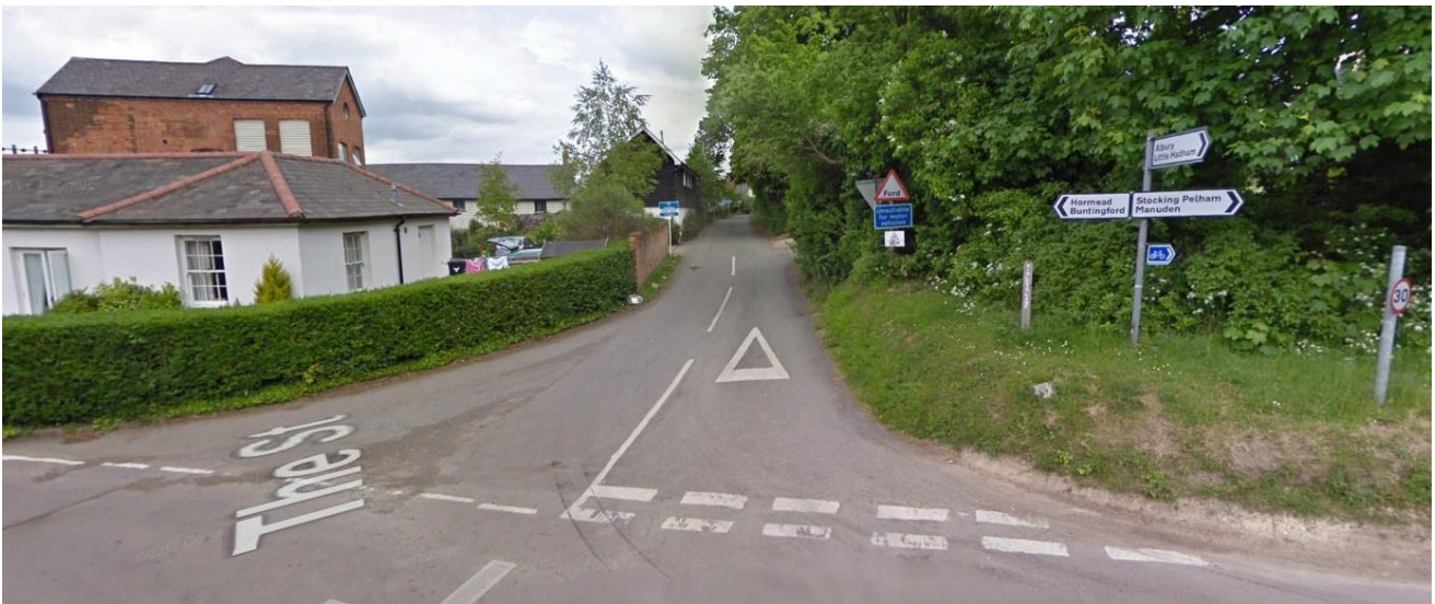
Fig. View on entering Violets Lane towards North View
