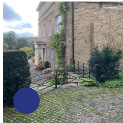
Existing Drive, Granite Cobblestones
