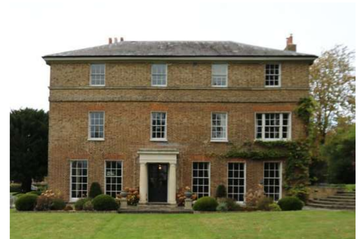
Site Photograph: Main House primary elevation.
