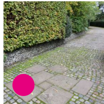
Existing Parking, Granite Cobblestone/ Sandstone Paving mix
