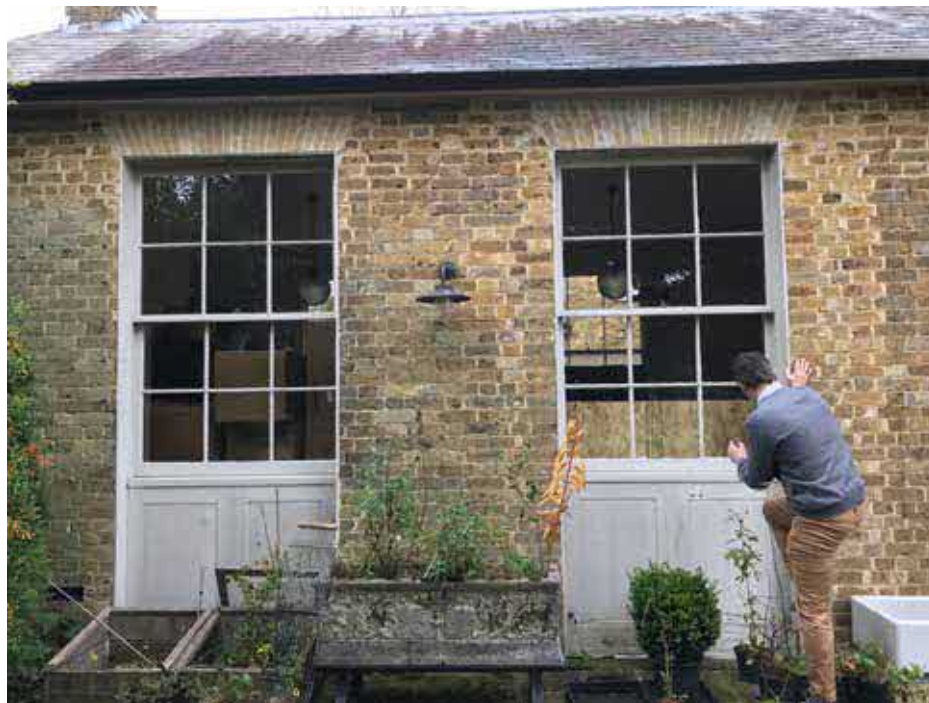
Figure 4.5 Photograph showing current arrangement. Source: Site visit.
