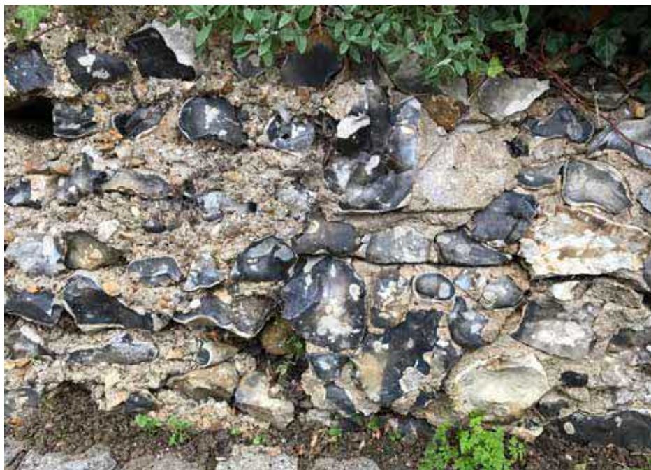
Figure 5.3 Photograph of a section of the flint wall to be relocated. Source: Photograph from site visit
