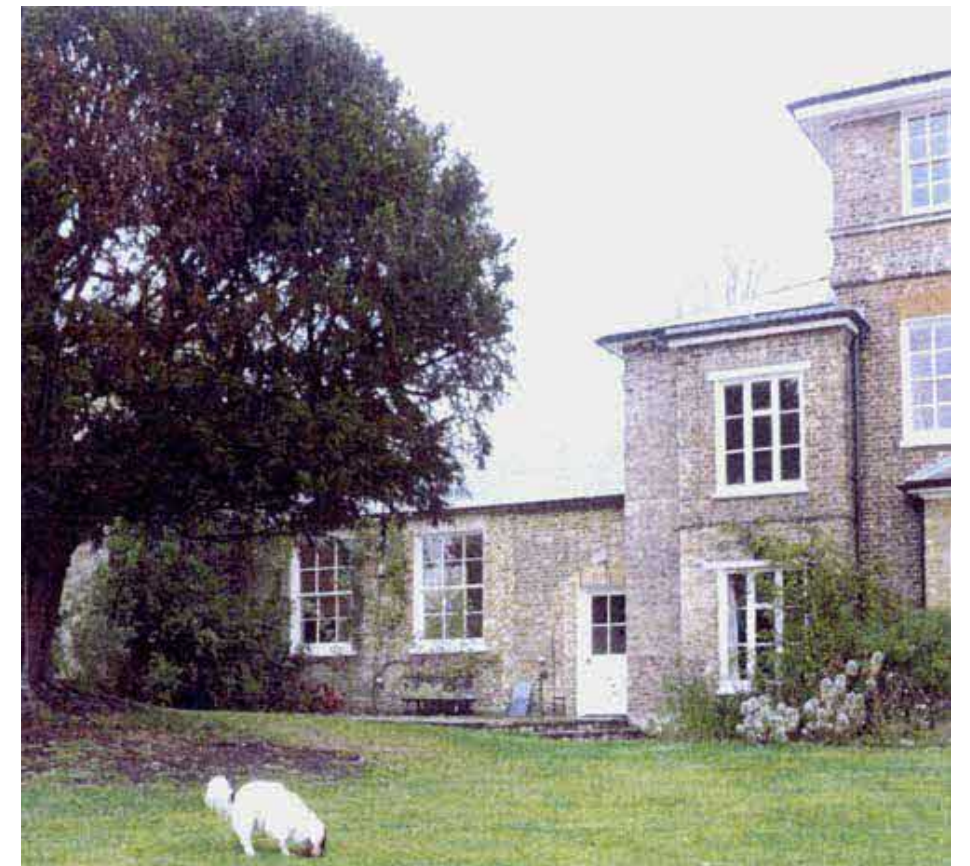
Figure 4.3 Photograph showing the two sash windows installed in 1990s. Source: Owners.
