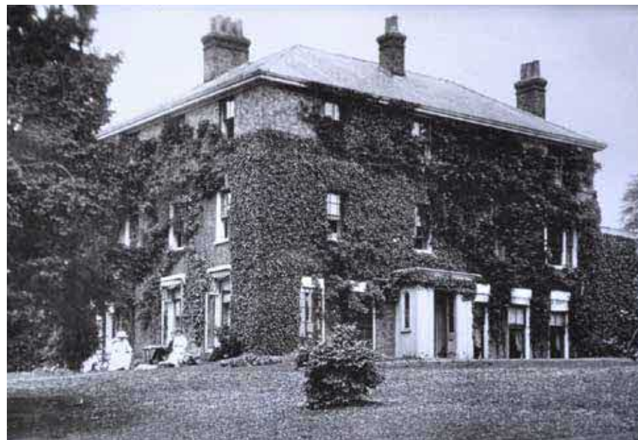
Figure 3.6 Little Munden Rectory c.1910, showing the south porch. This was mapped in 1880, and demolished c.1994. Source: Applicant.
