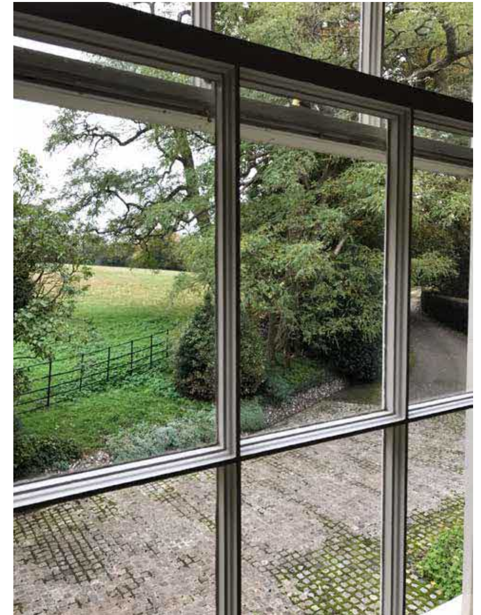
Figure 5.2 Photograph from the first floor showing proximity of the driveway to the house. Source: Site visit
