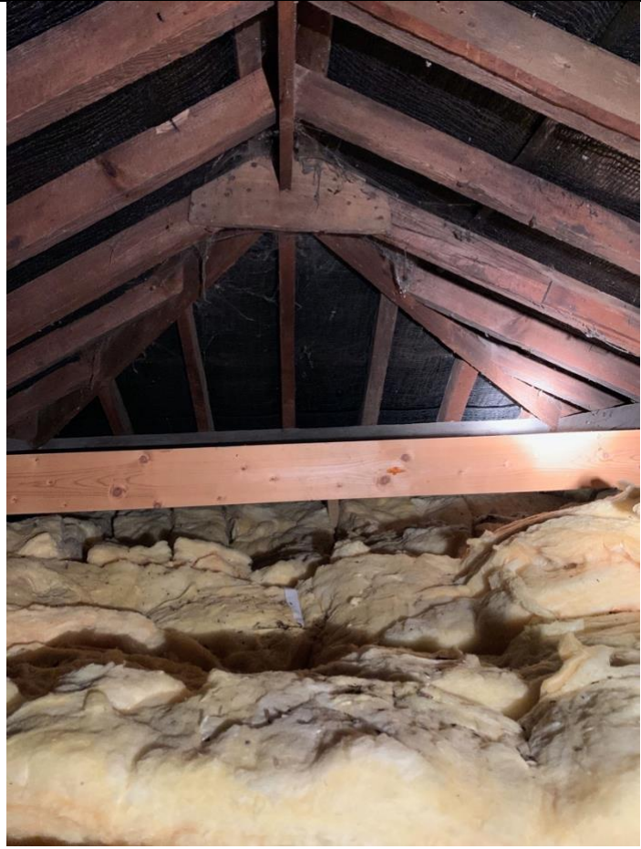
Photograph 3: Inside roof void 2.
