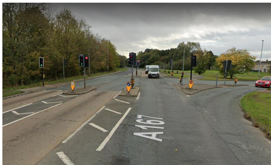
Image 3B-3 A167 / B6443 Traffic Signal Junction (taken October 2022)
