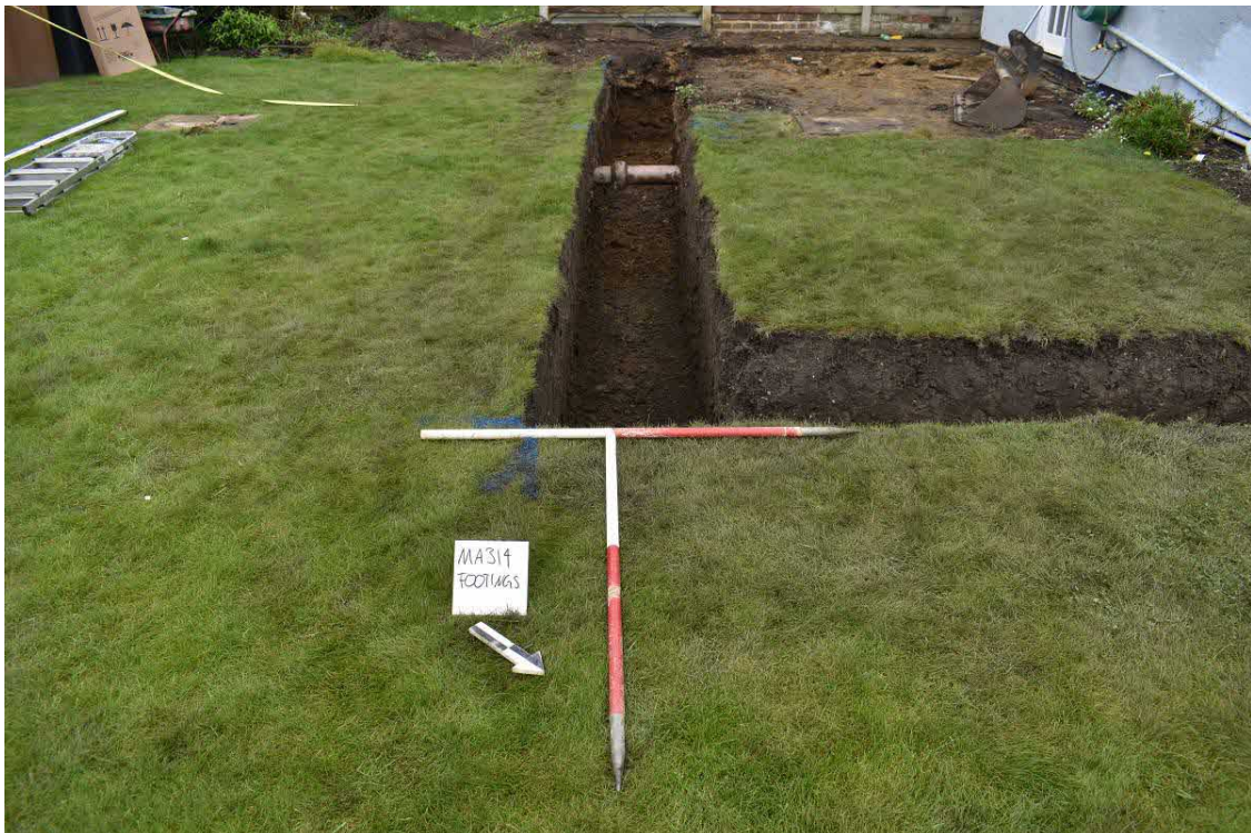
Plate 3: Footings of extension –Looking Southwest.
