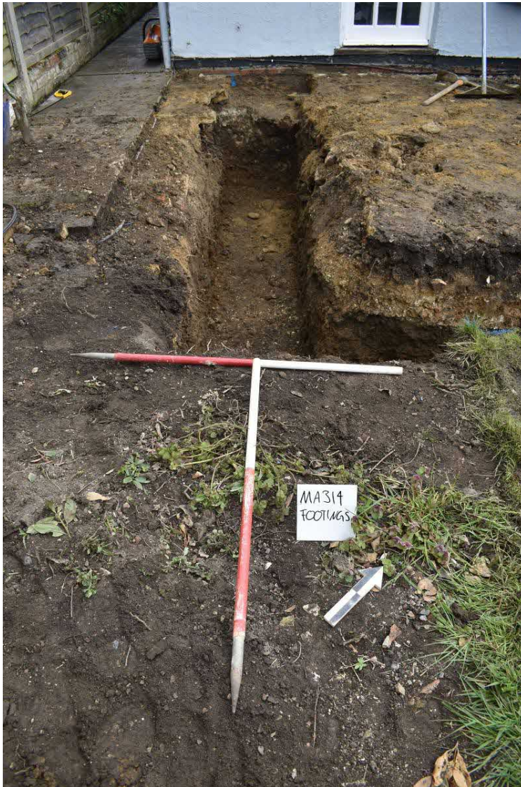
Plate 1: Footings of extension –Looking Northwest.
