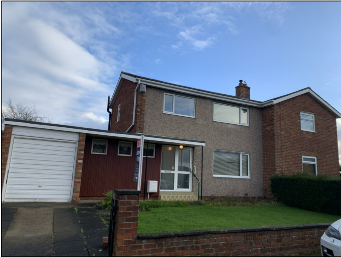
Photo 1 : Front elevation of property
