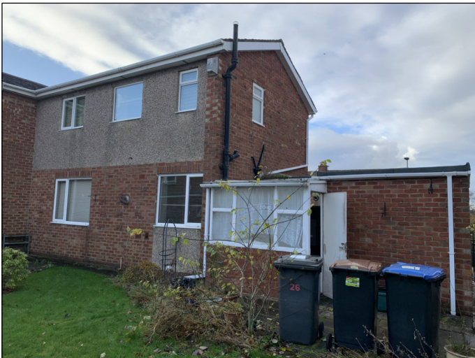
Photo 3 : Rear/gable of property
