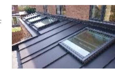
Typical Zinc Construction Pigments Blue, with ribbed roof upstand.
