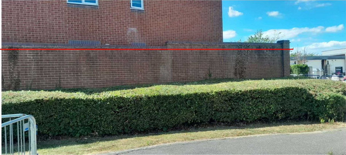
Side boundary wall
