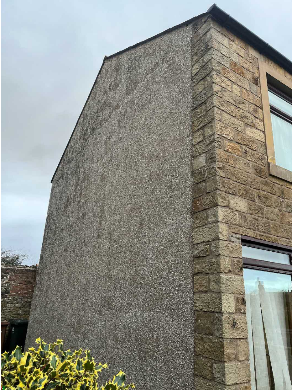
West side wall of existing house
