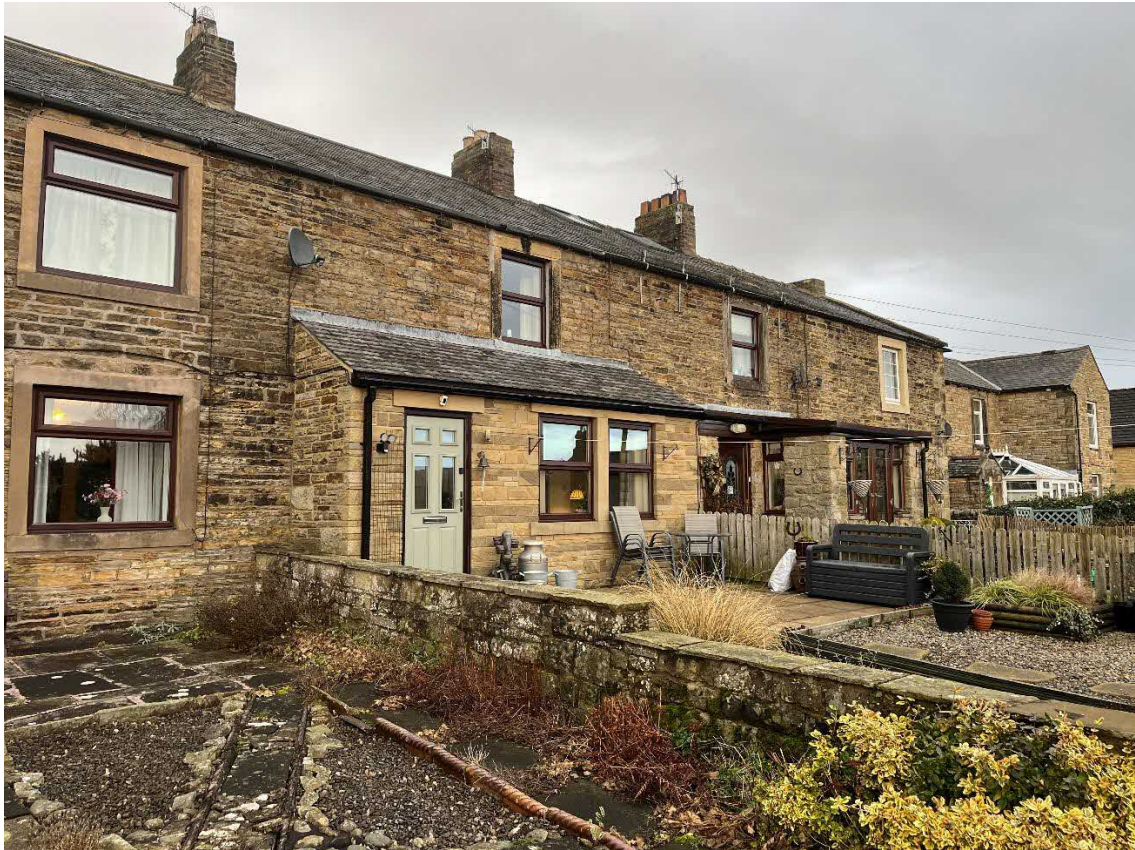
Adjacent properties – note forward extensions
