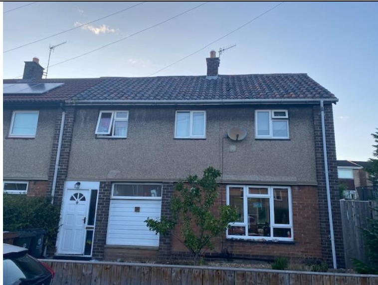
Photograph 2. Showing the front/ south eastern elevation of the property with UPVC doors and windows.
