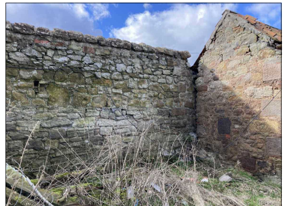
Existing stone wall, east side.
