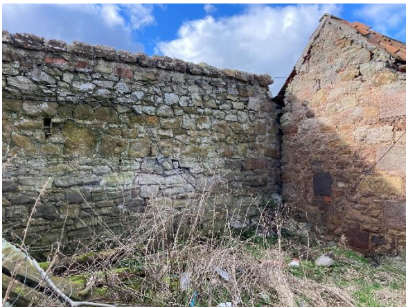
View from the east side.
