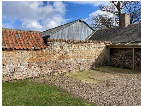
View from the west side.
