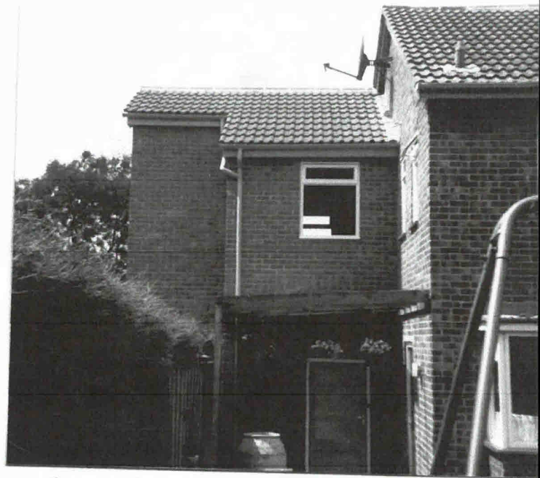
REAR PORCH BEFORE I PUT WOOD AND DOOR/WINDOW ON IT
