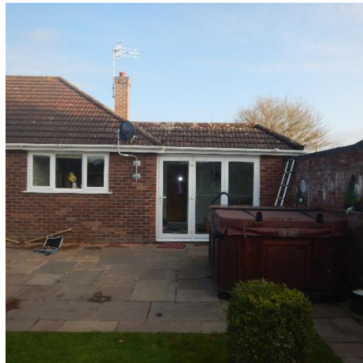
Existing rear and location of roof alterations
