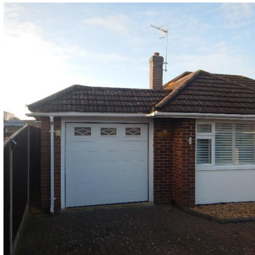
Existing front and location of roof alterations
