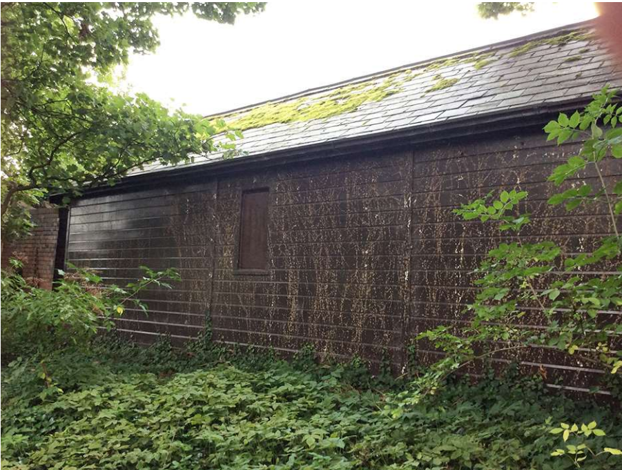
Figure 6: Platform 1 - View from North West
