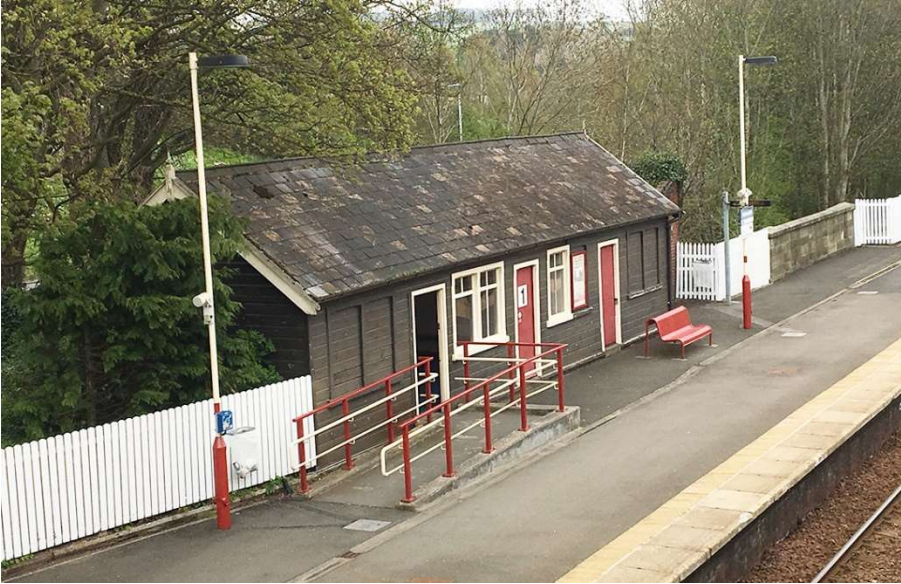
Figure 5: Platform 1 - View from South West
