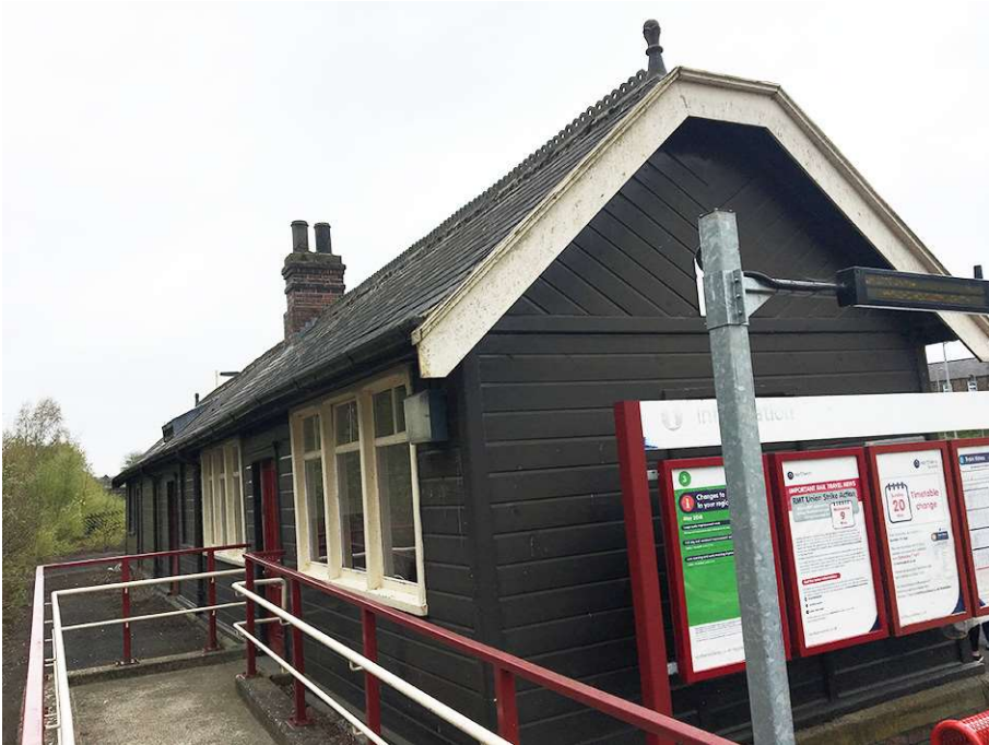
Figure 10: Platform 2 - View from South East
