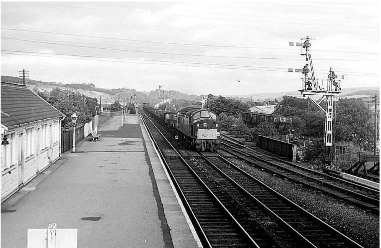
Figure 10: Platform 1 in the 1960's with the platform 1 waiting rooms on the left of the image
