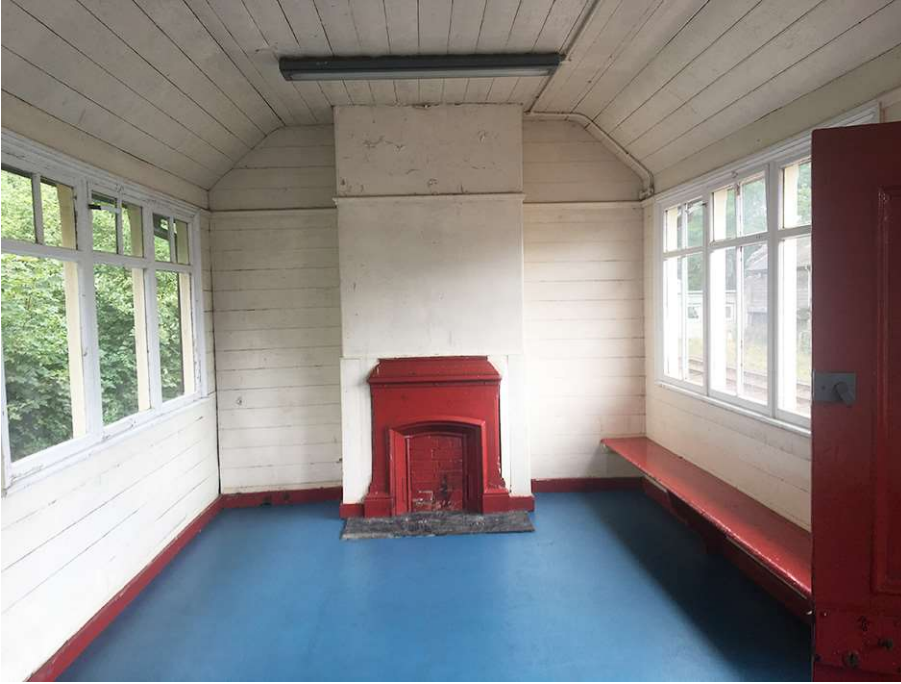
Figure 24: Platform 2 - Waiting room and fire place
