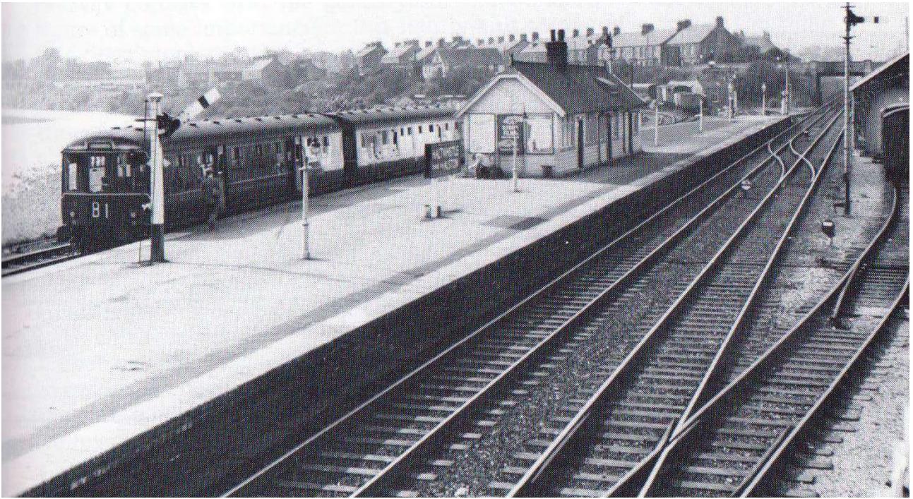
Figure 9: Platform 2 in 1963; Note the ventilation dormer on the North Side of the building above the toilets which have been roofed over.
