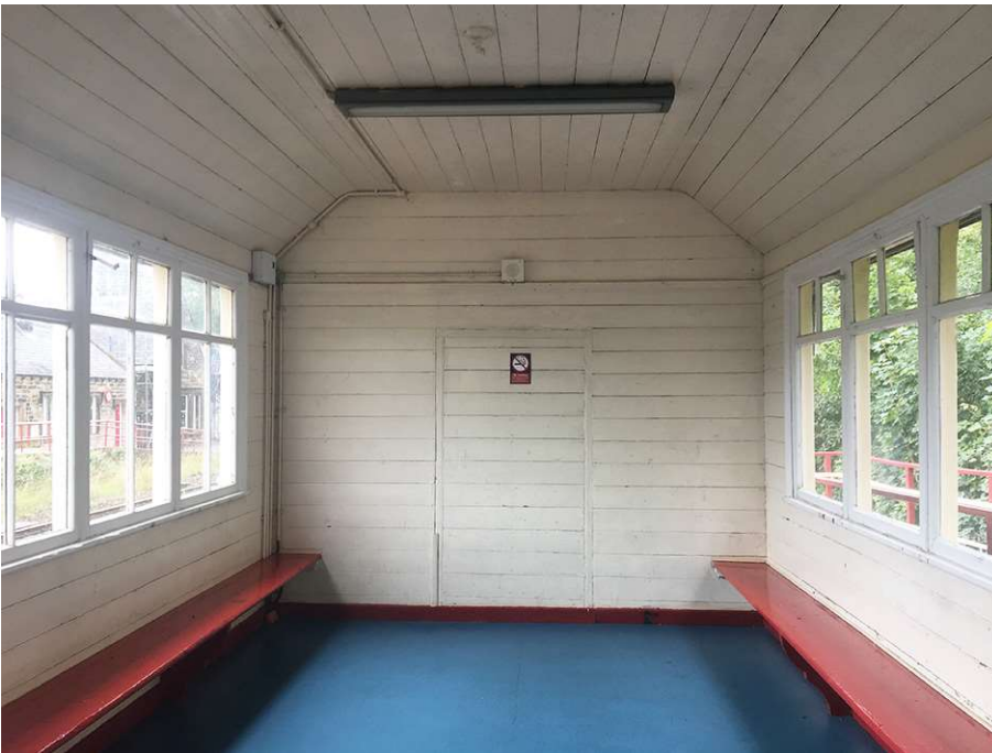
Figure 25: Platform 2 - Waiting room with blocked up door opening to East gable
