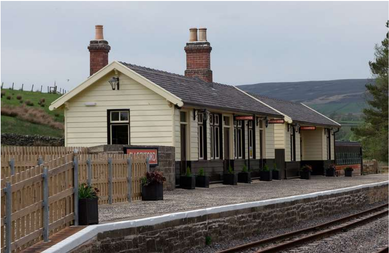
Figure 15: Slaggyford waiting rooms
