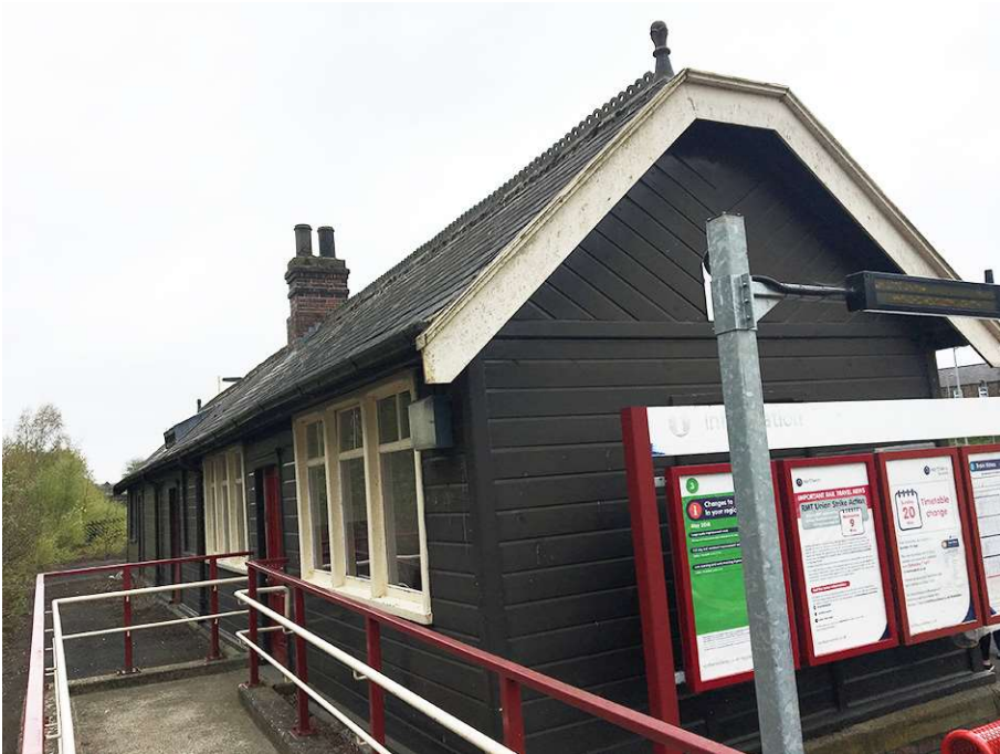
Figure 23: Platform 2 - View from South East
