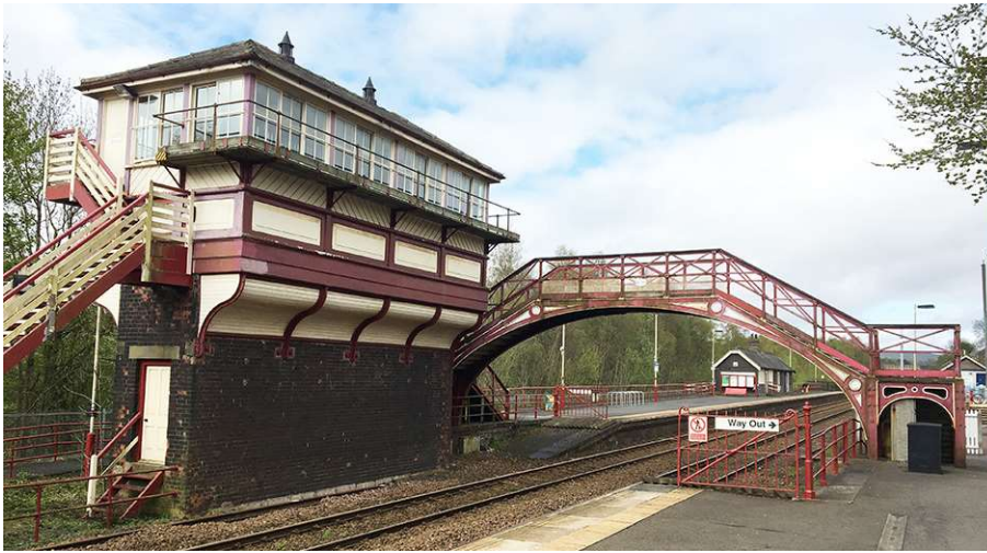
Figure 12: Haltwhistle Station - Footbridge and Signal Box
