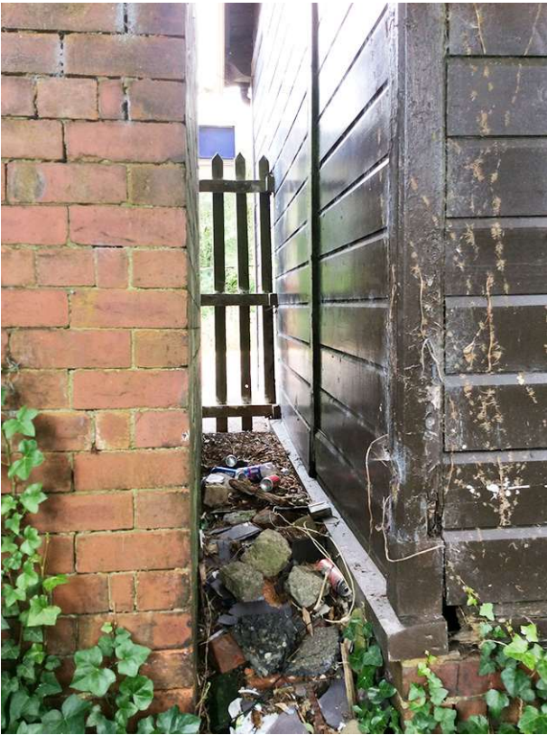
Figure 20: Platform 1 – North East and North West corners timber deterioration
