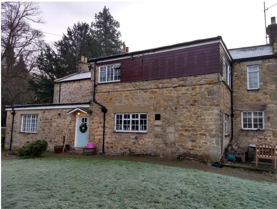
Existing rear (north) elevation in context (Elliott Architects)
