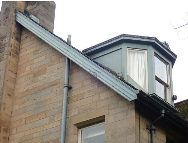
Barge boards to be replaced, northeast gable where bats emerged from beneath the slates
