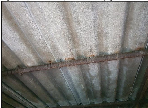
Figure 5: Unlined roof and metal frame
