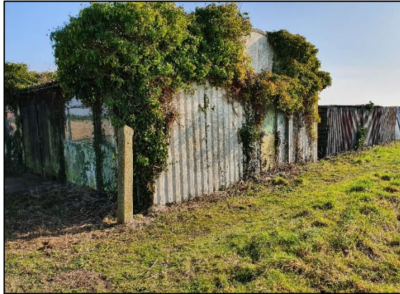
Figure 3: Western aspect – with ivy growth
