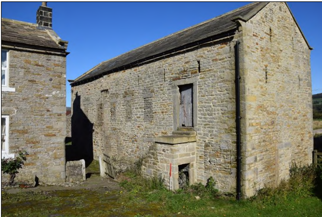
Photograph 4: Building 1. Note the placement of the blocked windows with reference to the floor height shown by the door. A dark line below the eaves, left of centre, is the iron strap that reinforces the junction between the older block and the extension at the far end
