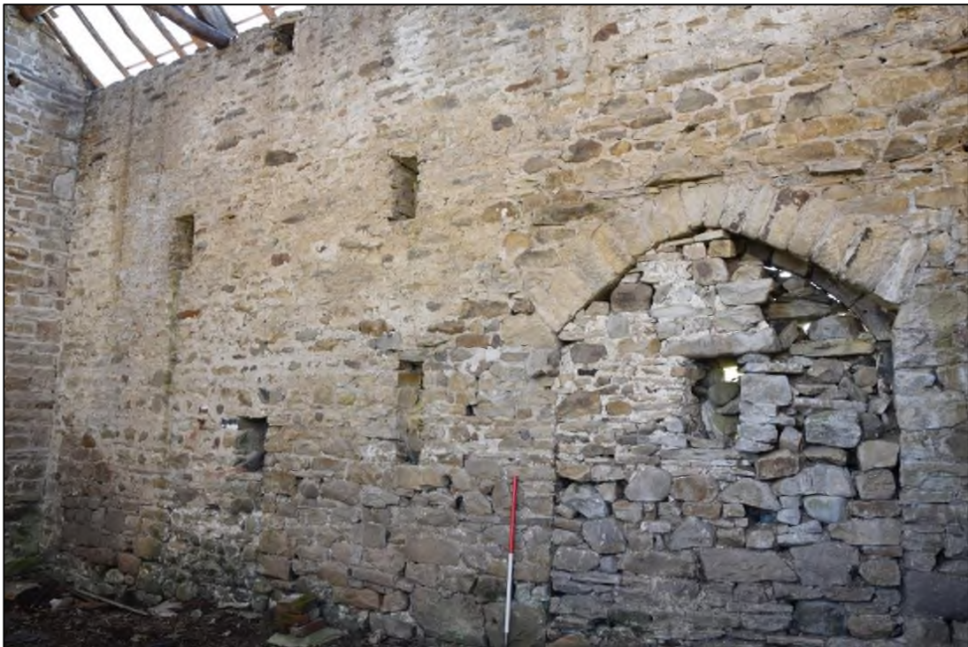
Photograph 40: The rebuilt south wall on the eastern part of the building. Note the change of masonry low down at the far corner
