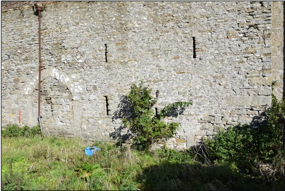
Photograph 35 (above): The wall at the east end of the south face is almost wholly rebuilt. The door jambs can be seen as in Photo 32
