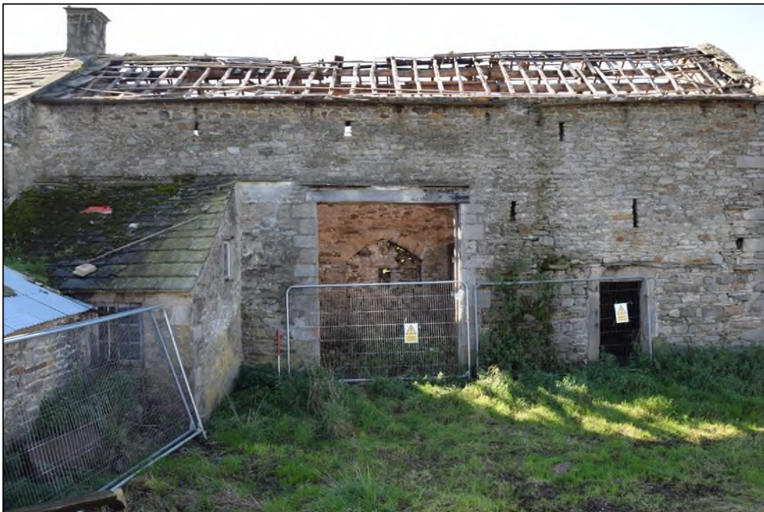
Photograph 28: The north face of building 2. Note the row of projecting throughs above the small door
