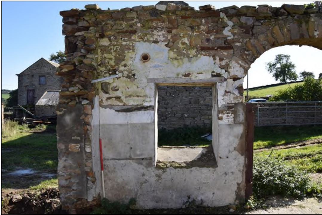
Photograph 57: The north-east corner has no sign of joists or sockets to correspond with those seen in Photo 56
