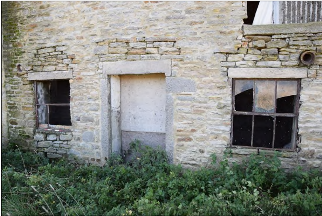
Photograph 13: The door and windows in the extension match those in the older block. The pipe is a ventilator for the cow byre
