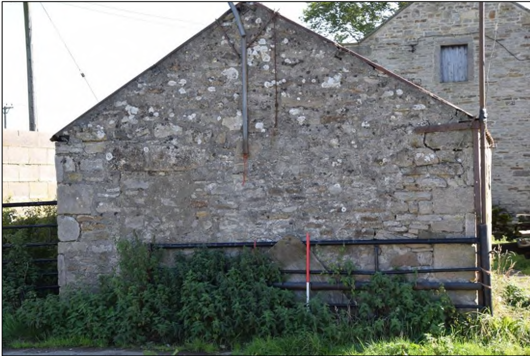
Photograph 65: The west end of the shed. A blocked door is faintly visible near the right-hand end
