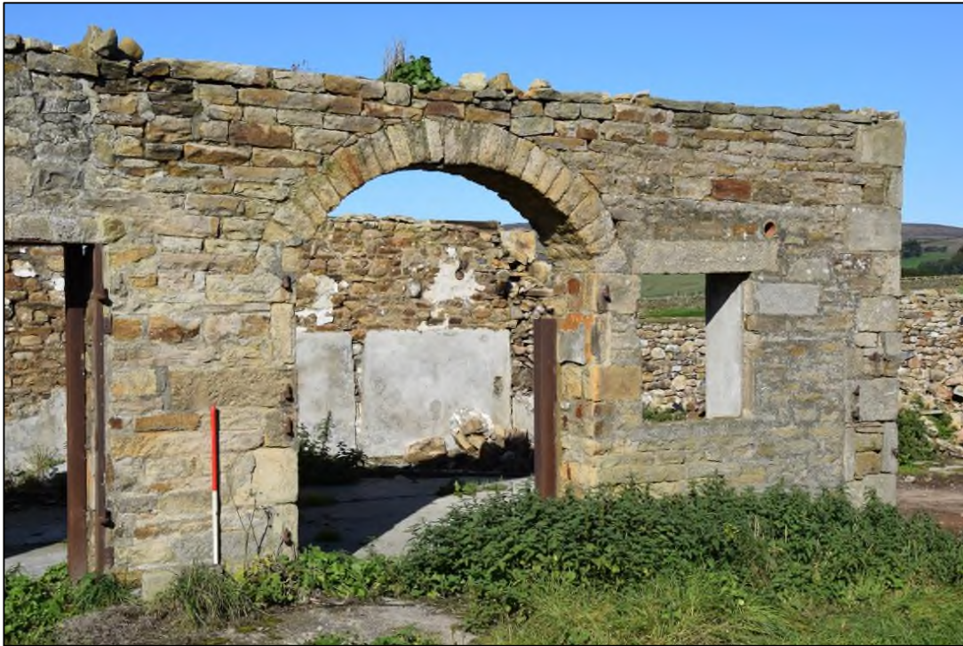
Photograph 49: The arched opening, superficially similar to a hemmel door, is a later addition to the building
