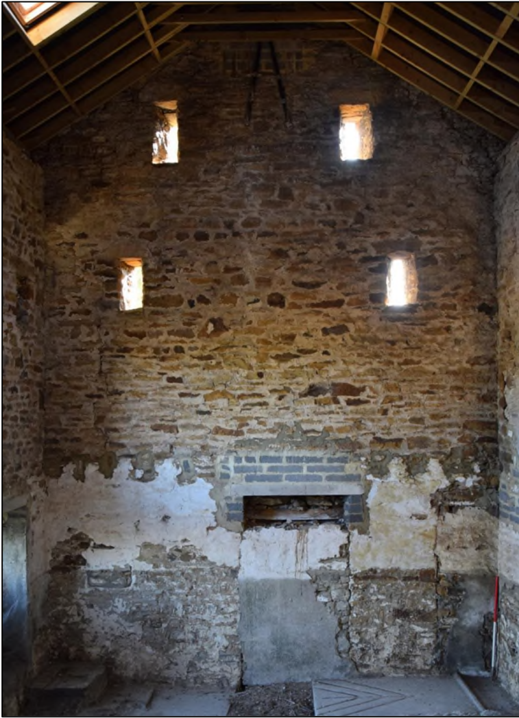
Photograph 17 (left): The east end of building 1, showing the wall finishes restricted to the byre. There is no sign of a loft; the roof is new
