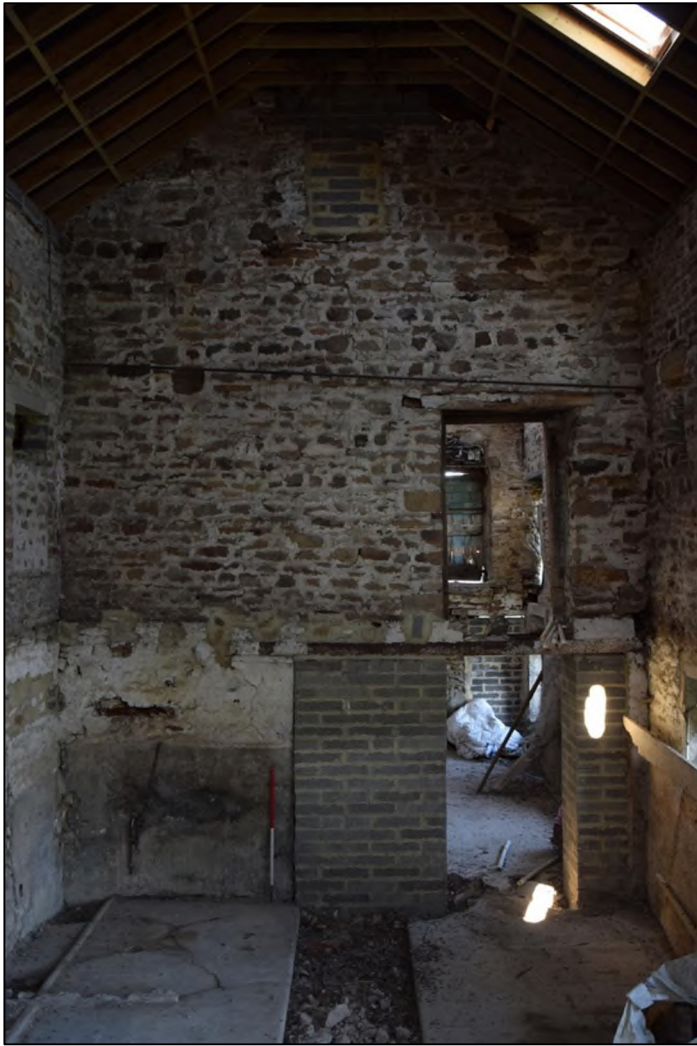
Photograph 19 (left): The old west end, now an internal wall, has been rebuilt at the base. The open door above would have been used for loading hay
