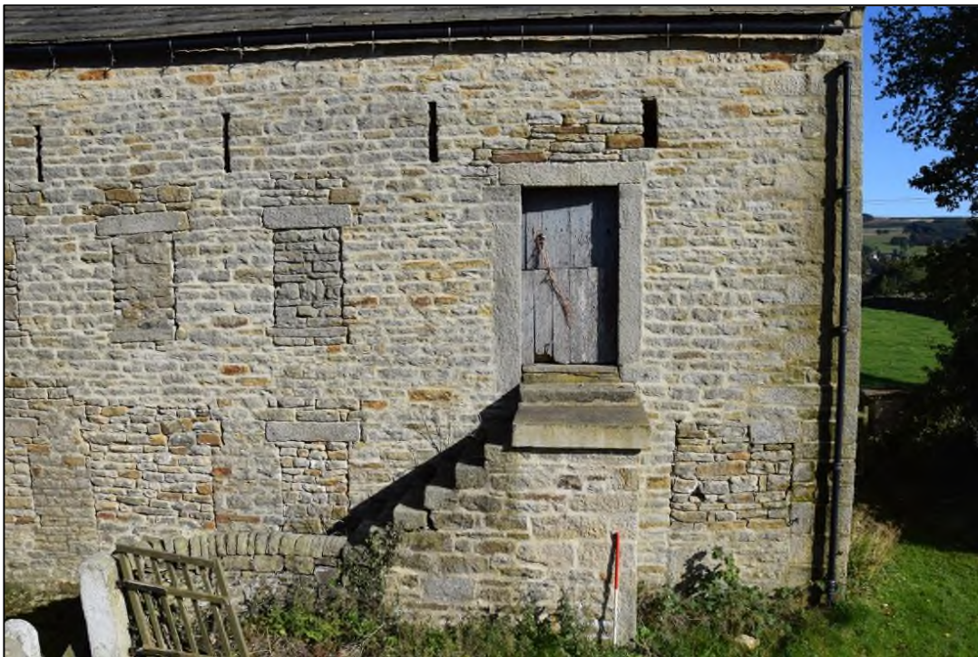
Photograph 6: The hay loft entrance near the south-east corner of building 1. Blocked doors can be seen to the right of the staircase and above the wooden gate
