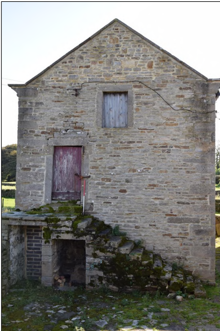
Photograph 7 (above): The west extension of building 1. A small step in the face, below the eaves at the right, marks the end of the older part. Compare the quoins here with those in Photo 5
