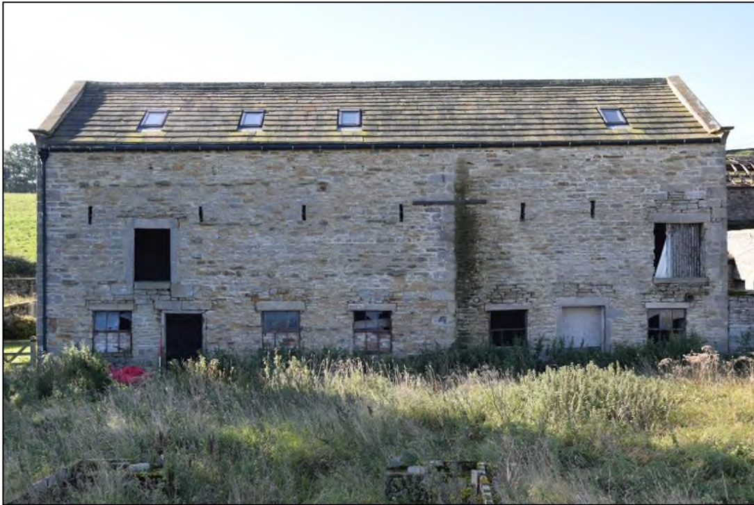
Photograph 9: The division between the two parts of building 1 is very clear in this view of the north face. The open stonework above the openings is the result of repair of the door and window lintels
