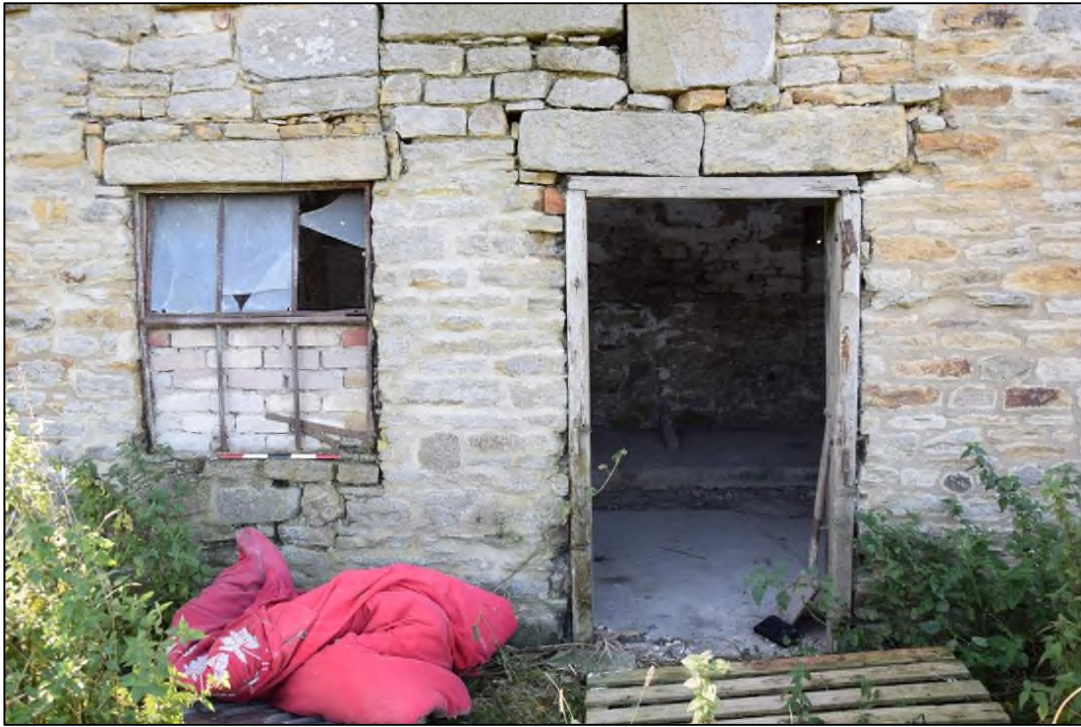
Photograph 11: Detail of the door and window at the east end of the north face. The loading door above has been altered
