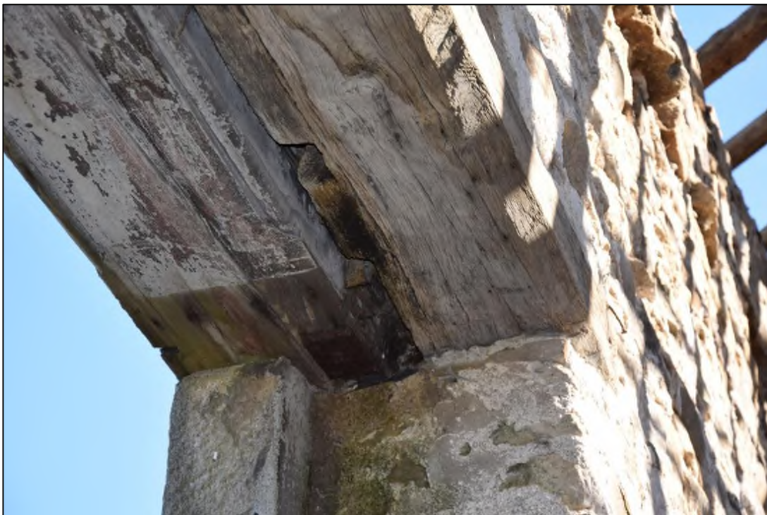
Photograph 46: Re-used timber in the lintel of the 20th-century door on the north side of building 2
