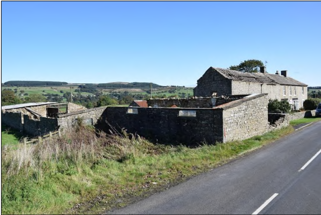
Photograph 3: The site from the south-west, with the truncated building 4 in the foreground
