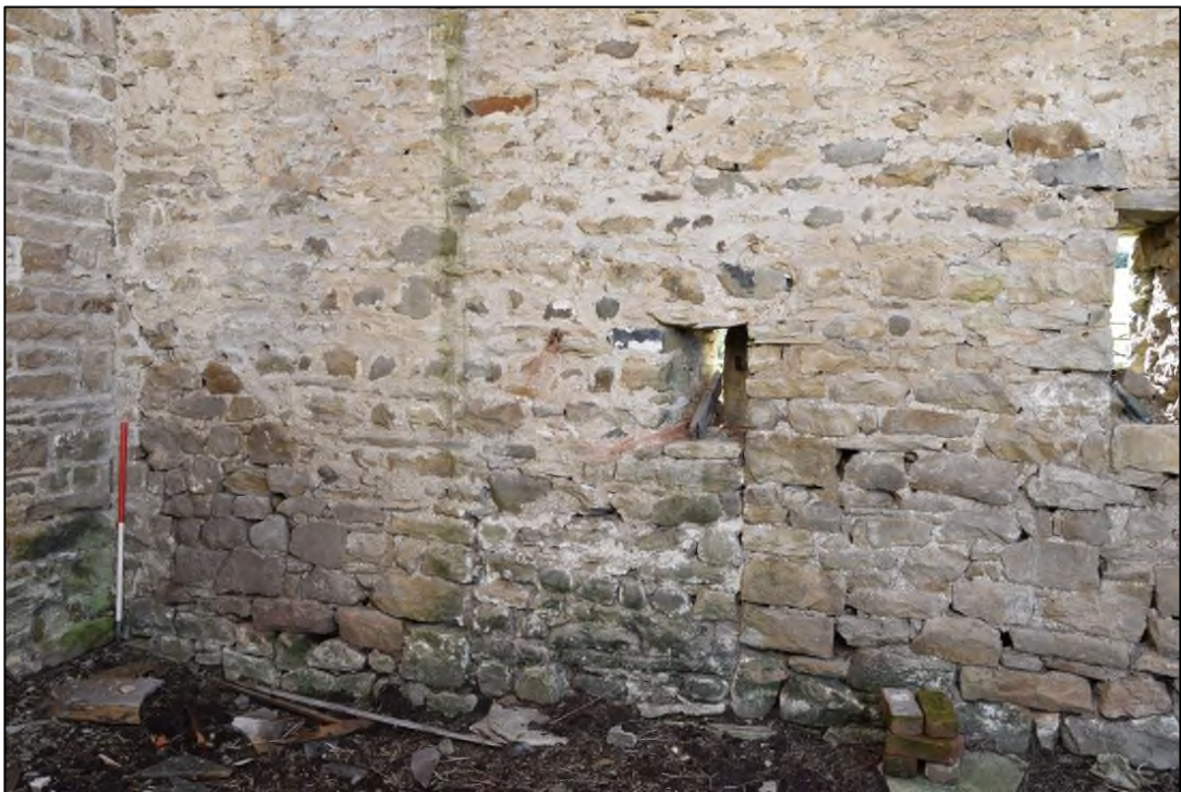
Photograph 42: The truncated blocked door at the south-east corner. The jamb can be seen in the low breather slit. Older masonry survives low down, beside the scale
