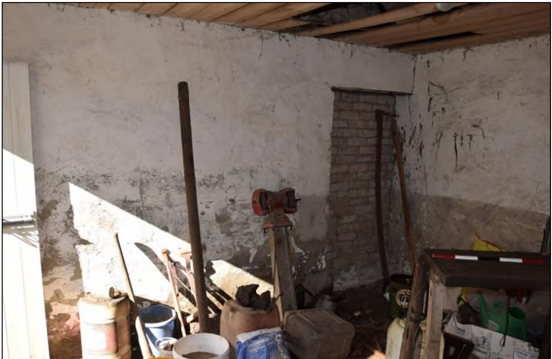
Photograph 68: A view looking north-west in the east room, with the blocked internal door
