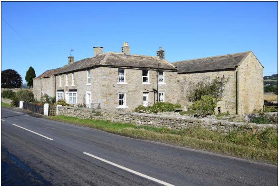
Photograph 2: The L-shaped houses at the east side of the site. Building 1 is at the right and building 2 continues the range at the left
