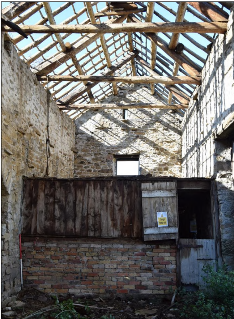
Photograph 35 (above): The wall at the east end of the south face is almost wholly rebuilt. The door jambs can be seen as in Photo 32
