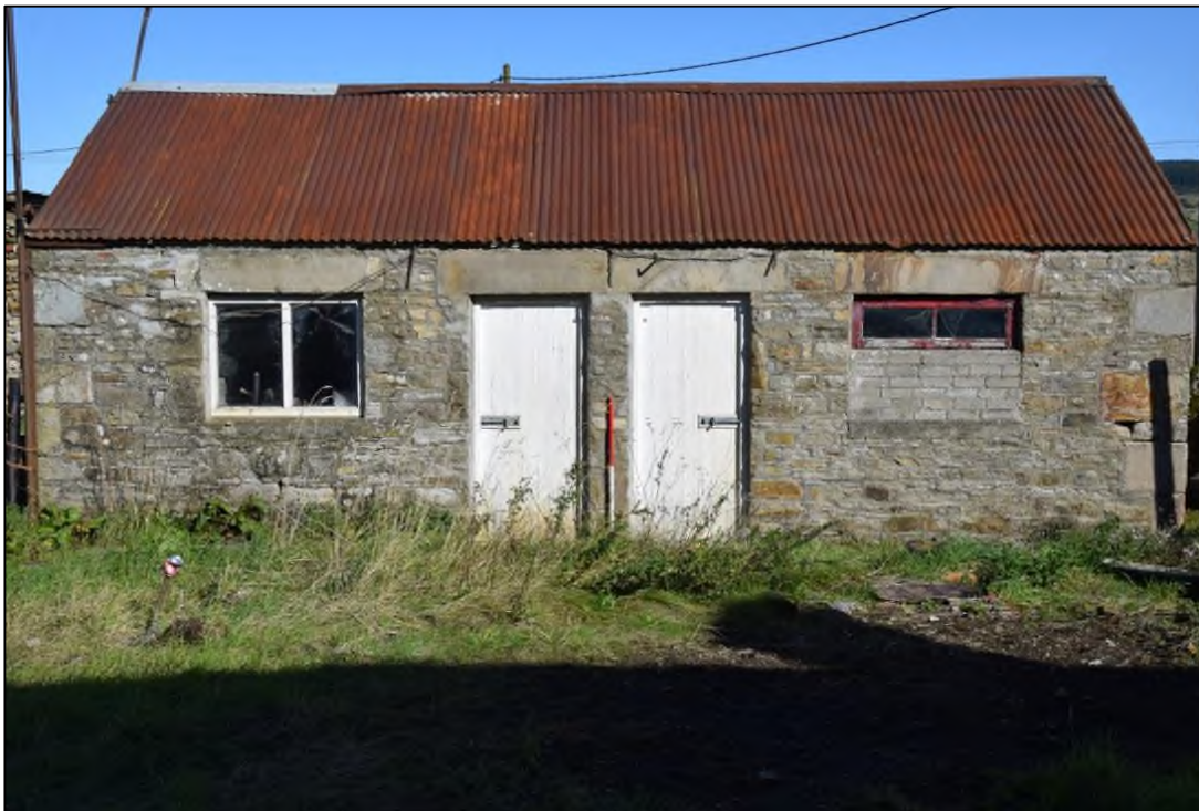
Photograph 64: The south face of building 5
