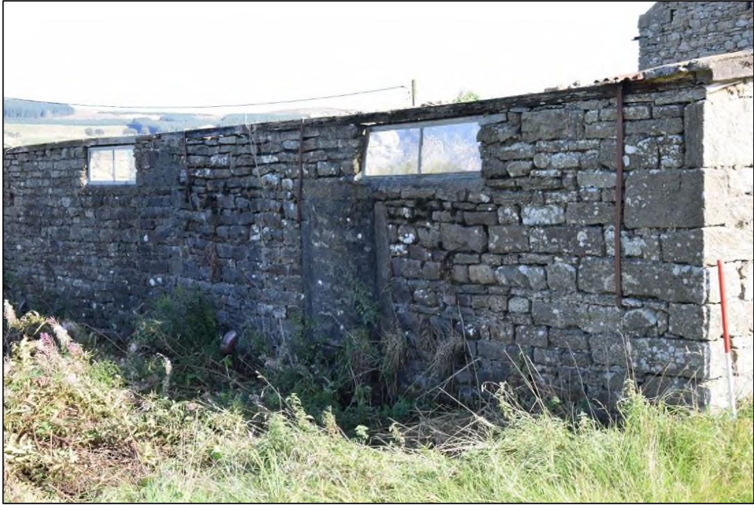
Photograph 51: The west face of building 4, with recent high windows above a blocked door
