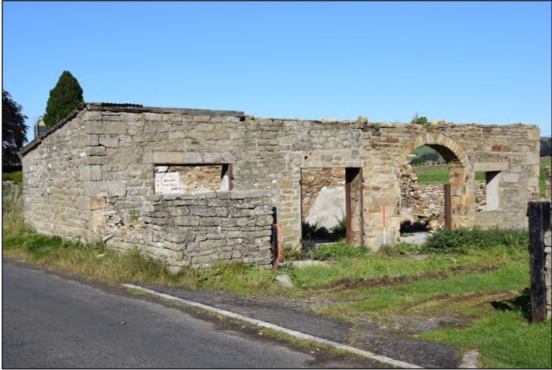
Photograph 47: Building 4 seen from the south-east
