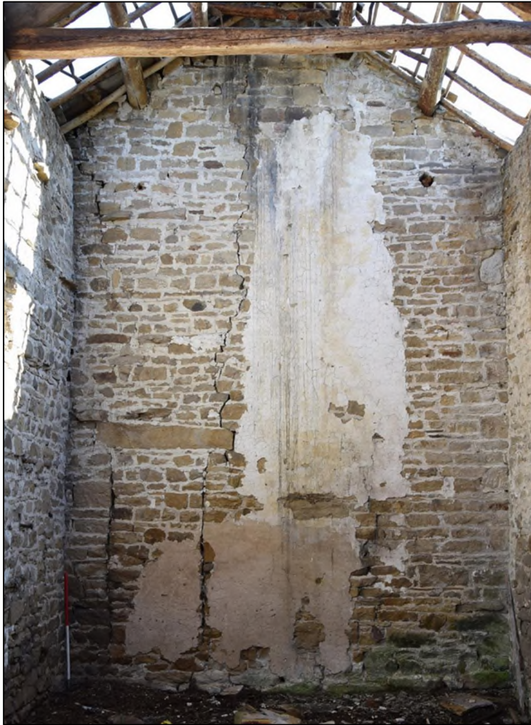
Photograph 43 (left): The east end of building 2 has a door into the adjoining house
