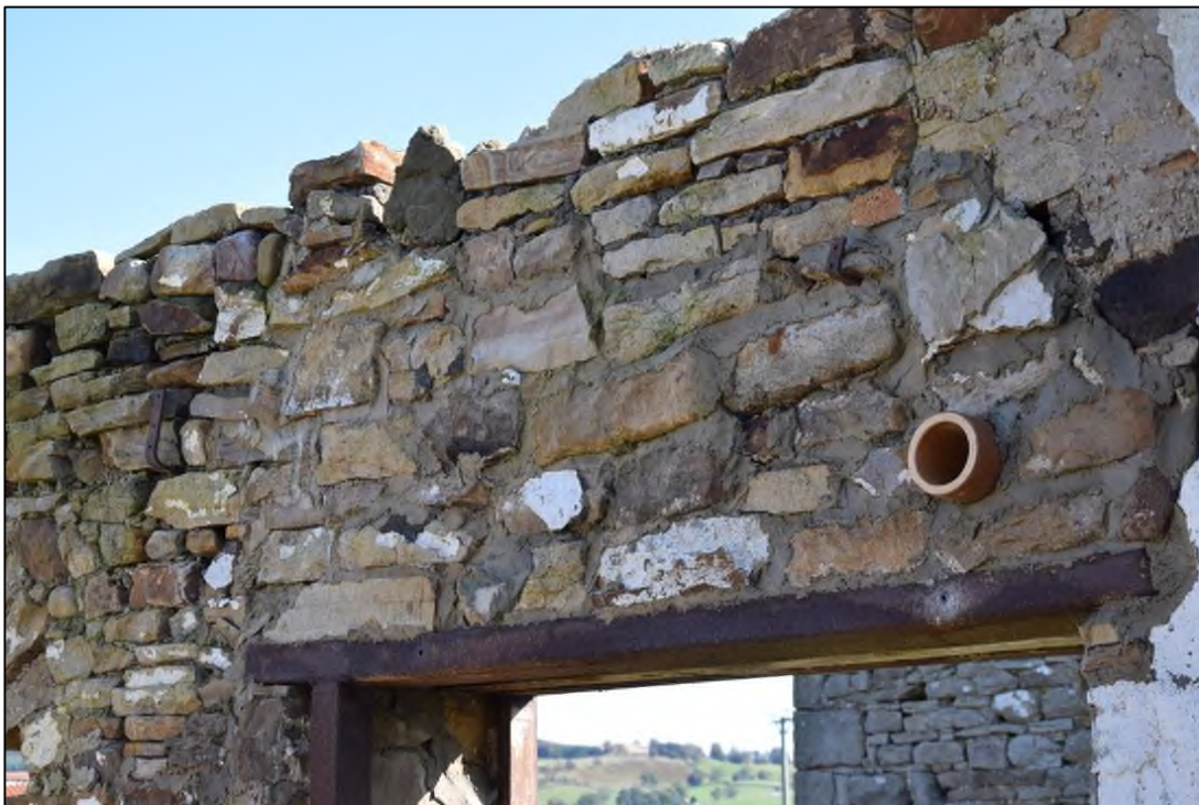
Photograph 60: The same pattern is seen over the middle door of building 4
