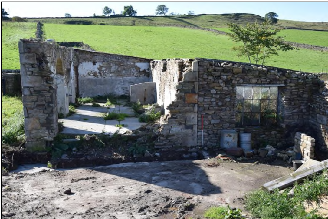
Photograph 50: Most of the north end of the building has been demolished. The wall with the window is what remains of an adjoining single-storey building
