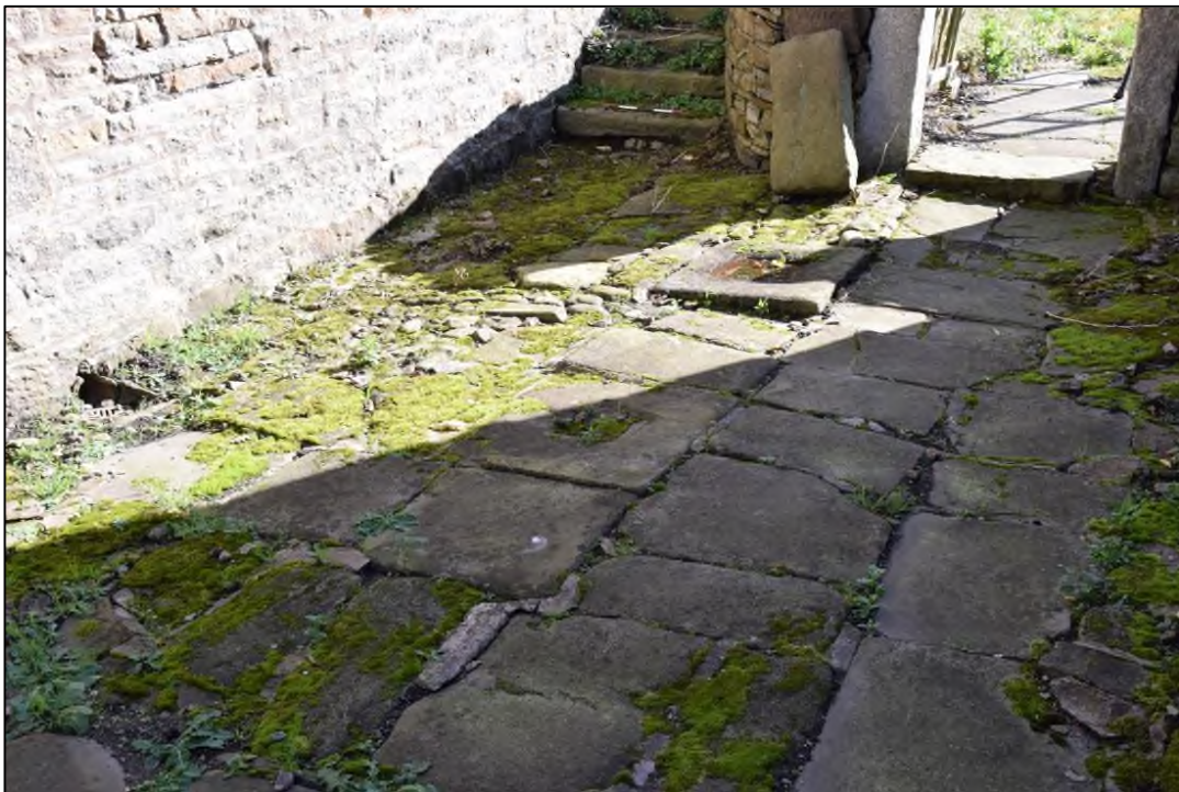
Photograph 14: The paved yard between building 1 and the eastern house has two recesses for uprights outside the old door, the blocking of which can be seen at the top left
