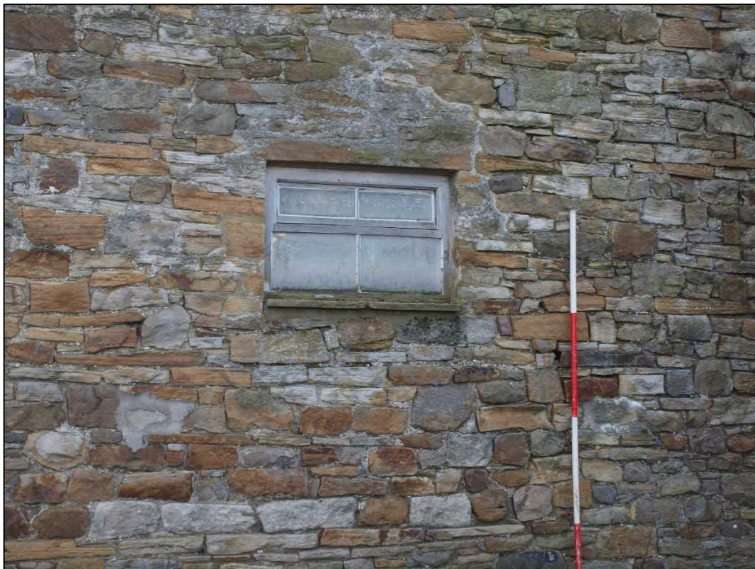
Plate 28: Ground floor window to bay 3 looking south
