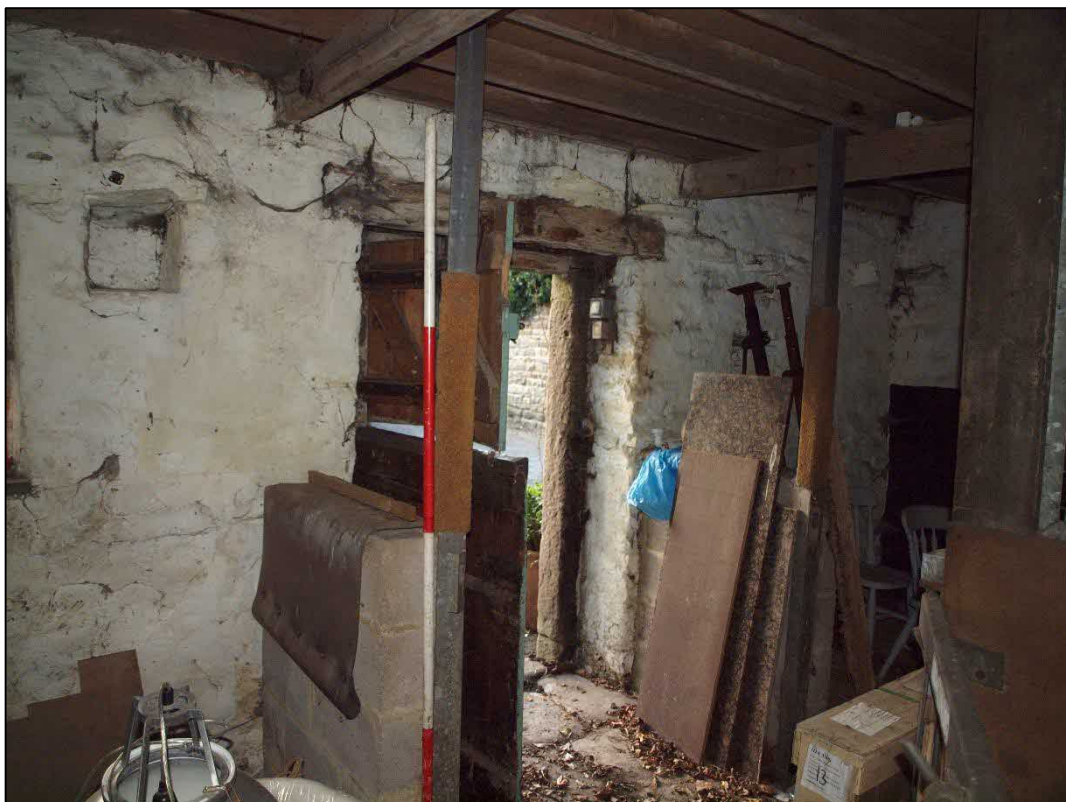
Plate 44: Doorway with niche in wall to the east looking southwest
