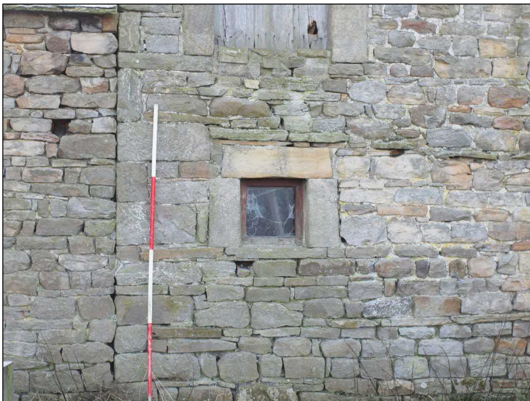
Plate 24: Ground floor window to bay 10 looking south
