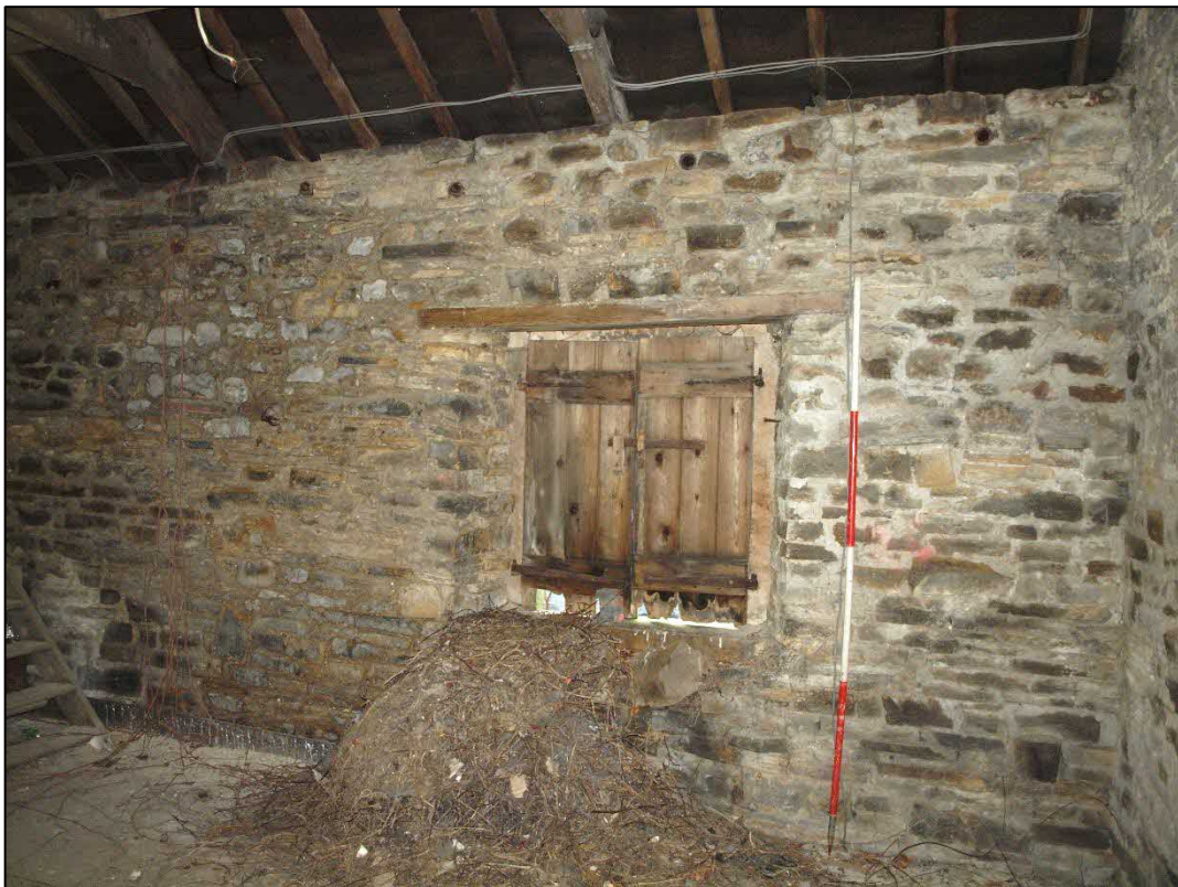
Plate 62: Pitching eye to south elevation looking south
