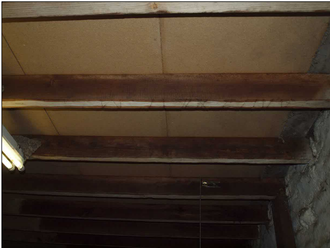
Plate 47: Modern ceiling looking south
