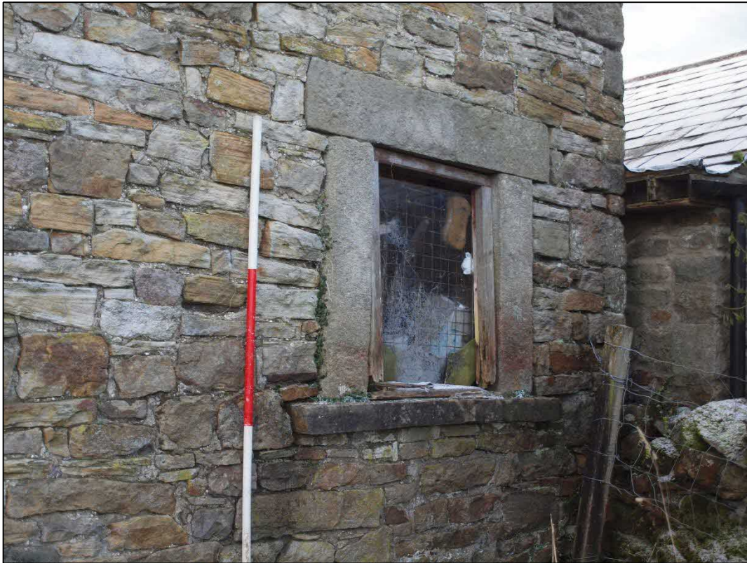
Plate 29: Window to bay 1 looking southwest
