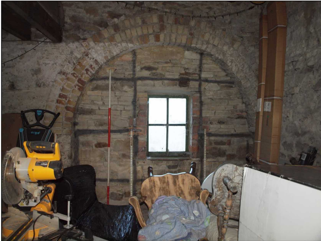
Plate 37: Blocked barn door in north wall looking north
