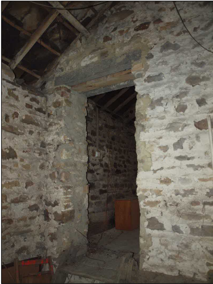
Plate 53: Detail of inserted doorway looking southwest
