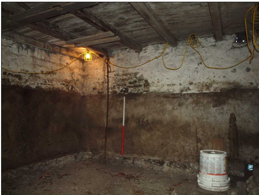
Plate 48: Interior of eastern gable extension looking northwest
