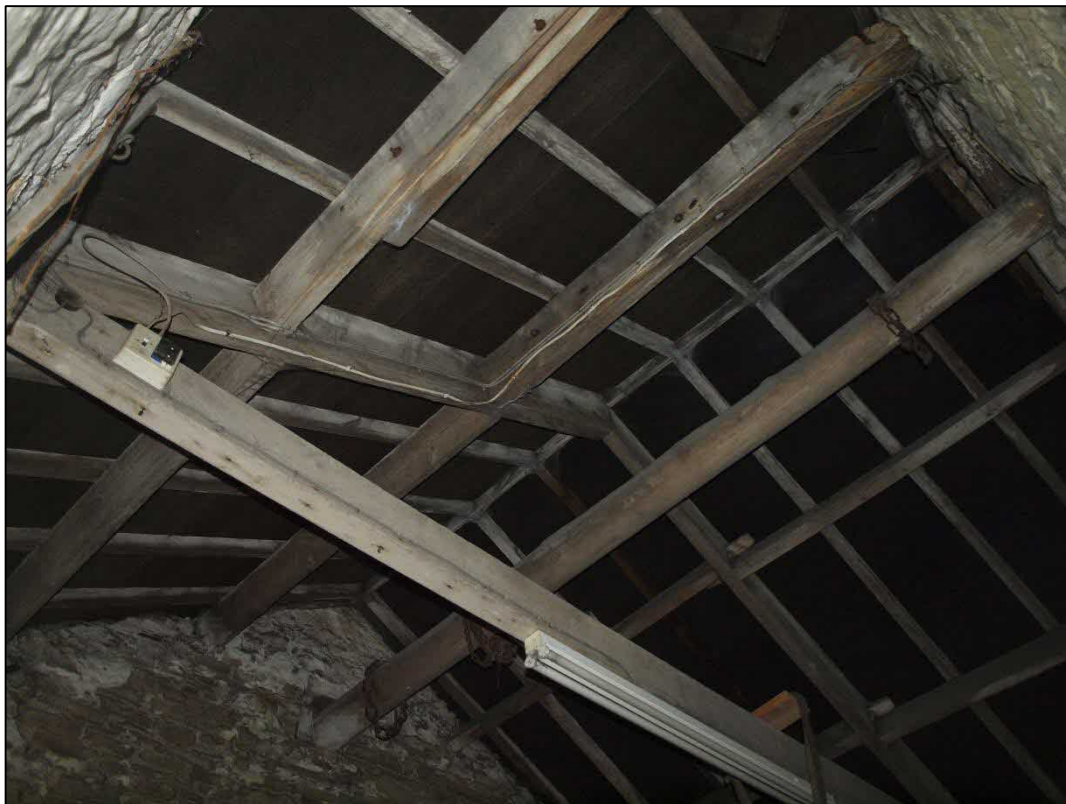
Plate 32: Details of roof structure looking northwest
