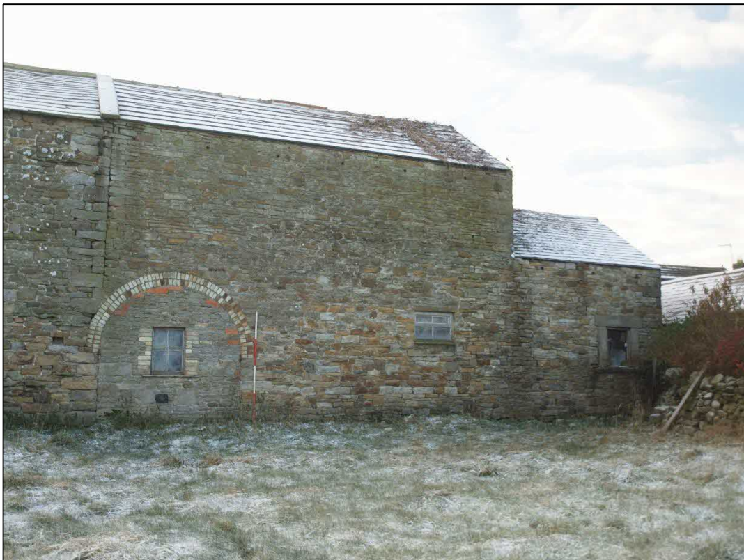
Plate 26: West end of elevation, bays 1 - 5 looking southwest
