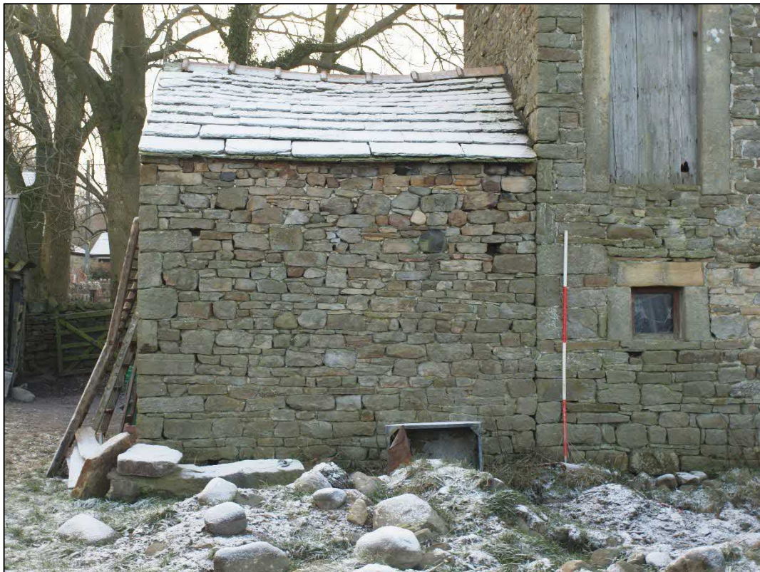
Plate 23: North elevation of eastern extension looking south
