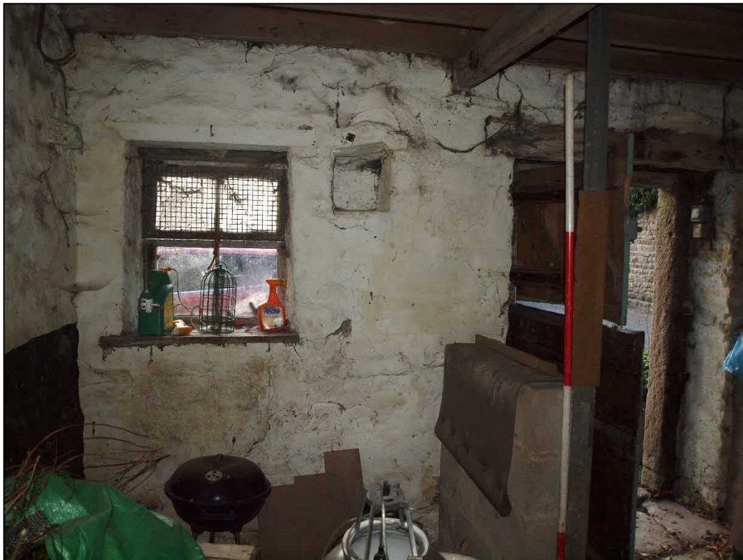
Plate 43: Southern wall showing window and doorway
