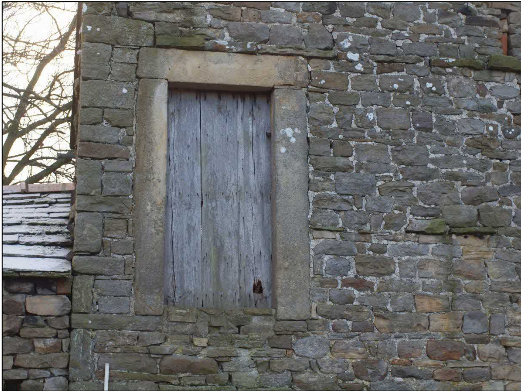
Plate 25: First floor doorway to bay 10 looking south
