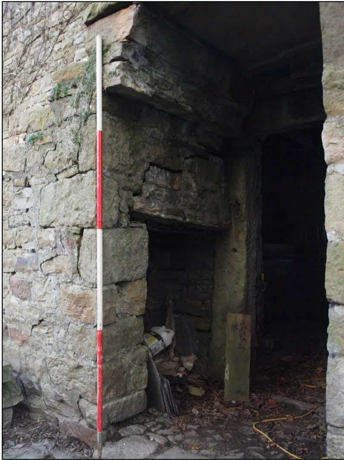
Plate 15: Ground floor doorway to bay 10 below stairs looking northwest
