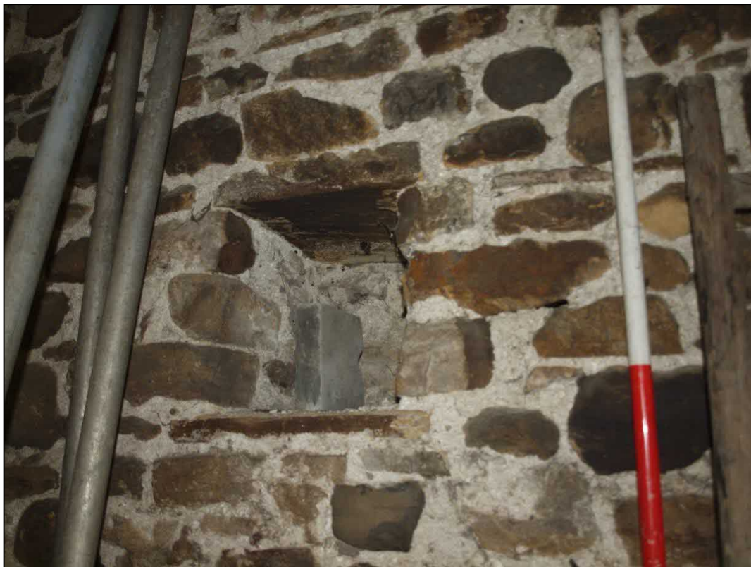
Plate 58: Niche in east wall looking east
