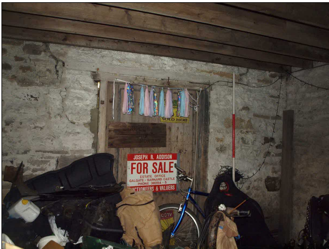
Plate 36: Doorway to bay 3 in west wall looking northwest
