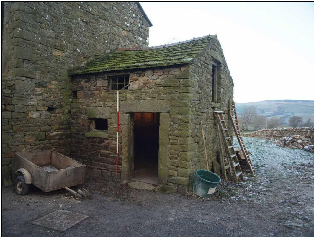
Plate 17: Bay 11 extension looking northwest
