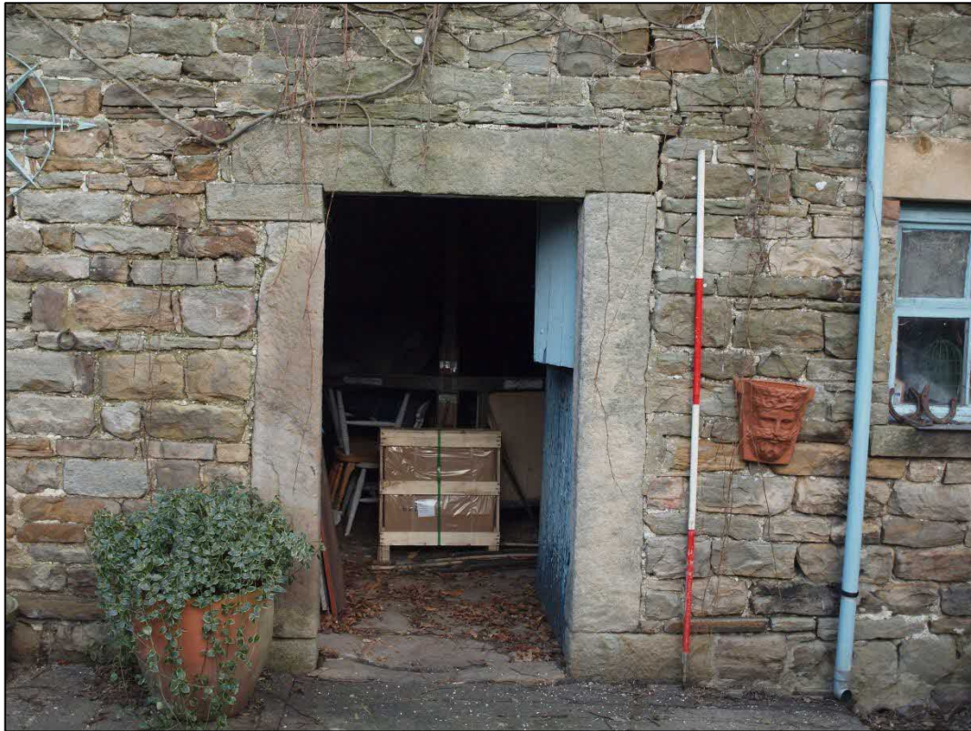
Plate 11: Doorway to bay 7 looking north
