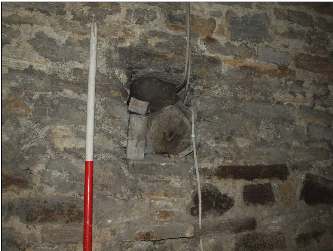
Plate 60: Ventilation slot in west gable
