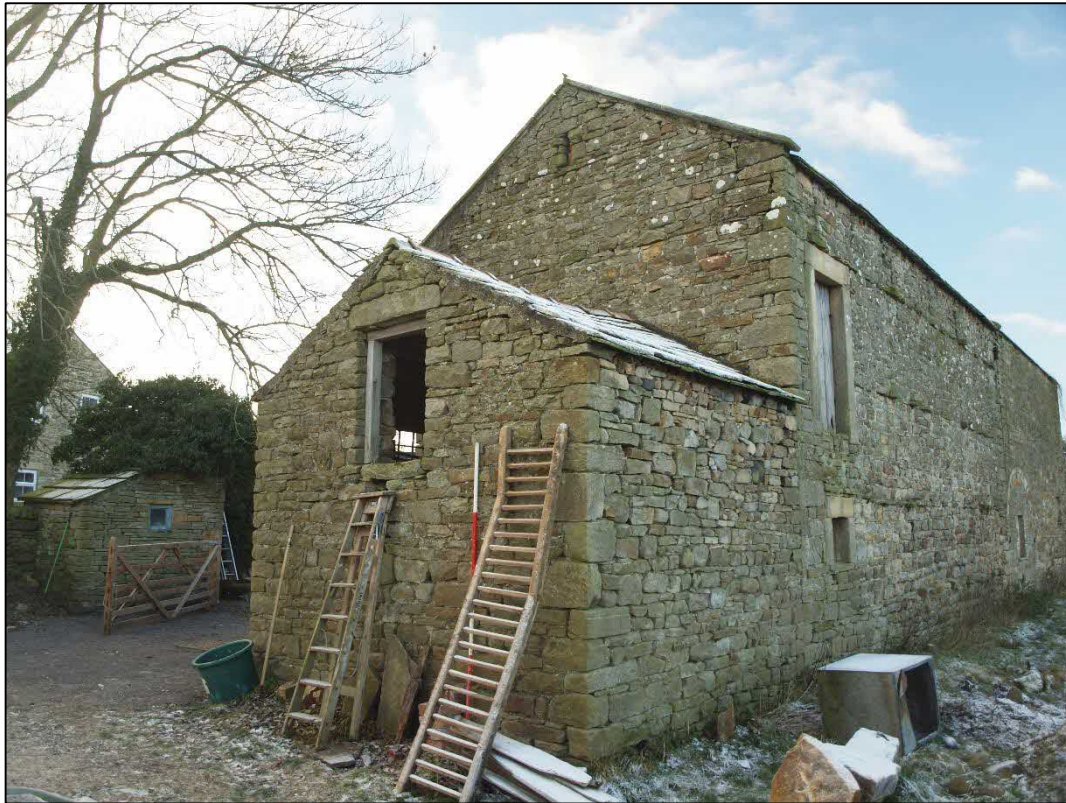
Plate 21: East gable looking west
