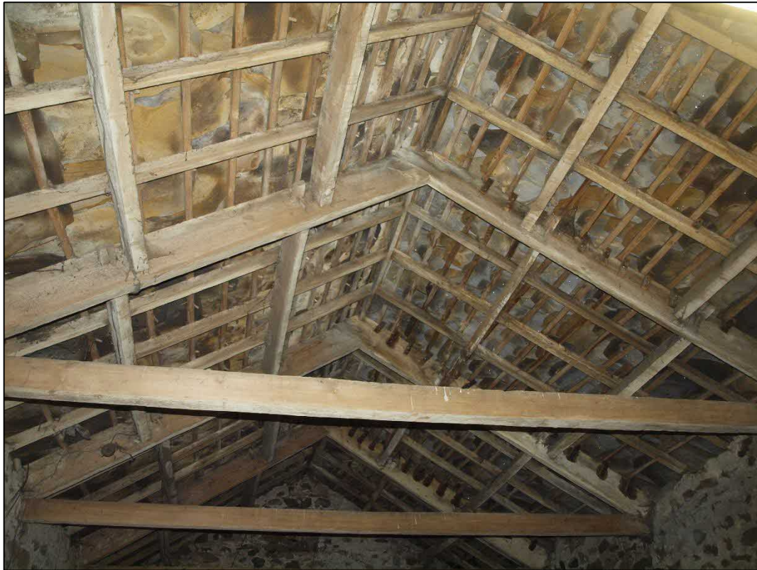
Plate 51: Truss detail looking west
