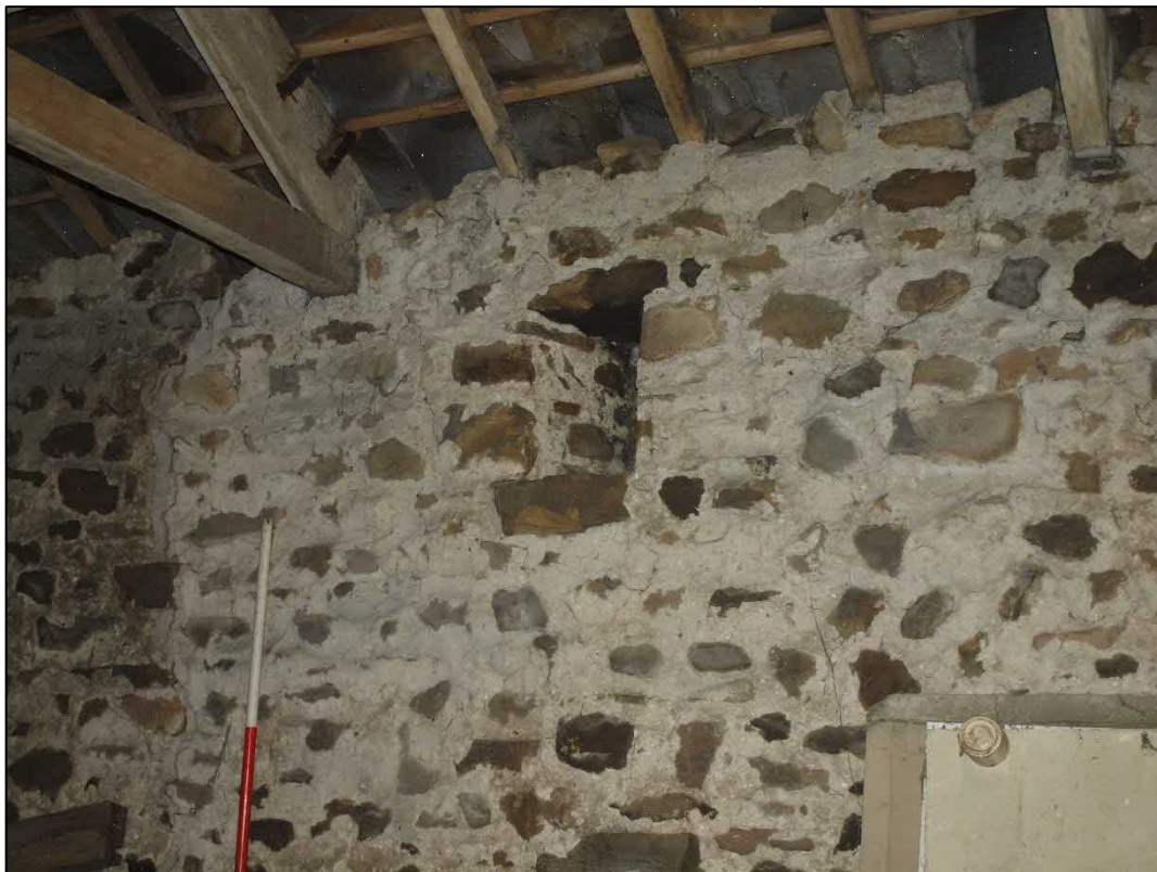
Plate 56: Ventilation slot in north wall looking northwest
