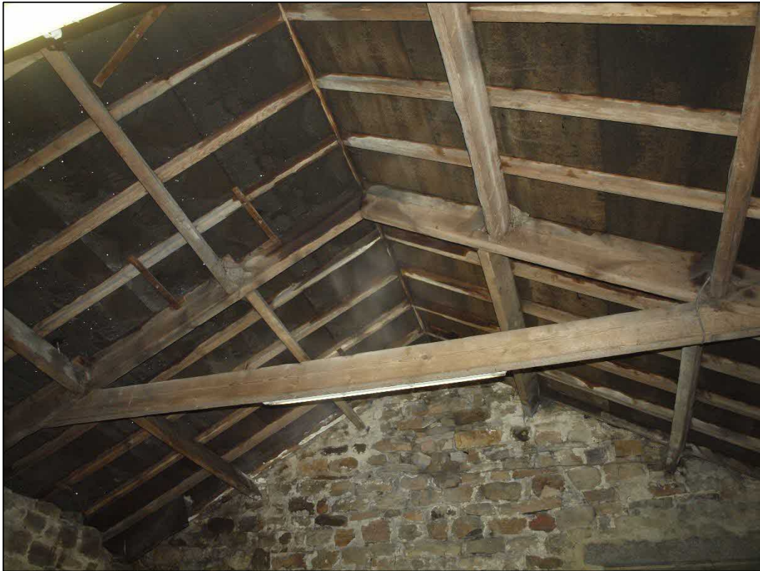
Plate 61: Detail of roof structure looking east
