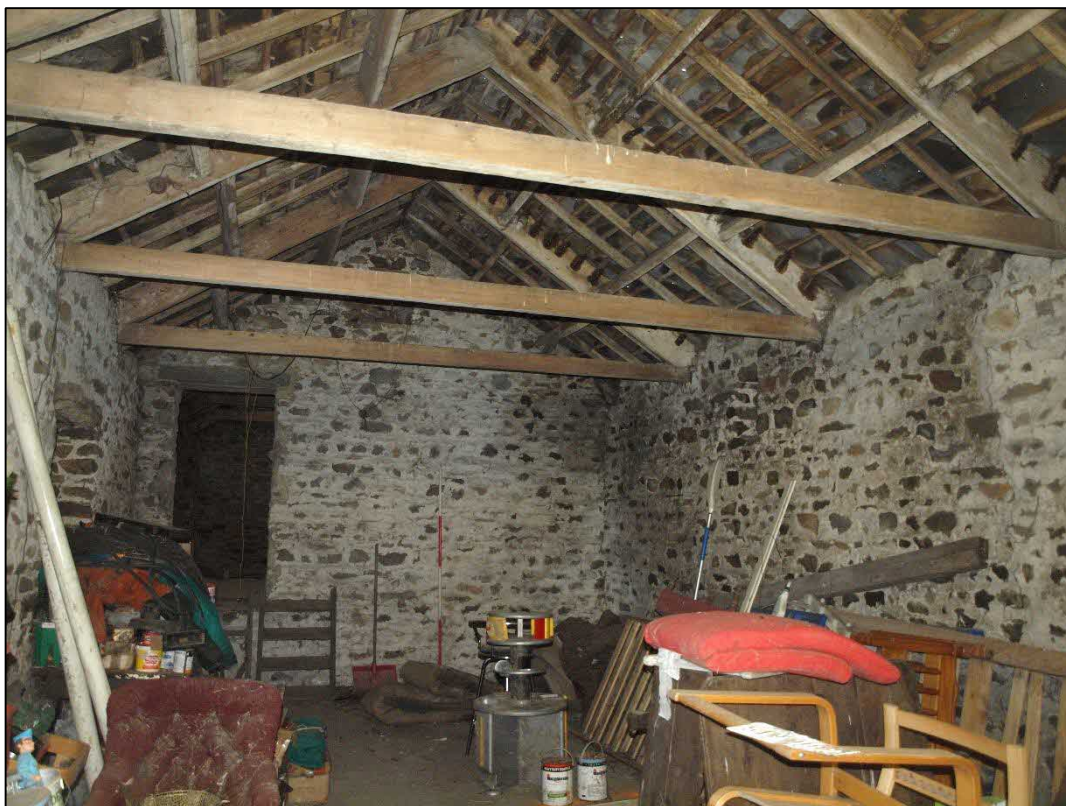
Plate 50: East end of first floor looking west
