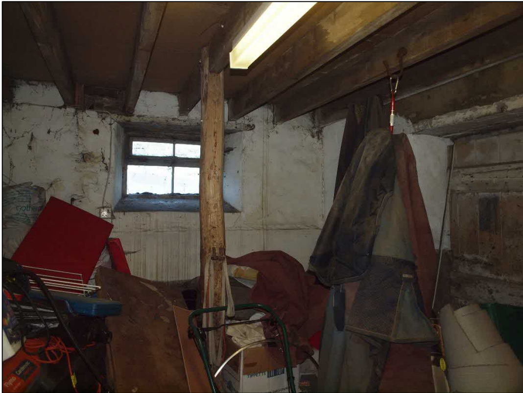
Plate 33: Room to bay 3 looking northeast
