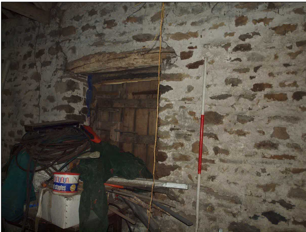
Plate 54: Pitching eye to south elevation looking south
