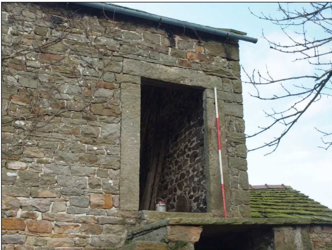
Plate 16: First floor doorway to bay 10 looking north
