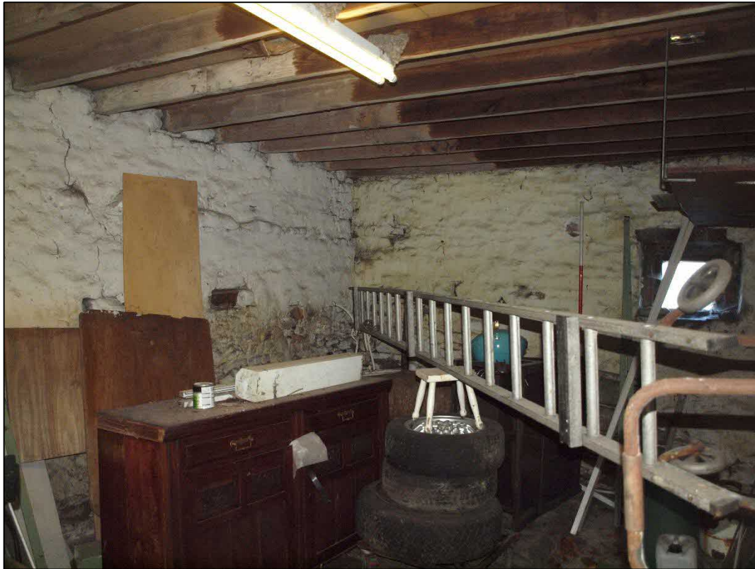
Plate 45: Room in bays 9 & 10 looking northwest
