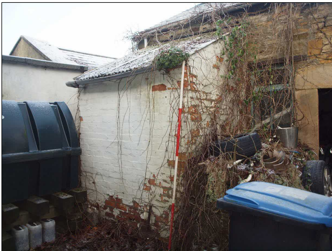
Plate 2: Brick lean-to to bay 1 looking northwest
