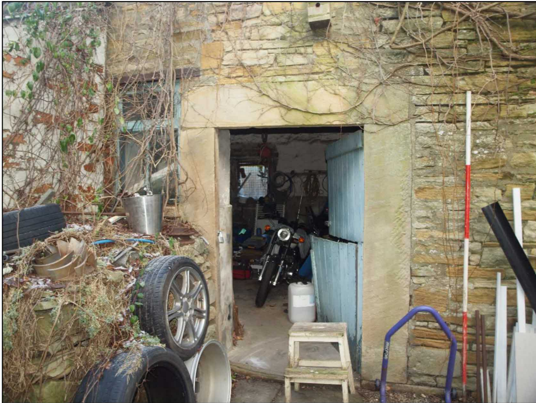
Plate 3: Doorway and window to bay 2 looking north
