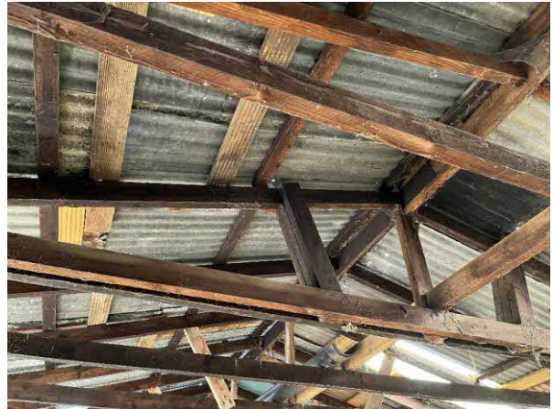
Photograph 4. Internal detail of the roof and wooden beams.
