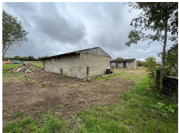
Photograph 6. The southern section of the stable building.
