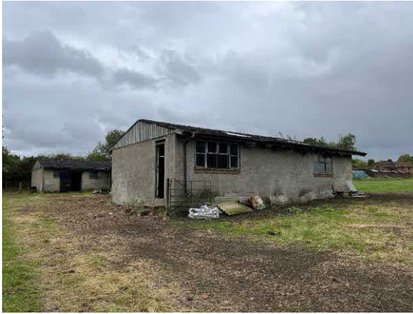
Photograph 1. The northern section of the stable building at Glebe Farm.
