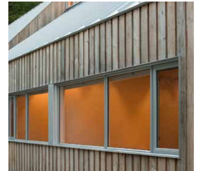
FIGURE 13. VERTICAL CLADDING AND ALUMINIUM WINDOW
