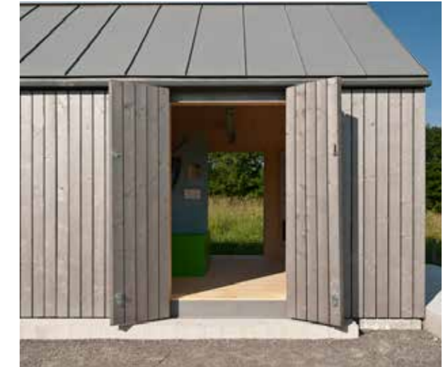
FIGURE 11. VERTICAL CLADDING AND METAL ROOF
