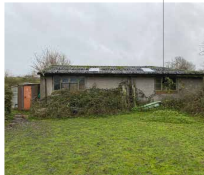
FIGURE 8. EXISTING NORTH ELEVATION
