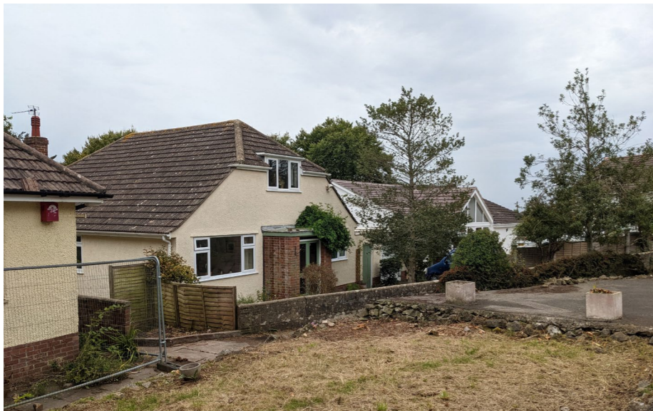
Neighbouring Treelands, located directly west of Woodrising. House has a mansard roof and concrete tiles, render and brick facade. Boundary with combination of low concrete walls and timber fence. Level tarmac driveway with rubble edge.
