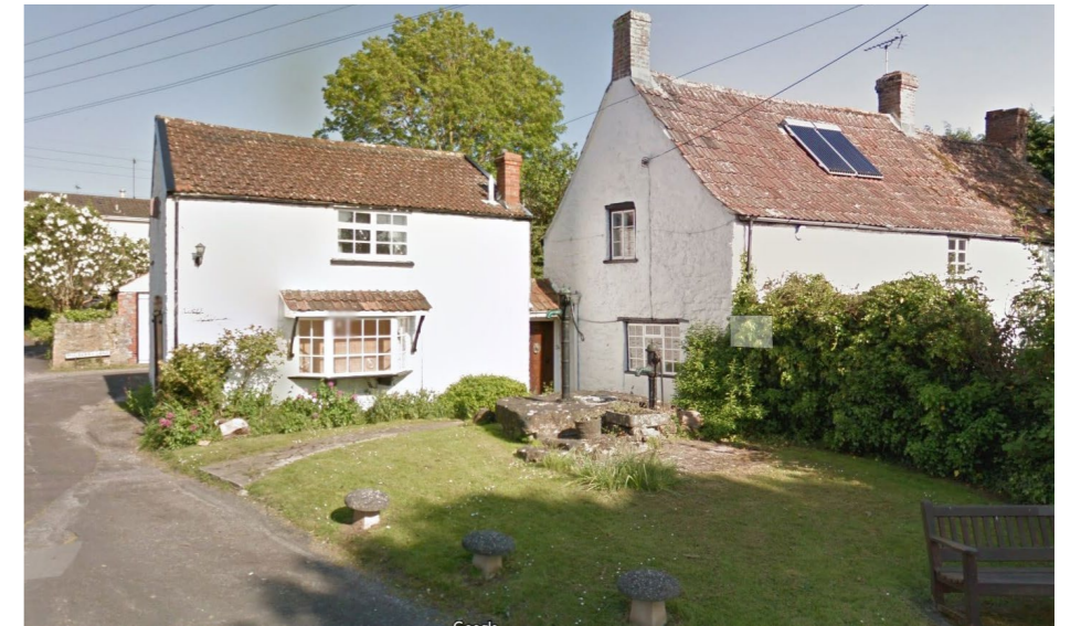
Grade II Listed building White rendered stone with corbelling detail to eaves. Windows with timber cills & lintels and white window frames.
