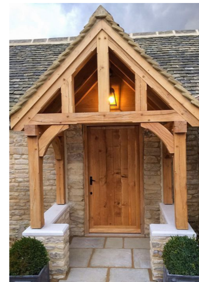
Timber porch & stone base
