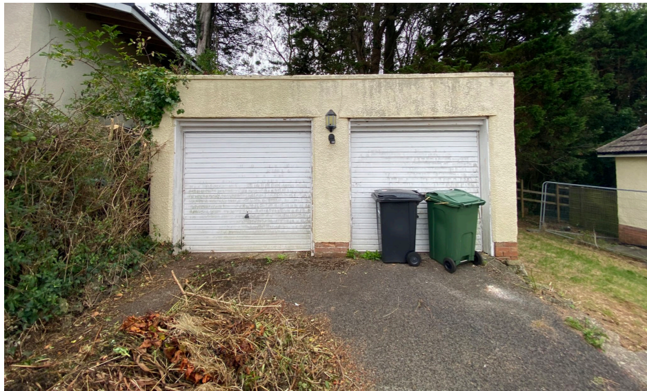
Front of double garage. Neighbours property is significantly higher on an upper level with wide overhanging eaves.
