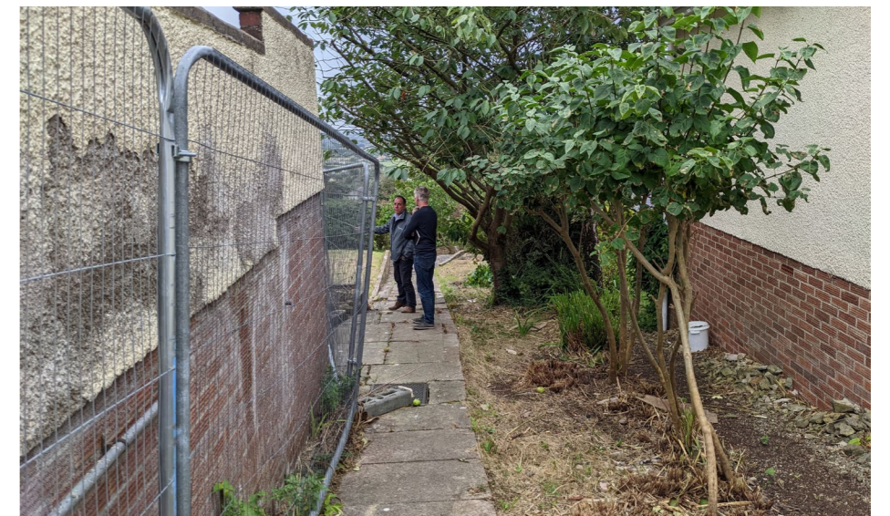
Area between Woodrising and Treelands, with concrete slabs and open plant edge
