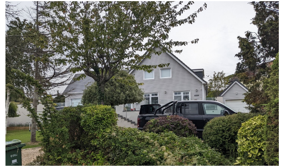
Upland Way along Hillside Road - recently re-clad with timber-effect weatherboarding, white UPVC windows and slate tiles
