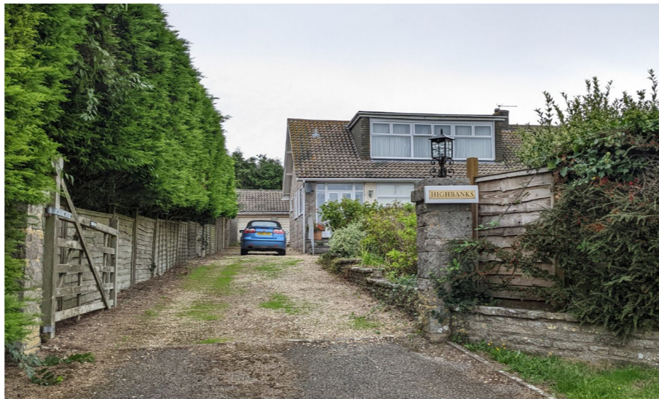
Mid-century bungalow with large dormer along Roman Road, UPVC windows and clay tile roof
