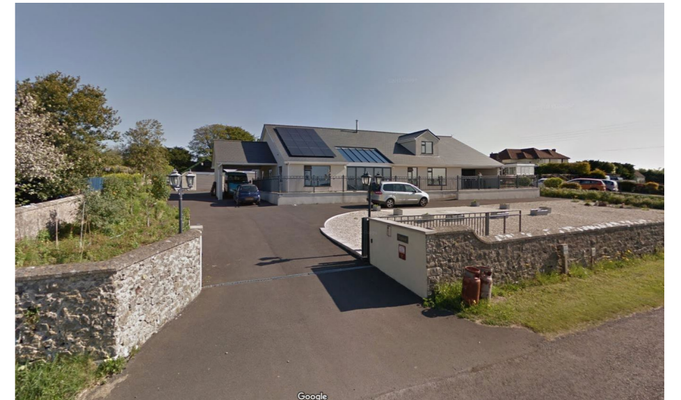
House along Roman Road 1.5 storey dwelling with areas of large glazed roof-lights, solar panels, car port dormer window and slate tiled roof
