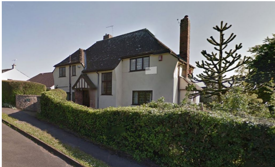
House along Hillside Road. Timber windows with wire glass, Tudoresque pitched porch, rendered facade with brick chimney & detailing and flat tiled mansard roof. Noticeably 2-3 storey house with corbel detailing.
