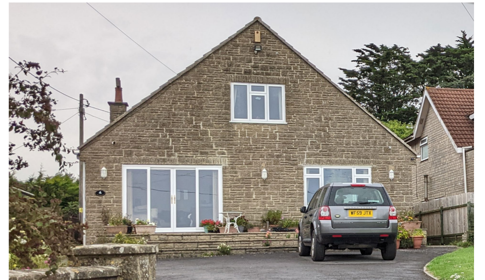
1.5 storey stone dwelling along Roman Road. Stone facade with corbels, thin verge detail, white UPVC windows and tarmac driveway and low height external stone walls.
