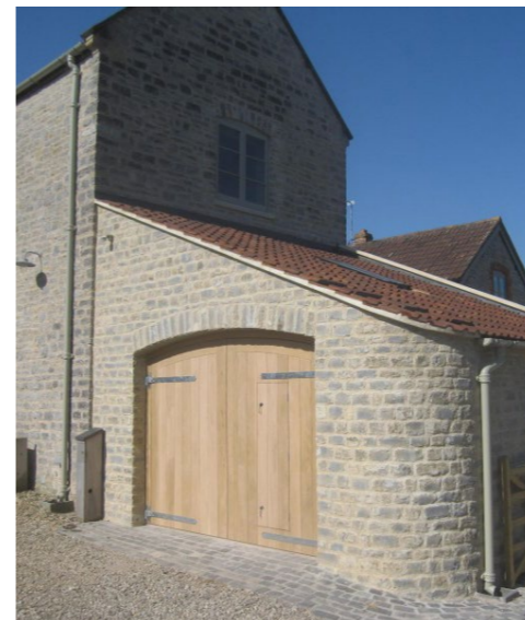
Rubble lias stone - similar to stone sourced locally
