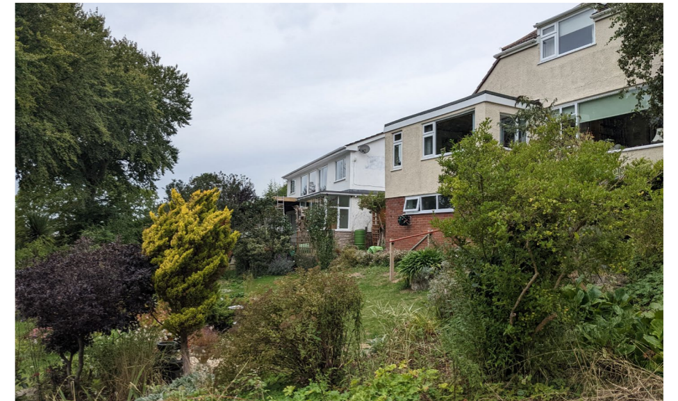
Rear elevations of neighbouring west properties show dwellings have internal arrangements spread across 3 floors.
