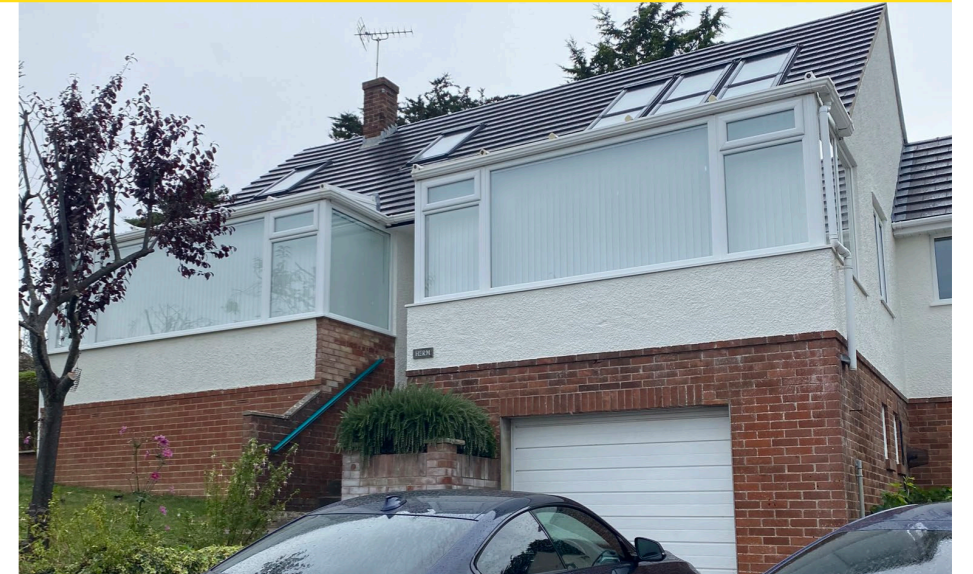
Herm along Hillside Road. Brick base and detailing with render above, white UPVC windows, flat tiles and roof-lights.
