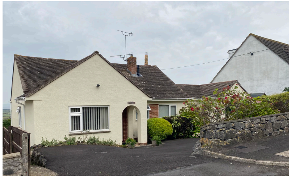
Ayton along Hillside Road. Cream render building with elements of brick, recessed arched porch, single storey in appearance, corbel detail, thin verge detail with concrete flat tiles.
