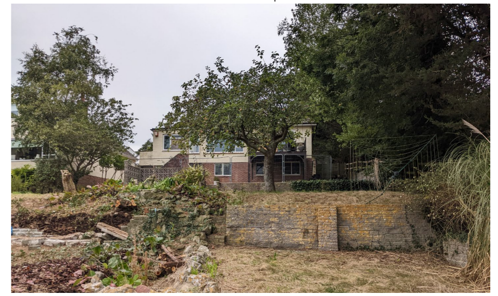
Rear elevation of Woodrising from lower garden level. Shows the trees closest to property within the landscape.
