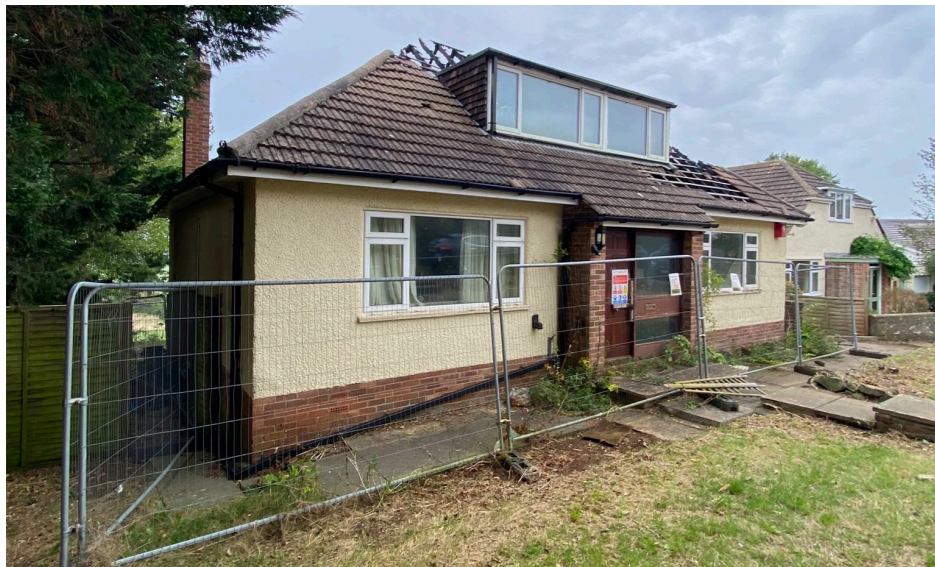
View of front elevation. Existing with brick base and porch detailing with upper cream coloured render
