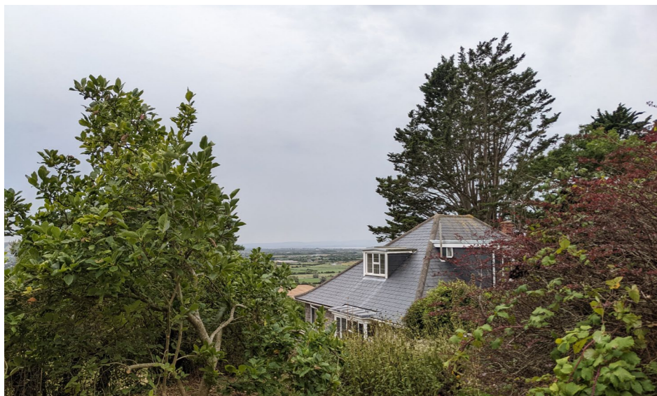
View south west from applicants garden. Roof of Bramble Bank in shot have mansard windows with single ply lead roof over. Roof predominately slate roof tiles with concrete ridges.
