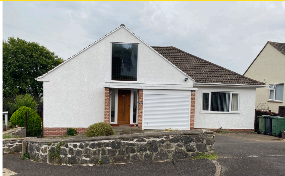
Sirius along Hillside Road: recessed entrance with flat roof porch, pitched elevation, thin profile roof verge, brick footing and render facade, corbel detail & large unobstructed windows facing street.
