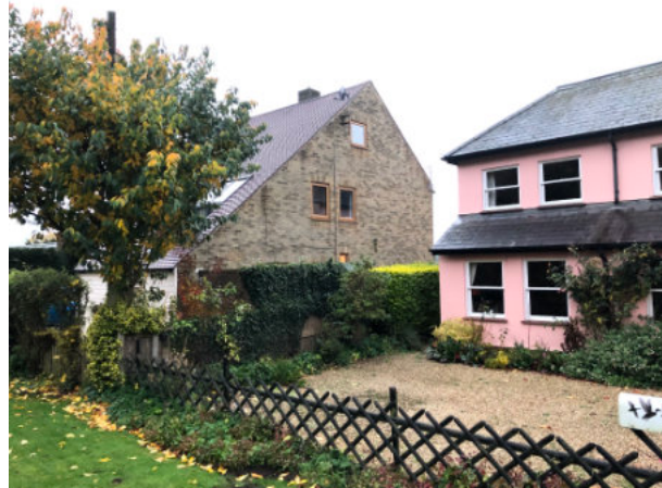
View from existing house frontage towards southern neighbouring boundary
