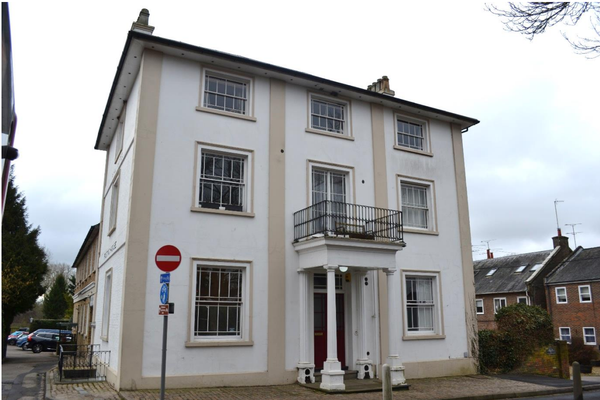
Figure 11: North (front) elevation of the Posting House.
