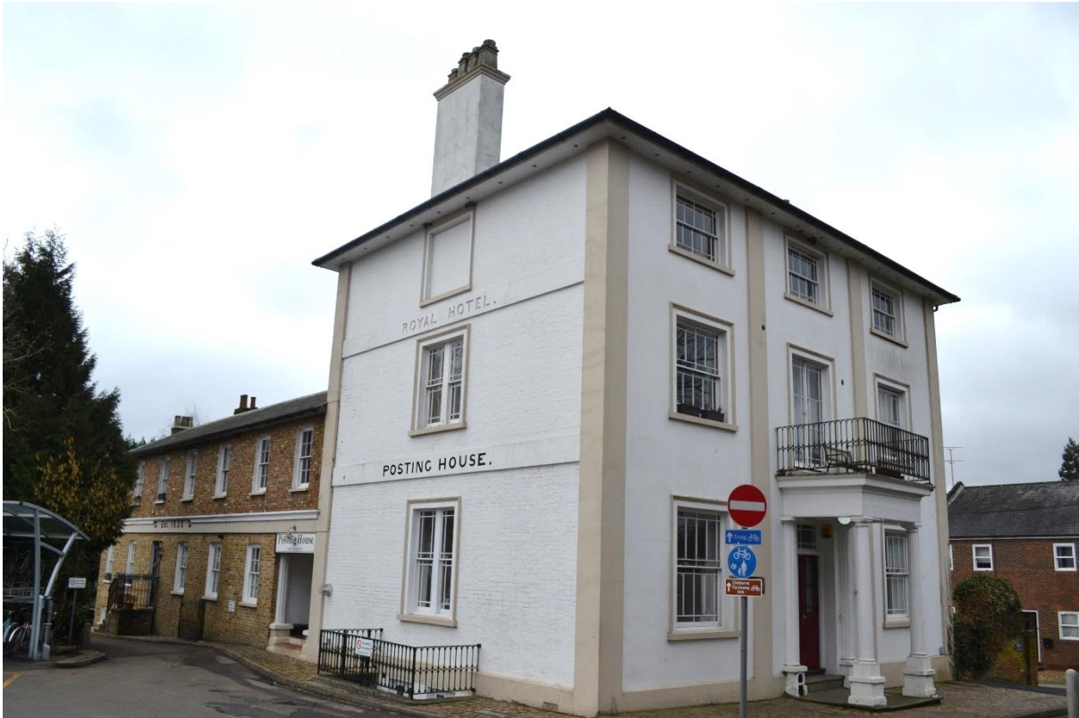
Figure 10: North-east elevation of the Posting House.
