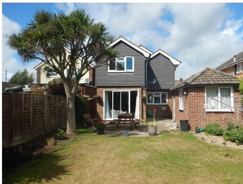
Existing rear of 21 Beverley Road
