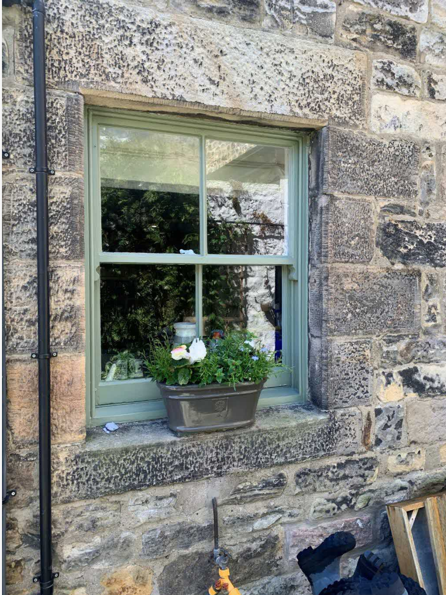
Photograph 2 showing one of the existing kitchen windows (east elevation ground floor).
