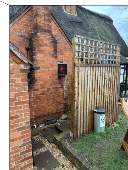
'A' - FENCE SCREENING EXTRACTOR FANS 1.8m x 1.8m x 2.4m high, close boarded fence with trellis above
