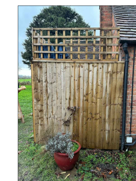
'A' - FENCE SCREENING EXTRACTOR FANS 1.8m x 1.8m x 2.4m high, close boarded fence with trellis above
